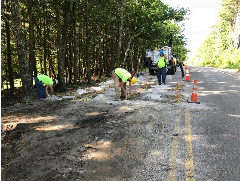
Photo 3 – Loading for first blast of the day near Tall Pines Way
