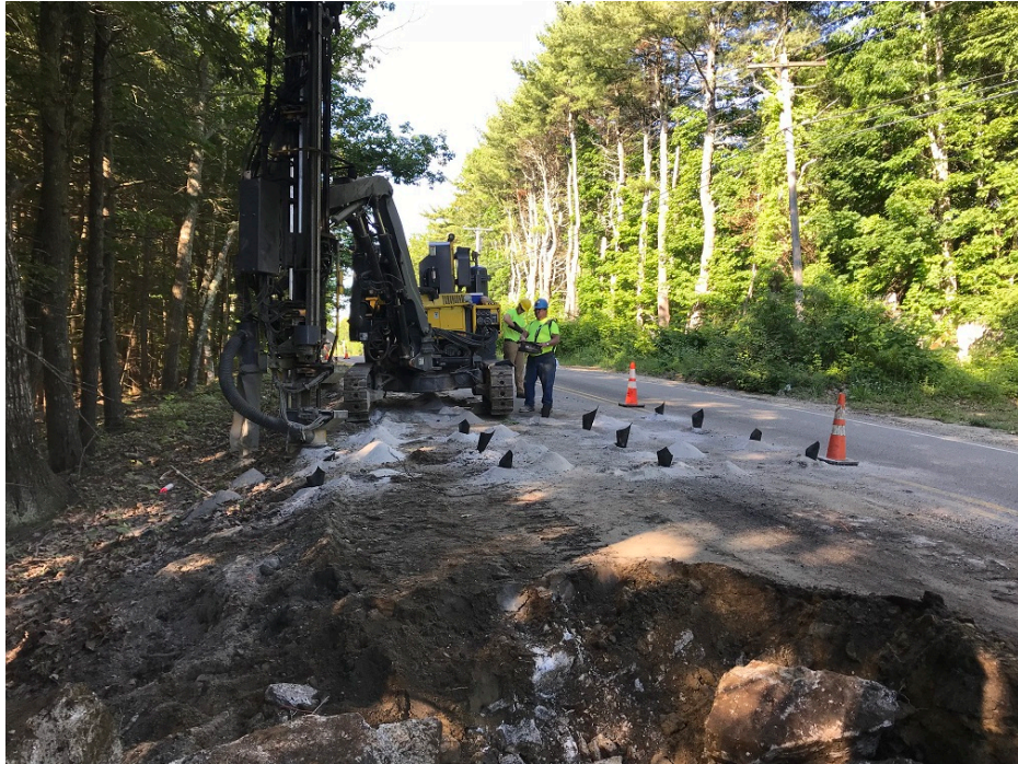
Photo 1 – Drilling for first blast of the day near Tall Pines Way
