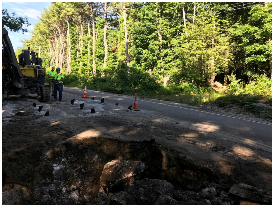
Photo 2 – Preparing for first blast of the day near Tall Pines Way
