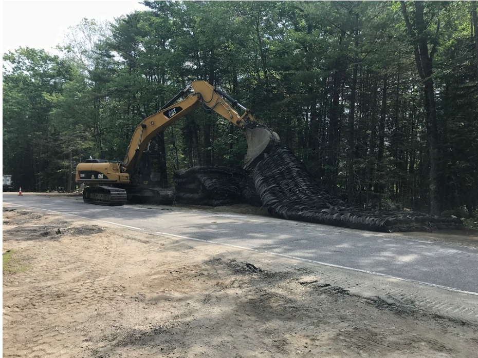
Photo 1 – Removing blasting mats after a blast near 15 Middle Road
