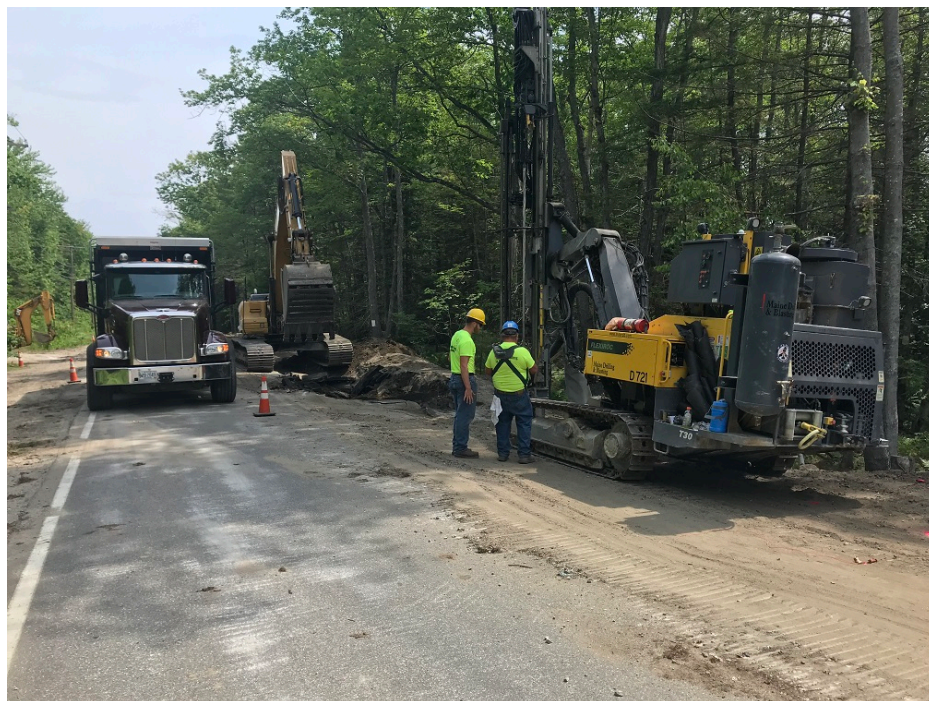
Photo 4 – Drilling for blasting and clean up after a blast
