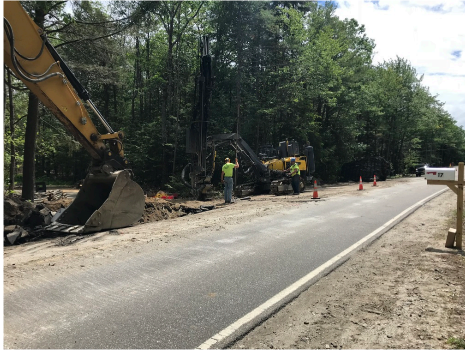
Photo 7 – Drilling for blasting holes
