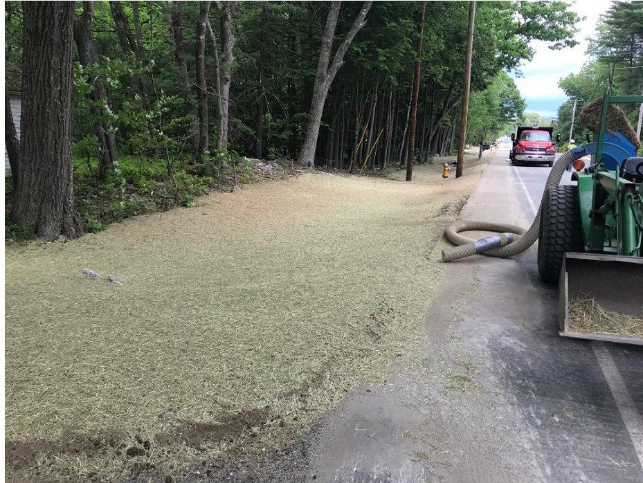
Photo 3 – Loam, seed, and mulch in front of 34 Middle Road
