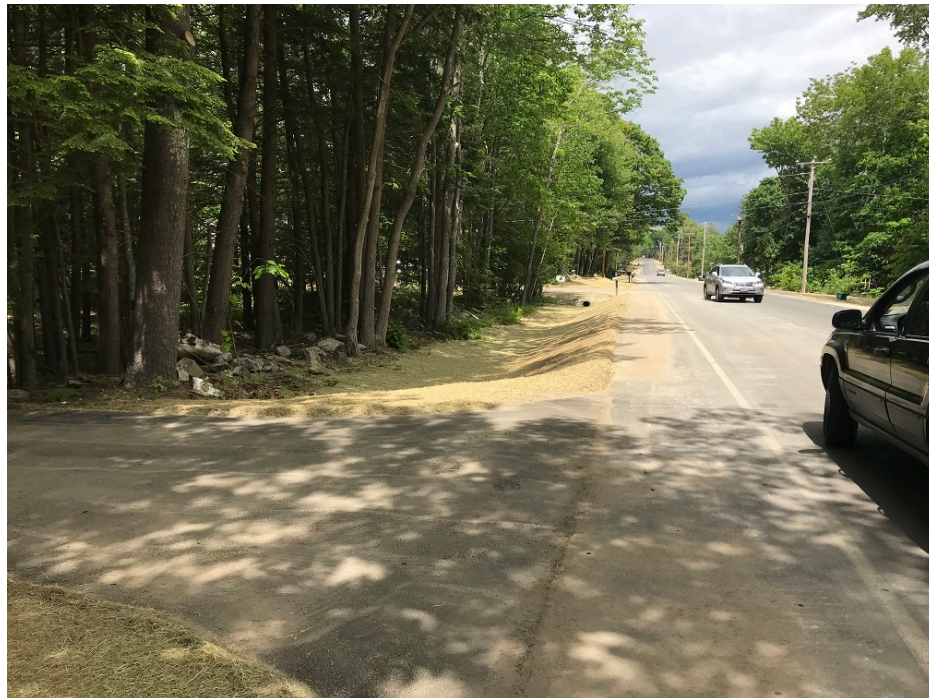
Photo 4 – Loam, seed, and mulch in front of 34 Middle Road
