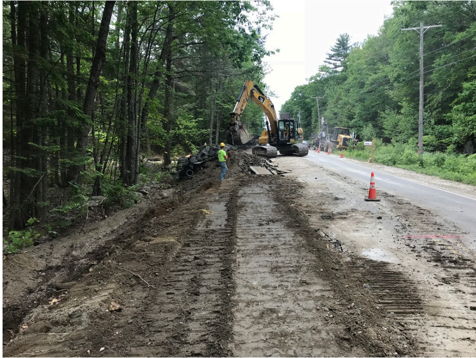
Photo 1 – Removing blasting mats after a blast
