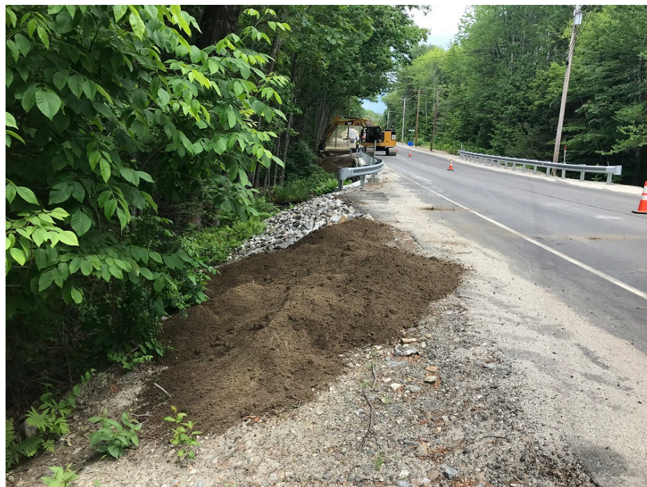
Photo 2 – Placing loam near Evergreen Lane
