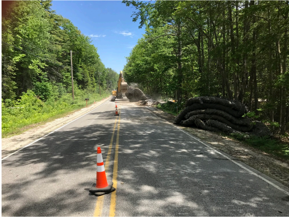
Photo 1 – Removing blasting mats after a blast
