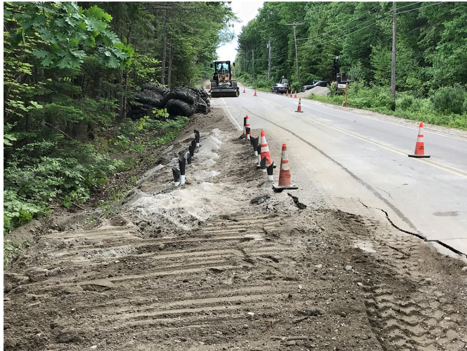
Photo 8 – Drill holes for blasting the next day
