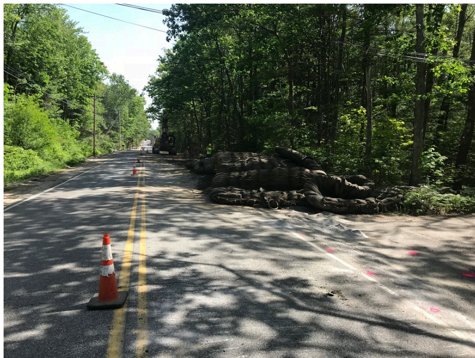
Photo 4 – Placing blasting mats
