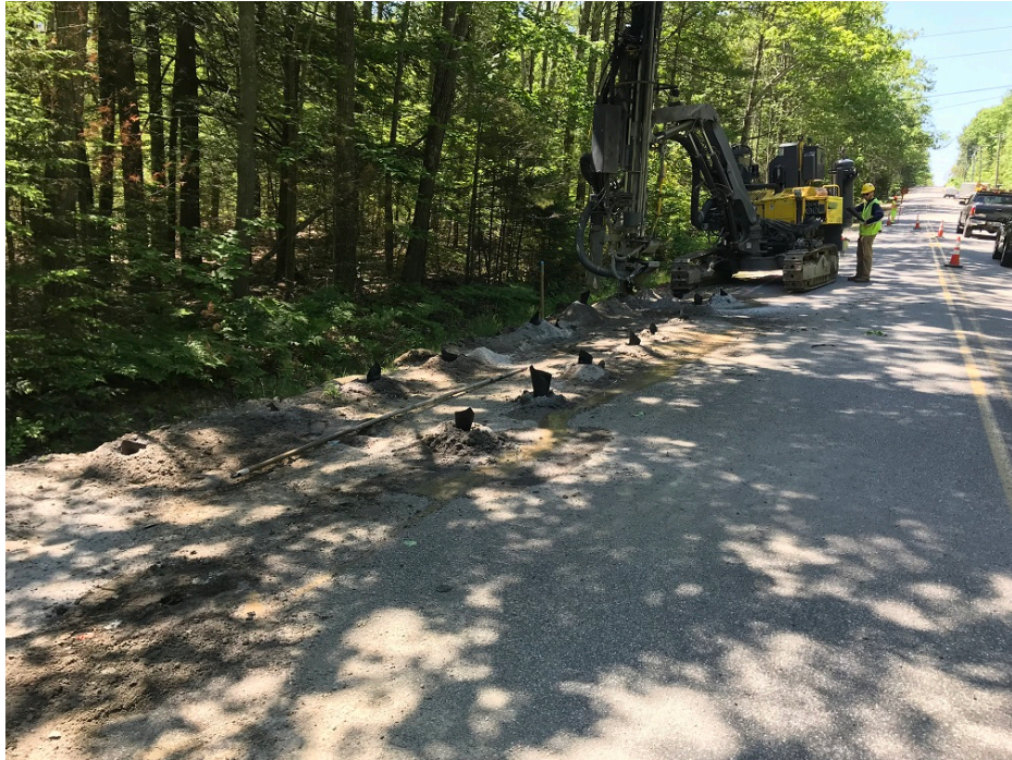
Photo 1 – Drilling for bedrock removal just north of Evergreen Lane
