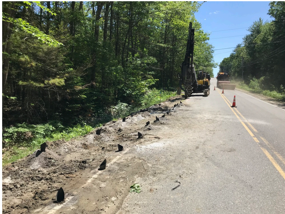
Photo 8 – Preparing to load probes for blasting bedrock just north of Evergreen Lane
