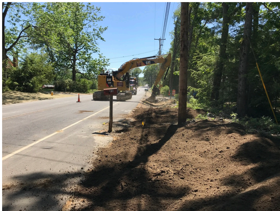
Photo 6 – Shaping the ditch in front of 88 Middle Road
