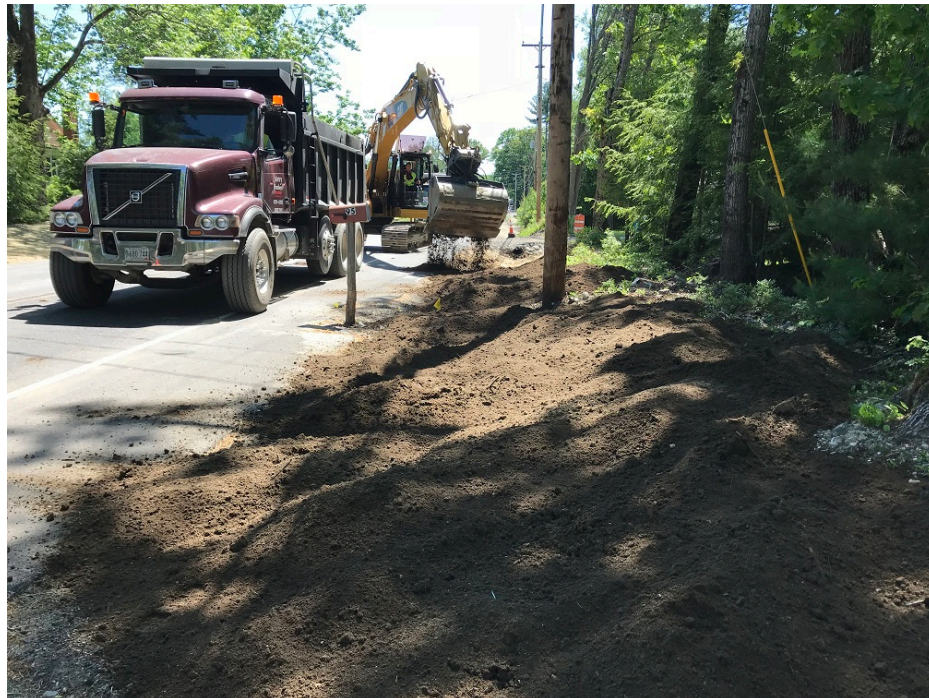
Photo 4 – Placing loam in front of 88 Middle Road
