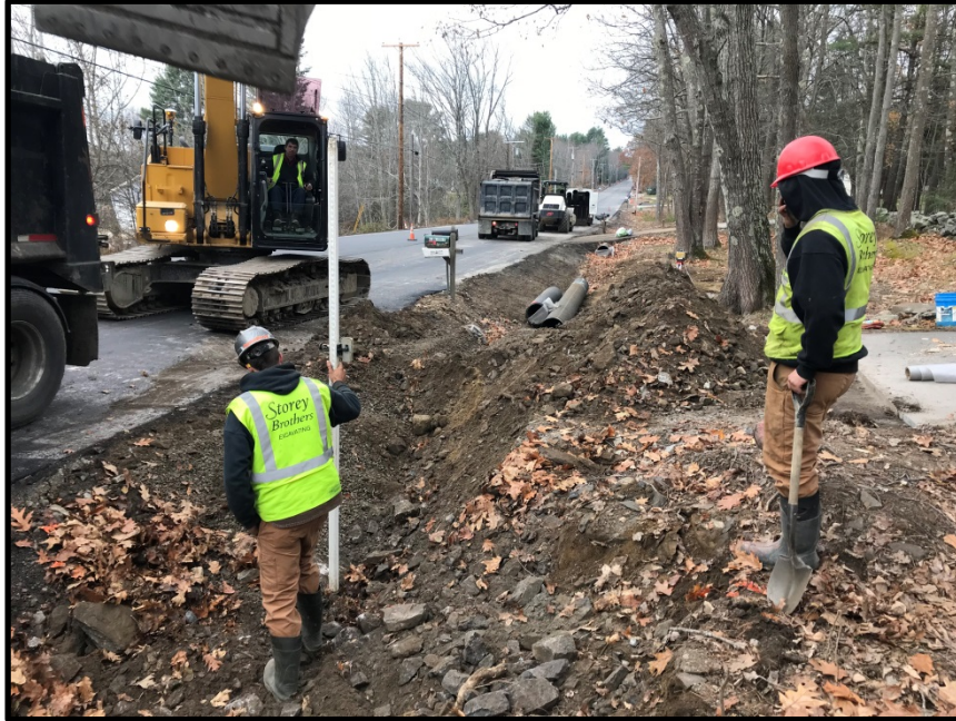
Photograph 1 – Thursday, November 16 th – Installing culvert at 62 Middle Road.
