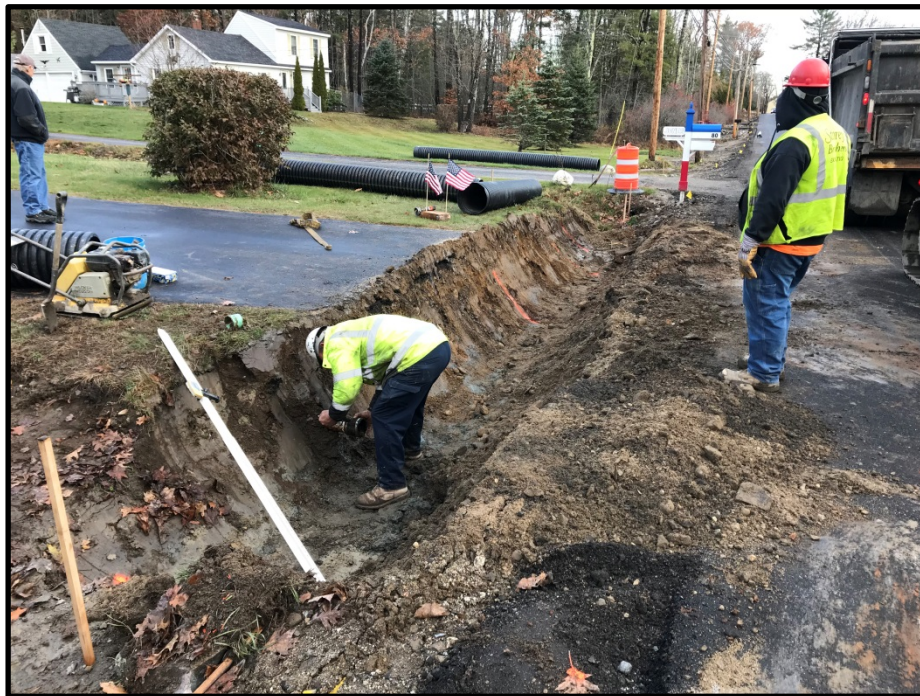
Photograph 4 - Friday, November 17 th – Installing culvert at 78 Middle Road.
