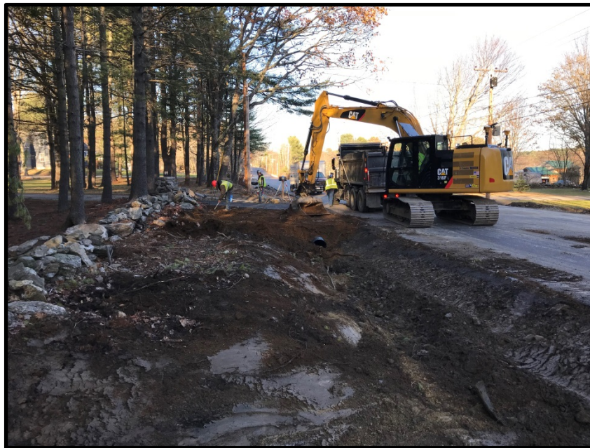
Photograph 8 - Tuesday, November 21 st – Extended culvert and ditching in front of 44 Middle Road.
