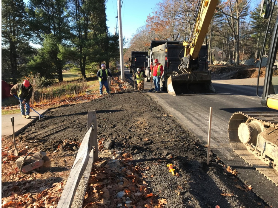
Photo 1 – Grading driveway and preparing for pavement at 71 Middle Road.
