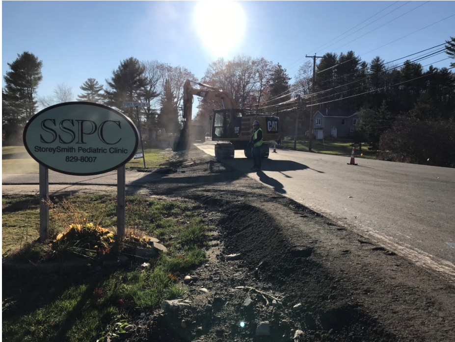
Photo 5 – Backing up edge of pavement at Storey Brook Lane.
