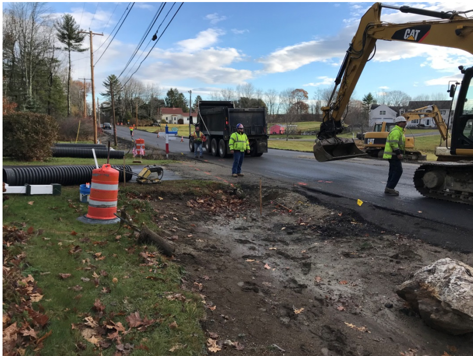
Photo 2 – Preparing to install driveway culvert at 78 Middle Road.
