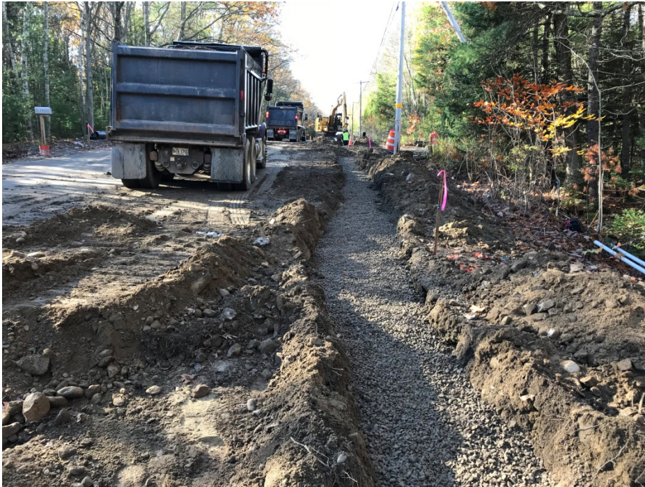
Photo 1 – Installing 6 inch UD STA 16+40 to STA 13+00 on west side of Middle Road.
