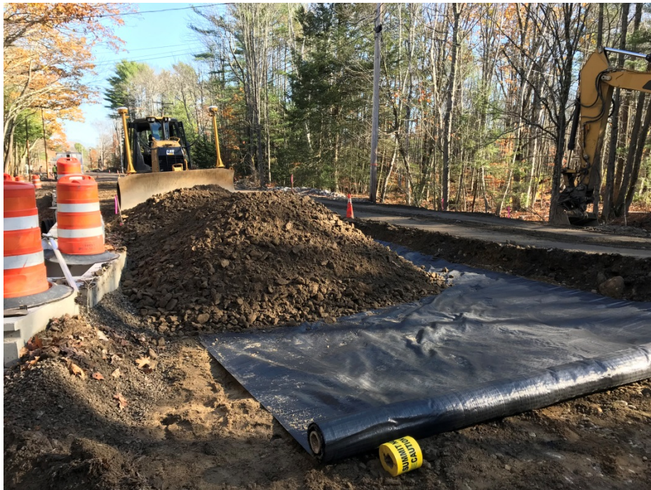
Photo 2 – Placing subbase gravel at STA 17+00.
