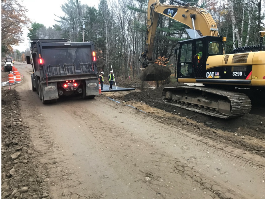
Photo 5 – Box cut for full depth construction on east side of Middle Road.
