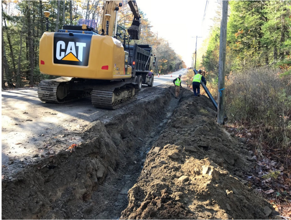
Photo 3 – Installing 6 inch UD at STA 13+00 on west side of Middle Road.
