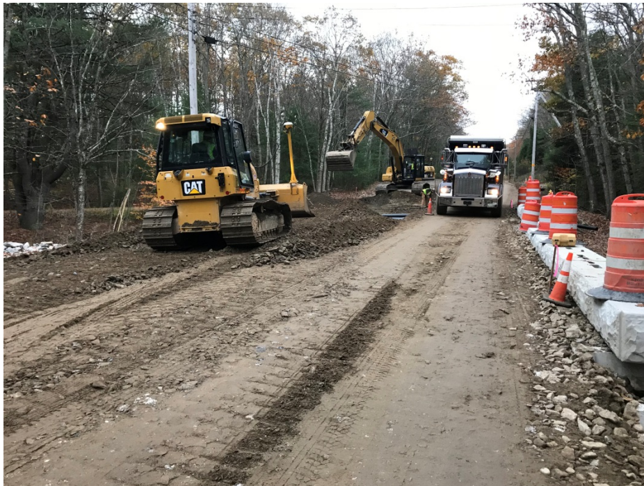
Photo 4 – Box cut for full depth construction STA 16+00 on east side of Middle Road.
