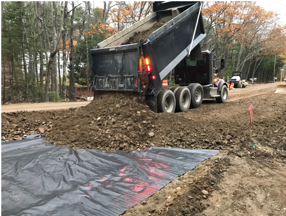
Photo 6 – Placing subbase gravel at STA 16+00 on east side of Middle Road.
