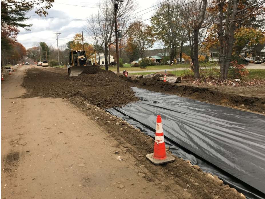
Photo 5 – Placing subbase gravel east side of Middle Road, STA 22+50.
