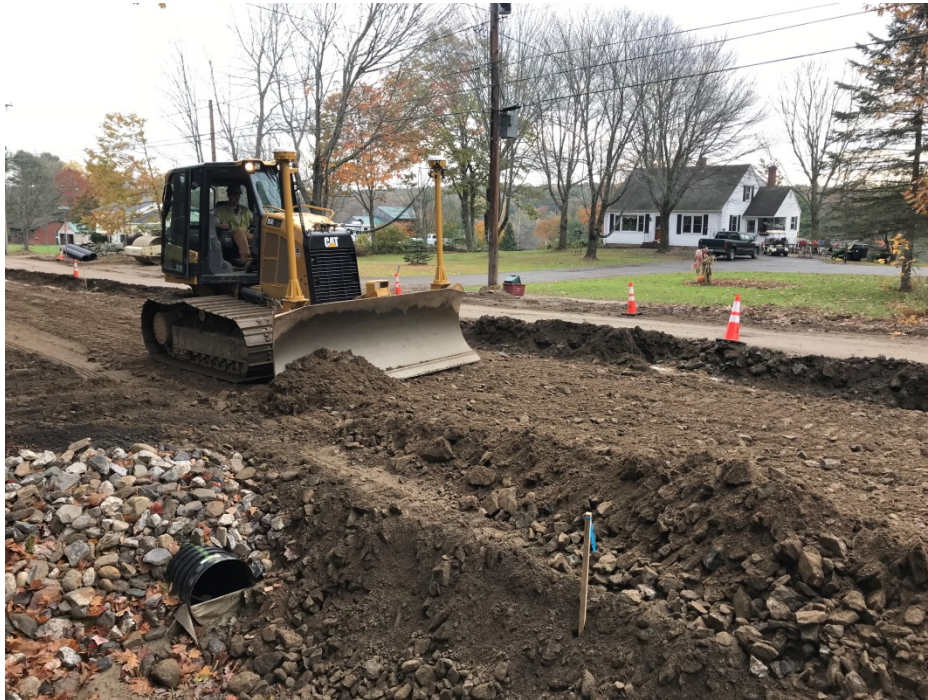
Photo 2 – Placing subbase gravel.
