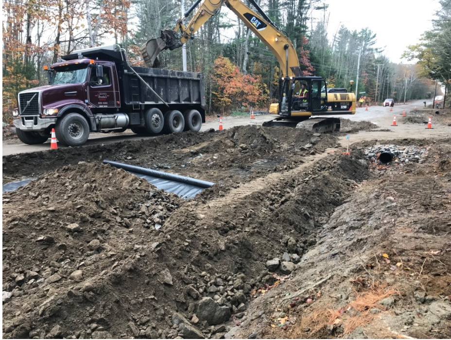
Photo 1 – Box cut for full depth construction on west side of Middle Road. Approximate STA 21+50.
