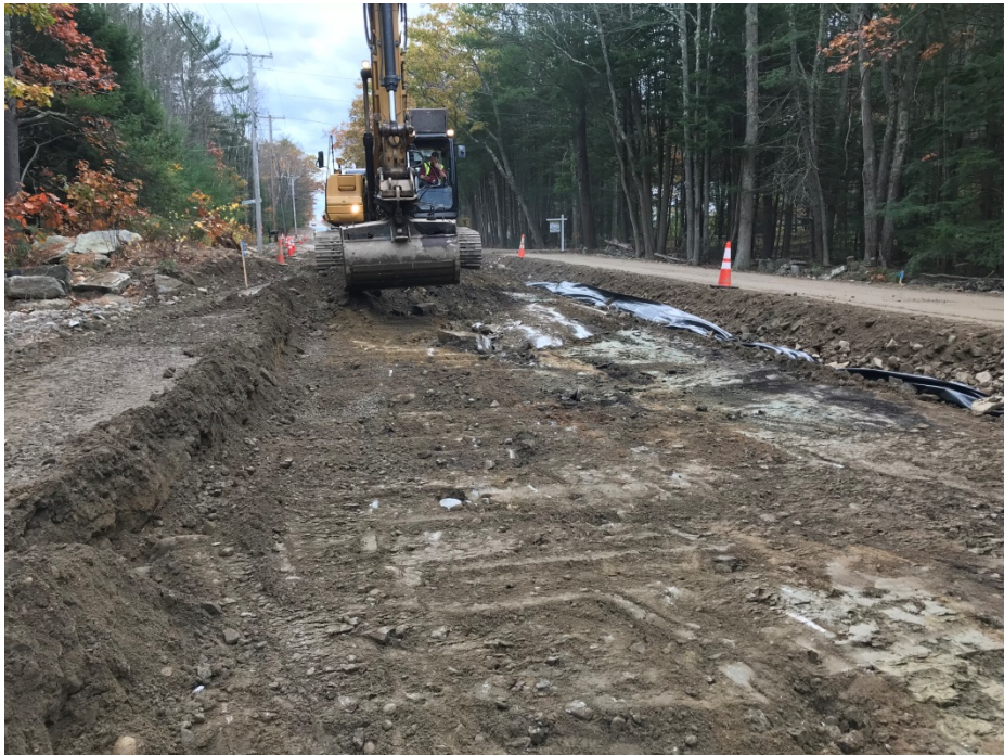
Photo 6 – Box cut for full depth construction east side of Middle Road, STA 20+50.
