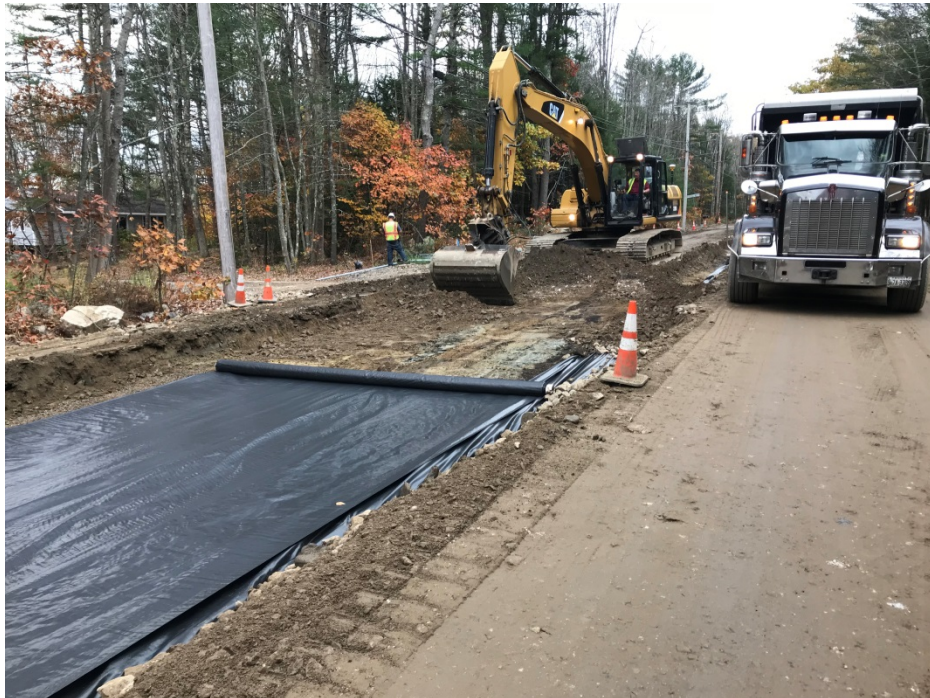
Photo 4 – Box cut for full depth construction STA 21+50 east side of Middle Road.
