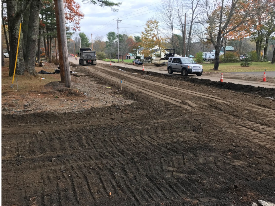
Photo 3 – Placing subbase gravel. Approximate STA 22+00
