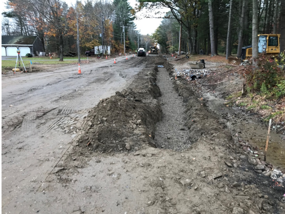
Photo 1 – Working on 6 inch UD at STA 24+00 southward on west side of Middle Road.
