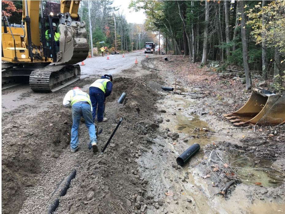
Photo 3 – Capped end of 6 inch UD on west side of Middle Road, STA 21+00.
