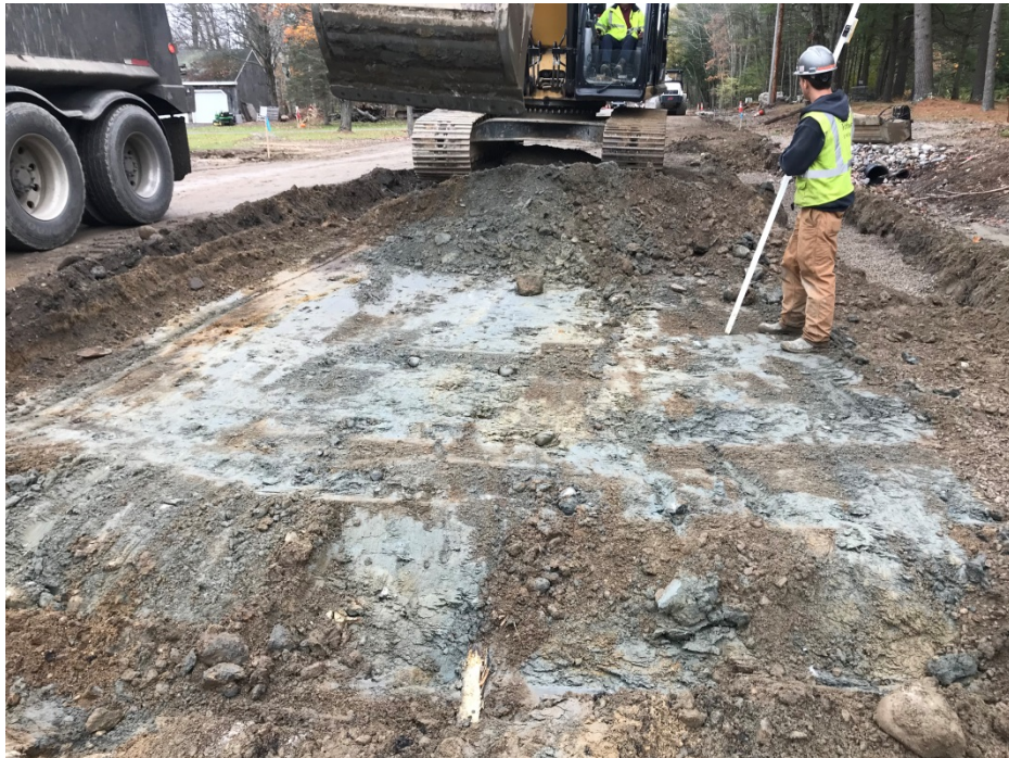
Photo 4 – Box cut for full depth construction STA 24+00
