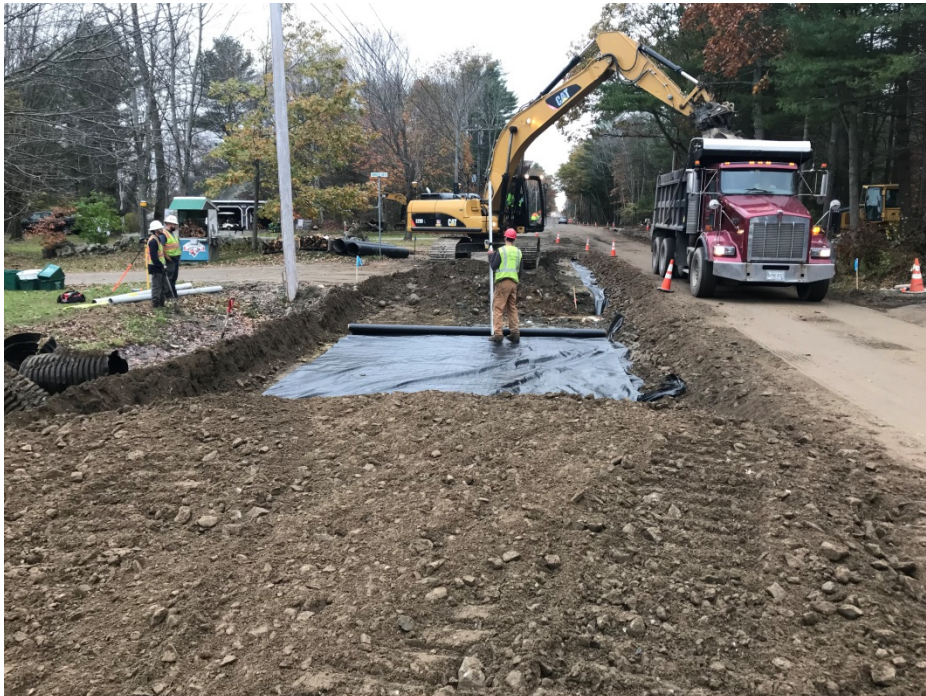
Photo 6 – Box cut for full depth construction east side of Middle Road, STA 24+00.
