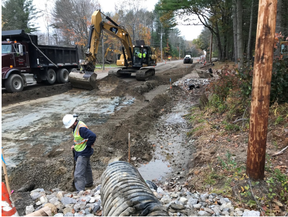
Photo 5 – Box cut for full depth construction on west side of Middle Road.
