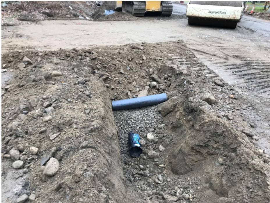
Photo 2 – Installing 6 inch UD on west side of Middle Road, STA 21+50.
