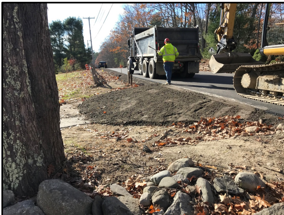
Photograph 10 – Wednesday, November 15 th – Backing up pavement and driveway entrances.
