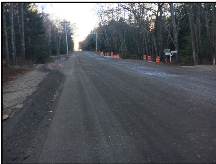
Photograph 4 - Friday, November 10 th – Middle Road fine graded looking southward from Waterfall Way.
