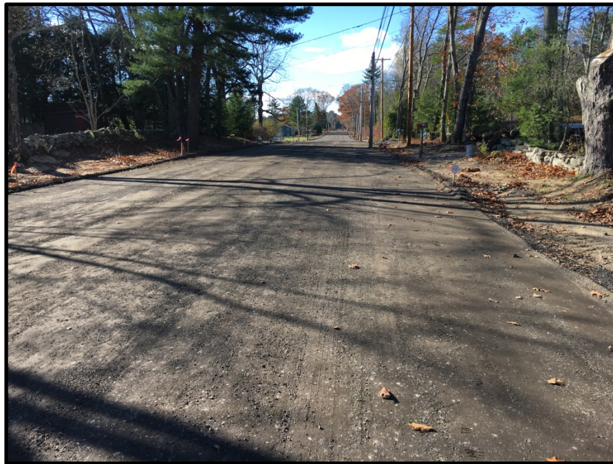
Photograph 3 - Friday, November 10 th – Middle Road fine graded looking southward from STA 49+50.
