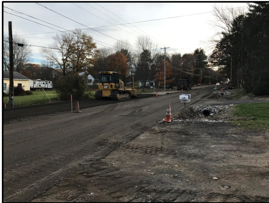
Photograph 2: Thursday, November 9 th – Placing and grading reclaim on east side of Middle Road near Shirley Lane.
