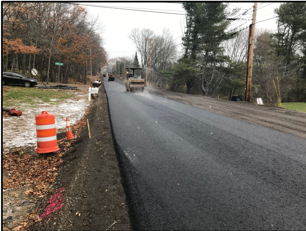
Photograph 6 - Monday, November 13 th – Compacting pavement on west side of Middle Road near Range Way.
