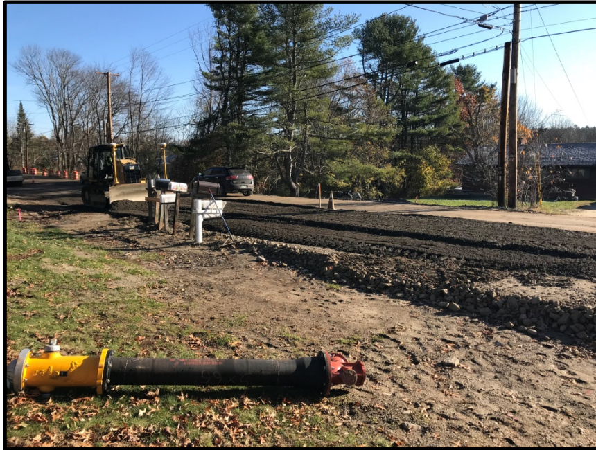
Photograph 1 – Thursday, November 9 th – Placing and grading reclaim on west side of Middle Road in area of Range Way.
