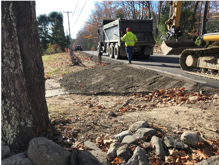
Photo 4 – Backing up driveways and edge of pavement.
