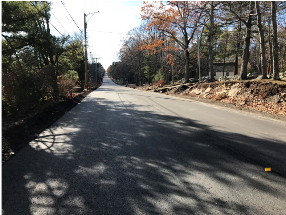
Photo 2 – Binder course pavement on Middle Road.
