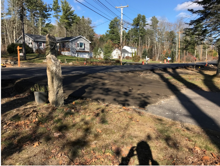
Photo 5 – Backing up driveways and edge of pavement.
