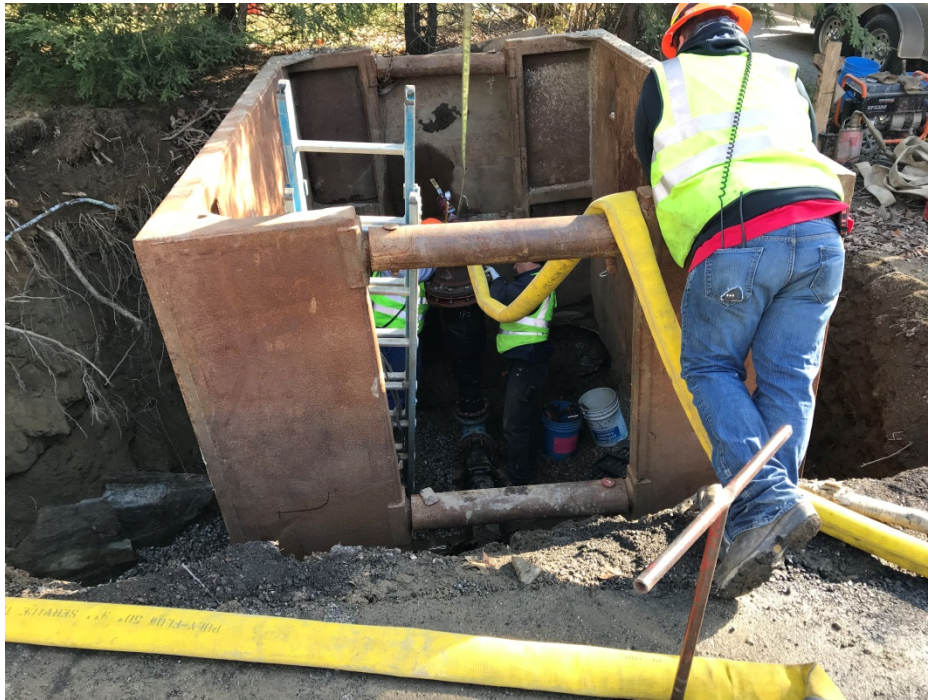
Photo 1 – Ted Berry setting up to pig the water main.
