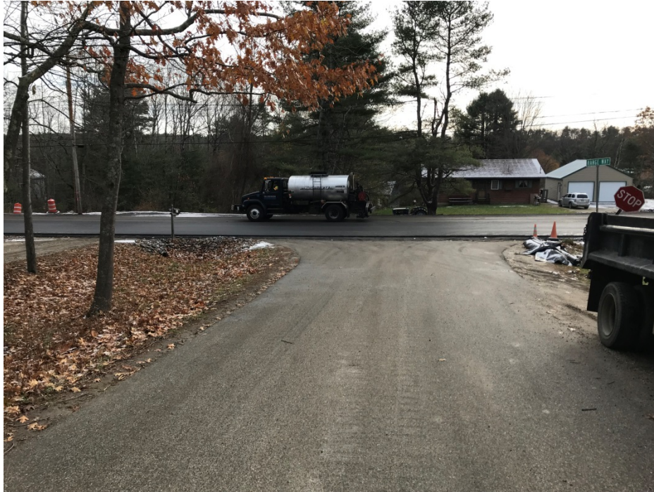
Photo 1 – Placing tack coat on centerline pavement joint.
