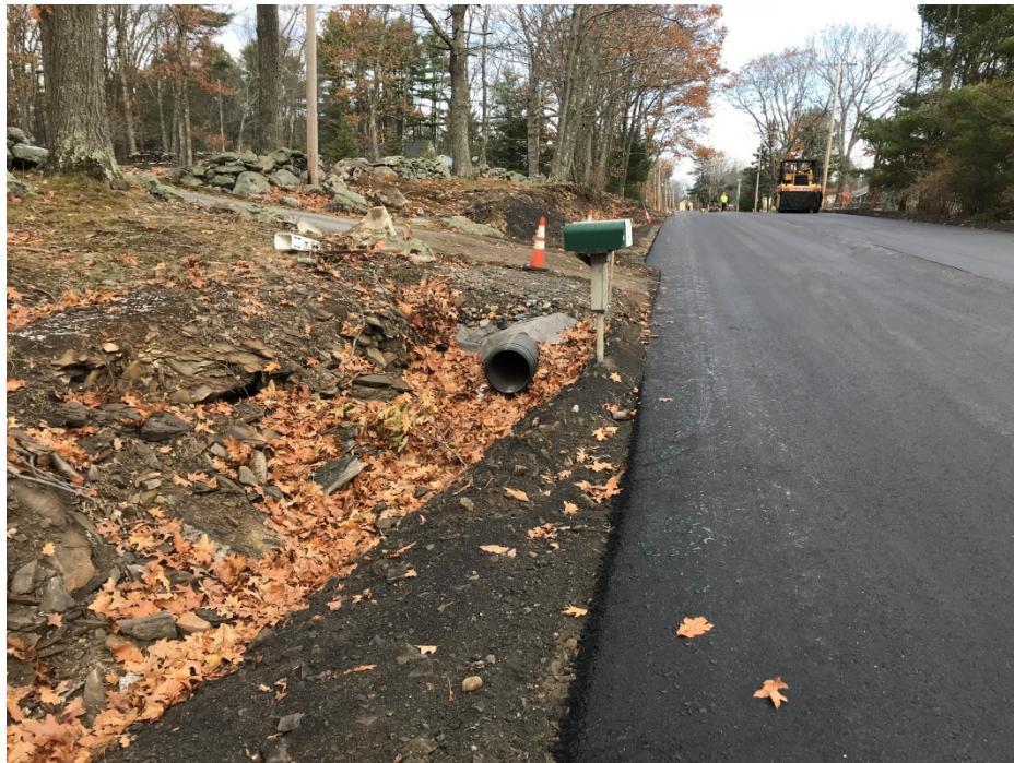
Photo 6 – Culvert at 70 Middle Road that will be reset lower to help with gradient at entrance of driveway.
