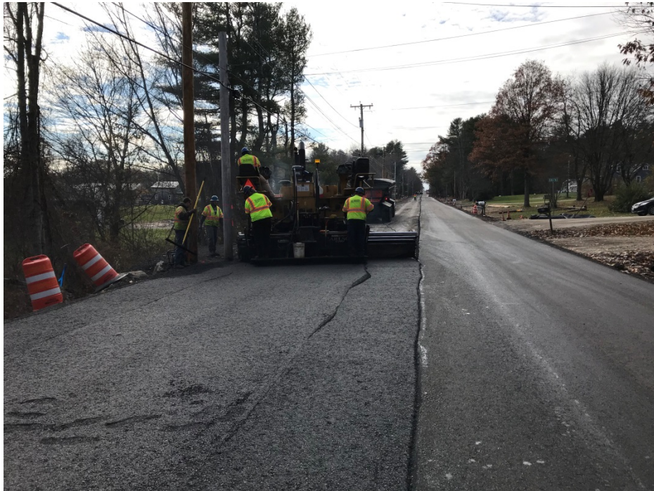
Photo 4 – Paving east side of Middle Road in front of Range Way.
