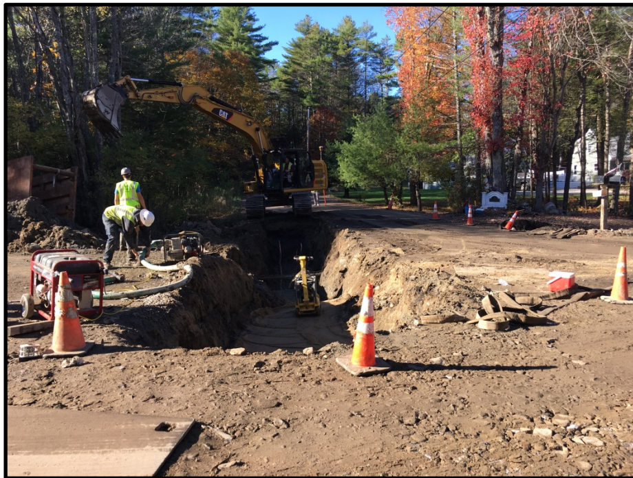
Photograph 4 - Friday, October 27 th – Backfilling water service at 42 Middle Road.
