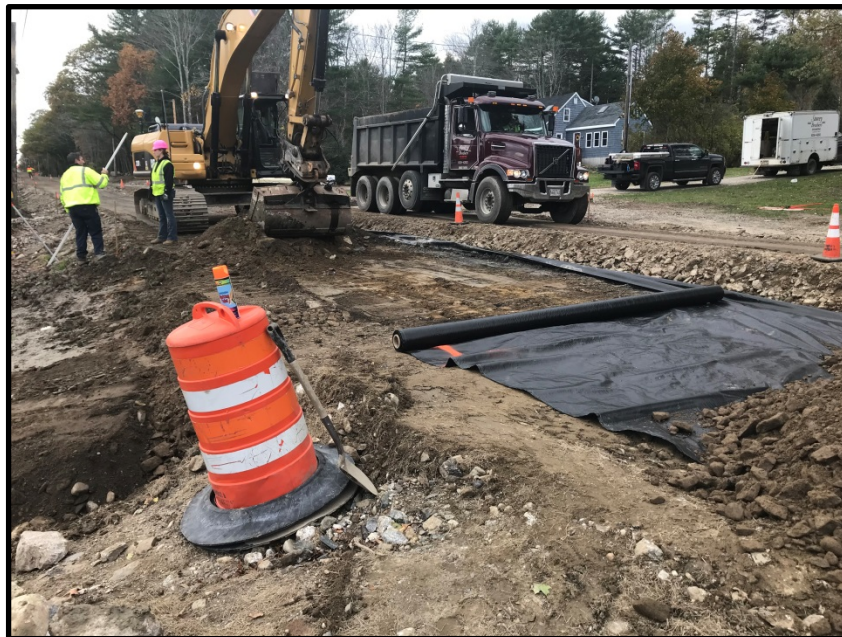
Photograph 8 - Tuesday, October 31 st – Box cut for full depth construction at STA 26+00 on west side of Middle Road.
