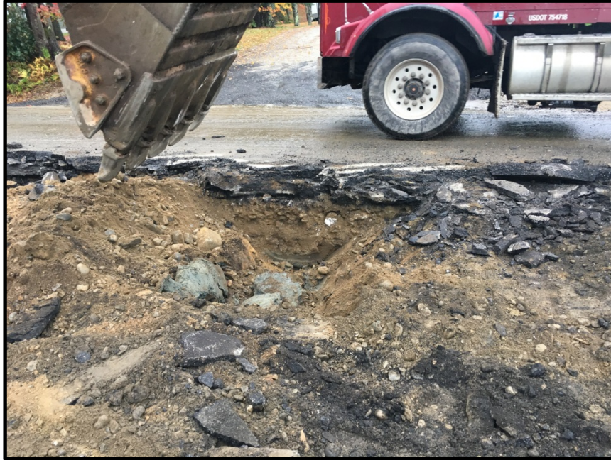
Photograph 1 – Thursday, October 26 th – Performed test pit while stripping existing pavement to determine existing pavement and gravel depths.
