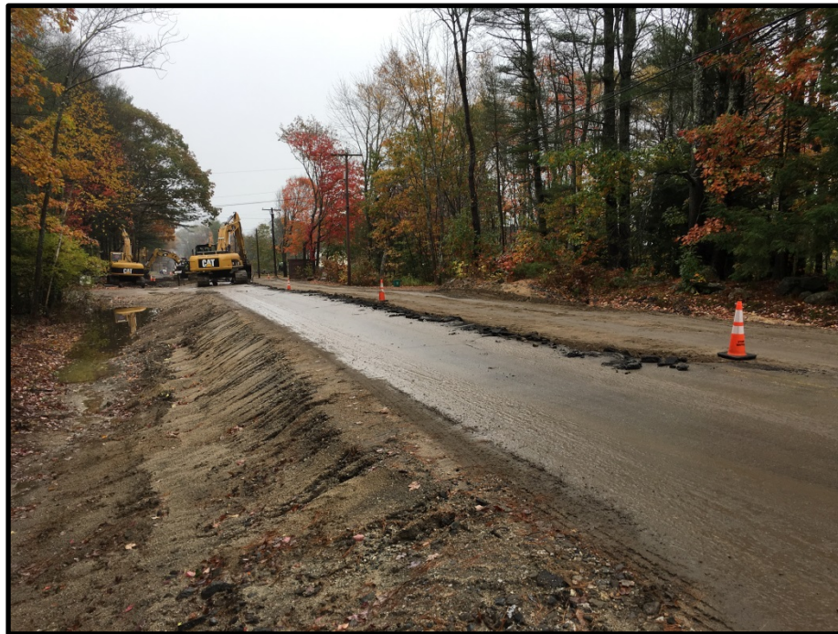
Photograph 2: Thursday, October 26 th – Stripping existing pavement in are in front of 42 Middle Road.
