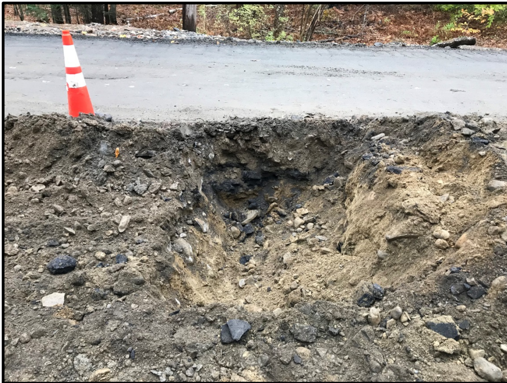
Photograph 6 - Monday, October 30 th – Test pit 2 excavated while stripping existing pavement to determine existing depths of pavement and gravel.
