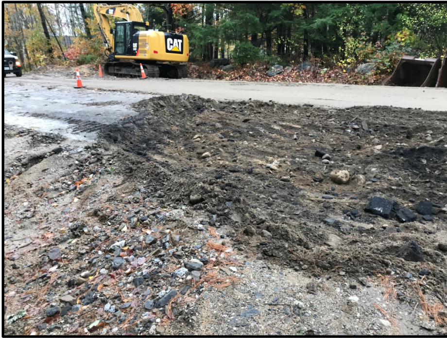
Photograph 5 – Monday, October 30 th – Stripping existing pavement at STA 19+75 on east side of Middle Road.
