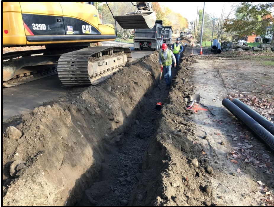
Photograph 9 – Wednesday, November 1 st – Installing 6 inch UD piping on east side of Middle Road STA 26+80 to STA 20+00 to help dewater the area with blasted ledge.
