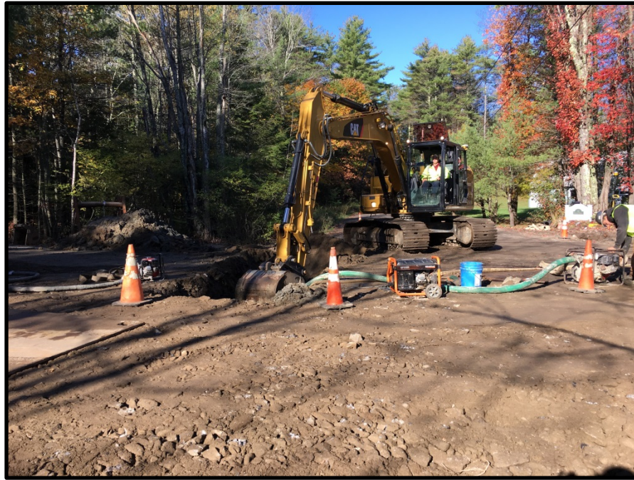
Photograph 3 - Friday, October 27 th – Installing water service for 42 Middle Road.
