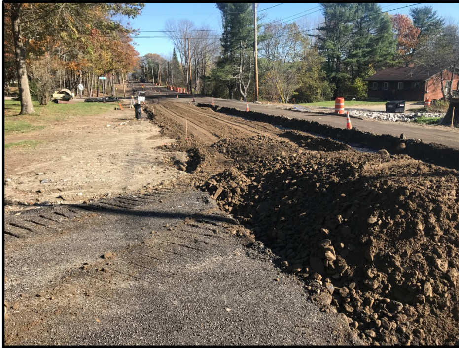
Photograph 7 – Tuesday, October 31 st – Box cut for full depth construction at STA 27+00 on east side of Middle Road.
