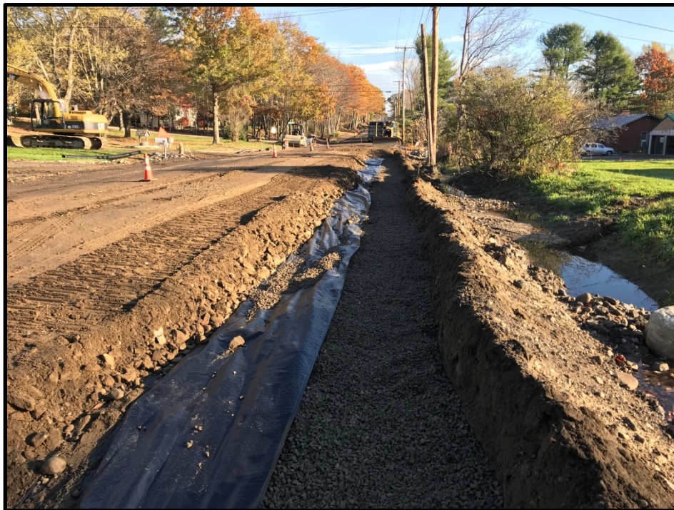
Photograph 10 – Wednesday, November 1 st – Backfilled 6 inch UD on east side of Middle Road STA 26+80 to STA 20+00.
