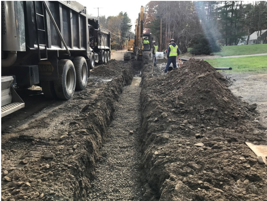
Photo 6 – Installing 6 inch UD on west side of Middle Road STA 26+00.
