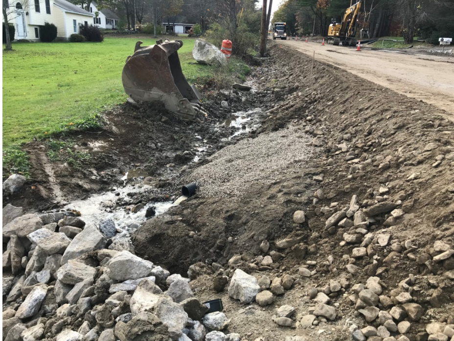
Photo 5 – 6 inch UD outlet after completing installation on east side of Middle Road STA 26+80 to STA 20+80.
