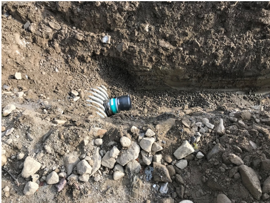
Photo 4 – Inserta tee coupling for 6 inch UD outlet into 18 inch culvert STA 26+80.
