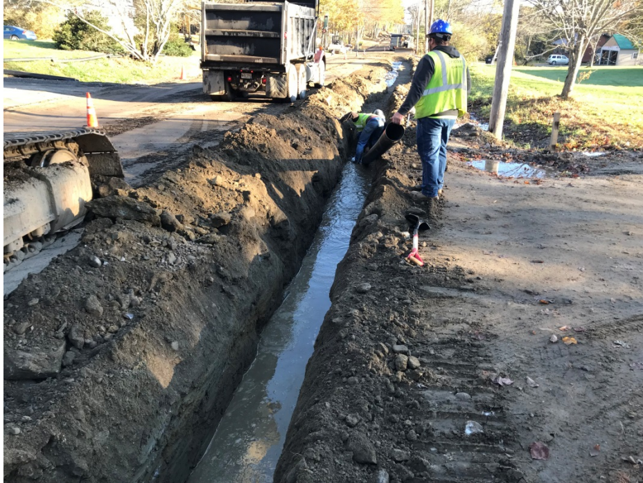
Photo 1 – Installing 6 inch UD in front of Shirley Lane.
