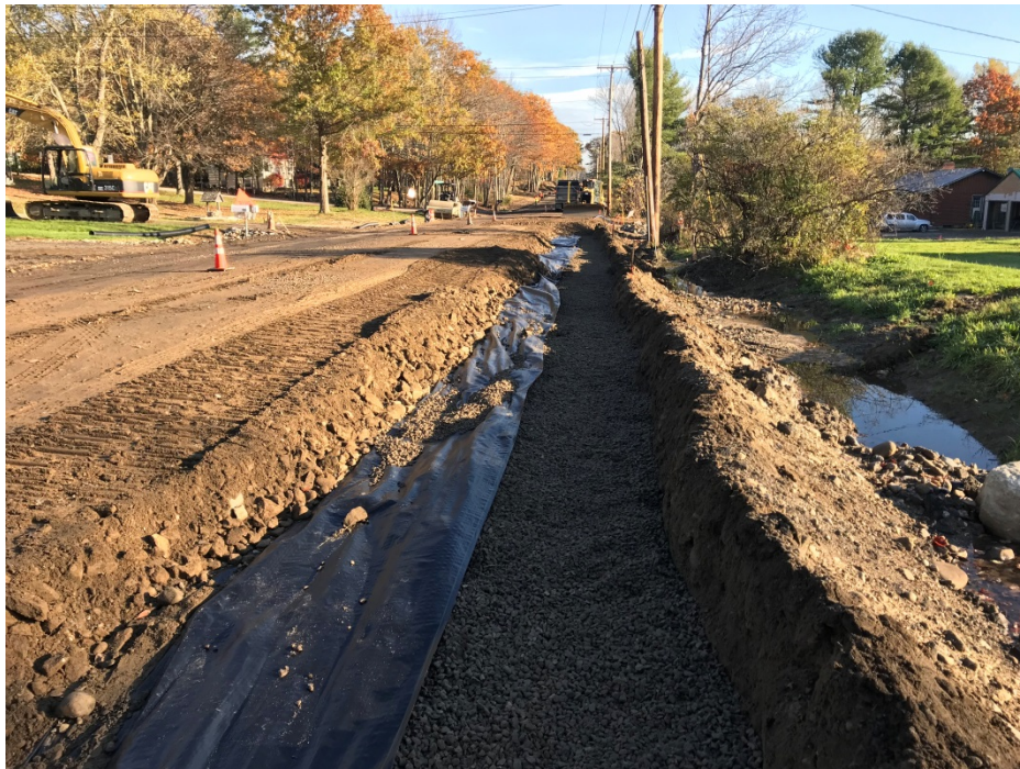
Photo 2 – Backfilled 6 in UD along east side of Middle Road STA 25+00
