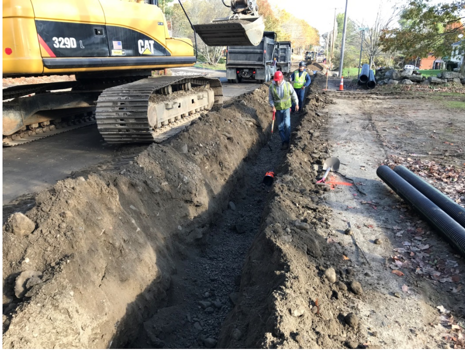
Photo 3 – Installing 6 inch UD at STA 24+00 on east side of Middle Road.
