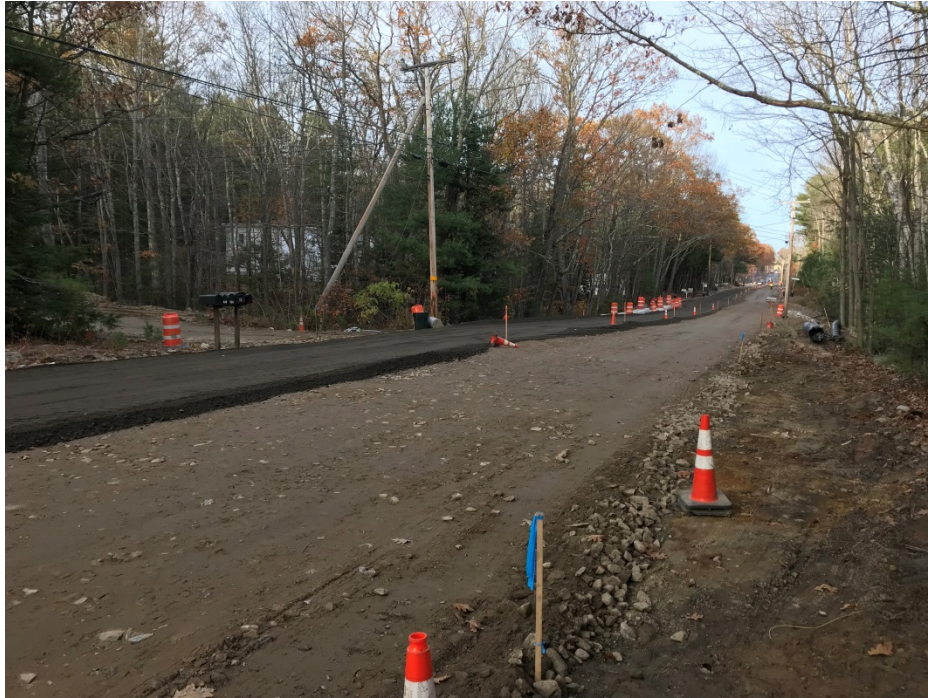
Photo 5 – Reclaim placement on west side of Middle Road.
