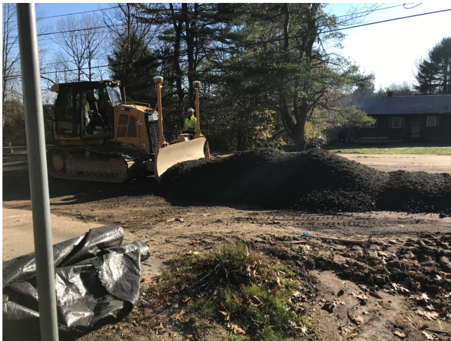
Photo 2 – Placing reclaim STA 27+00.
