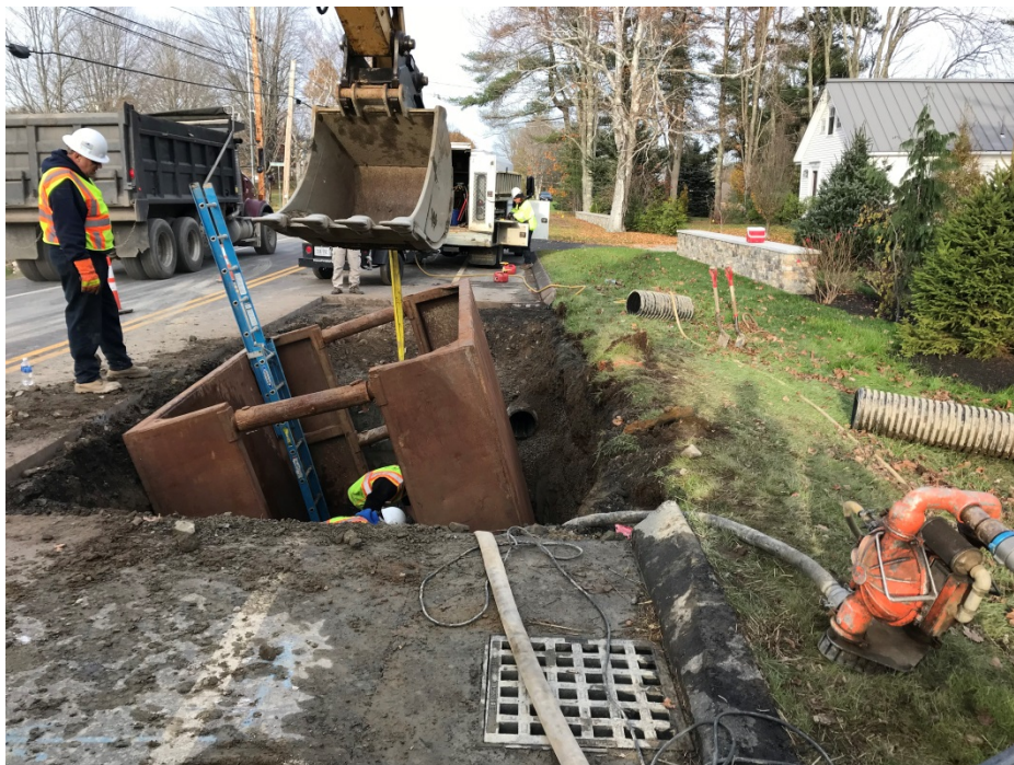
Photo 4 – Area of water main break in front of 125 Middle Road.
