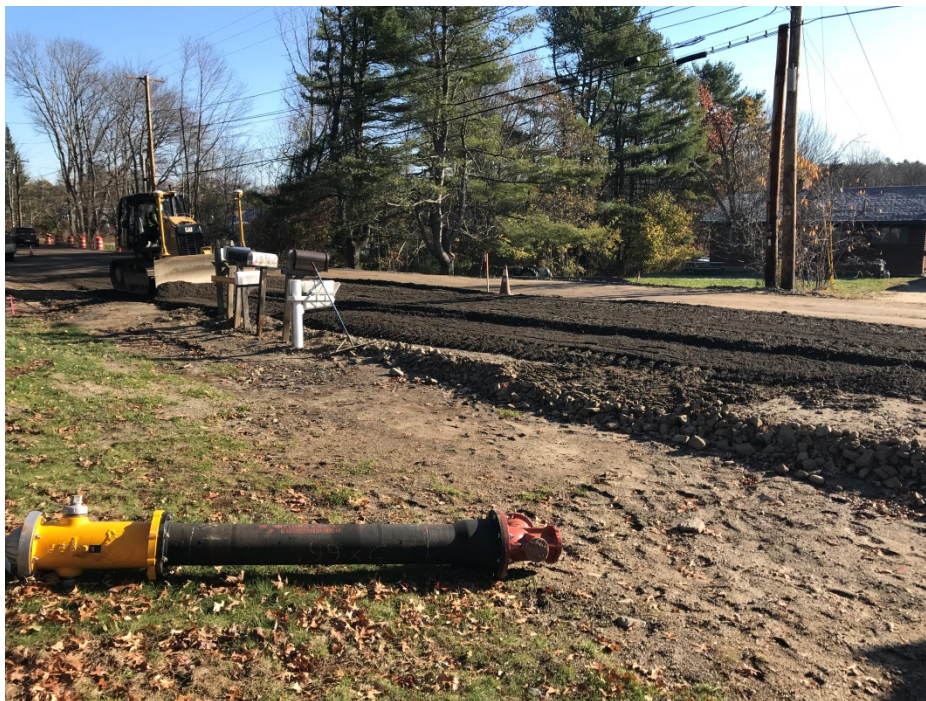
Photo 3 – Grading reclaim to prepare for pavement placement.
