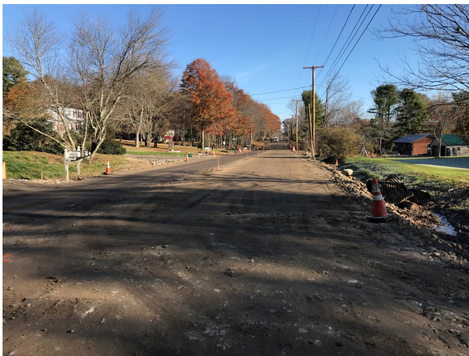
Photo 1 – Grade stakes on center line to begin grading reclaim.
