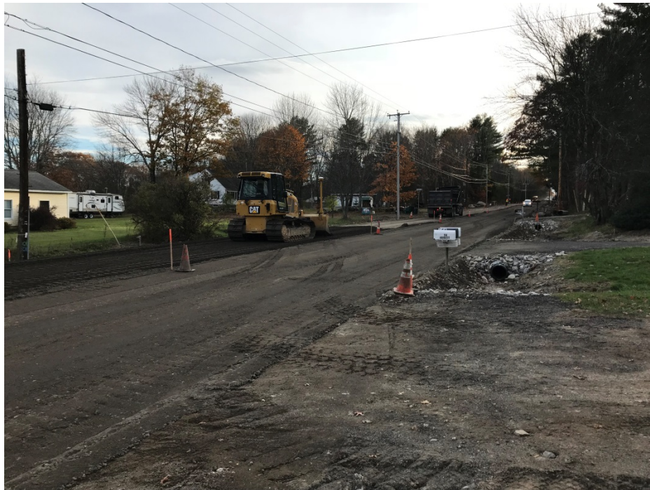
Photo 6 – Placing and grading reclaim on east side of Middle Road STA 25+50.
