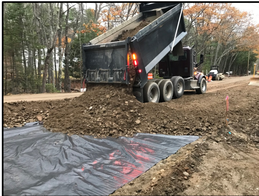
Photograph 8 - Tuesday, November 7 th – Placing subbase gravel STA 16+00 on east side of Middle Road.
