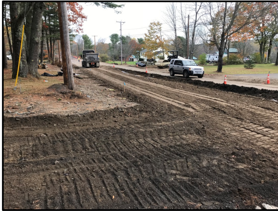
Photograph 3 - Friday, November 3 rd – Placing subbase gravel STA 21+00.
