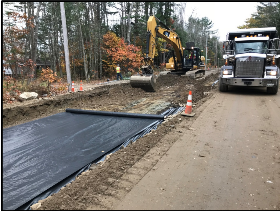
Photograph 4 - Friday, November 3 rd – Working on box cut for full depth construction STA 20+00 on east side of Middle Road.
