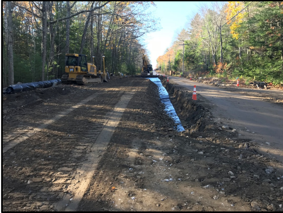
Photograph 9 – Wednesday, November 8 th – Box cut for full depth construction STA 15+00 to STA 14+00. STA 14+00 will be the ending STA for 2017 construction.
