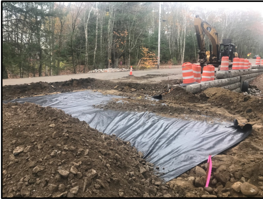
Photograph 5 – Monday, November 6 th – Continuing box cut for full depth construction STA 17+50 on west side of Middle Road.
