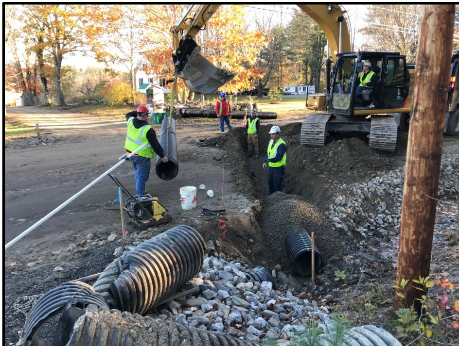
Photograph 10 – Wednesday, November 8 th – Installing the 15 inch corrugate PE cross culvert close to Shirley Lane.
