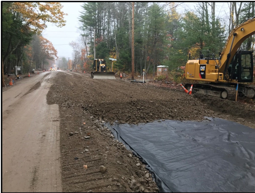
Photograph 6 - Monday, November 6 th – Placing subbase gravel in front of Waterfall Way.
