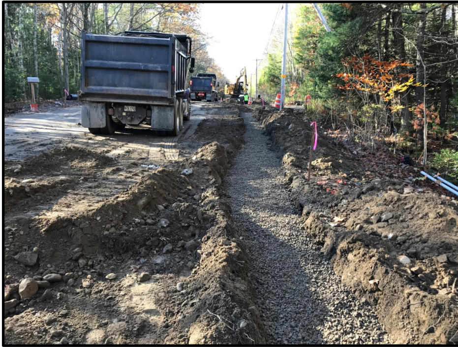
Photograph 7 – Tuesday, November 7 th – Installing 6 inch UD STA 16+40 to STA 13+00 on west side of Middle Road.
