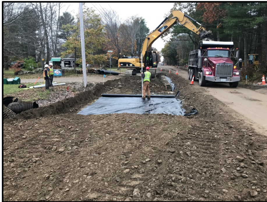
Photograph 2: Thursday, November 2 nd – Working on box cut for full depth construction STA 23+50.
