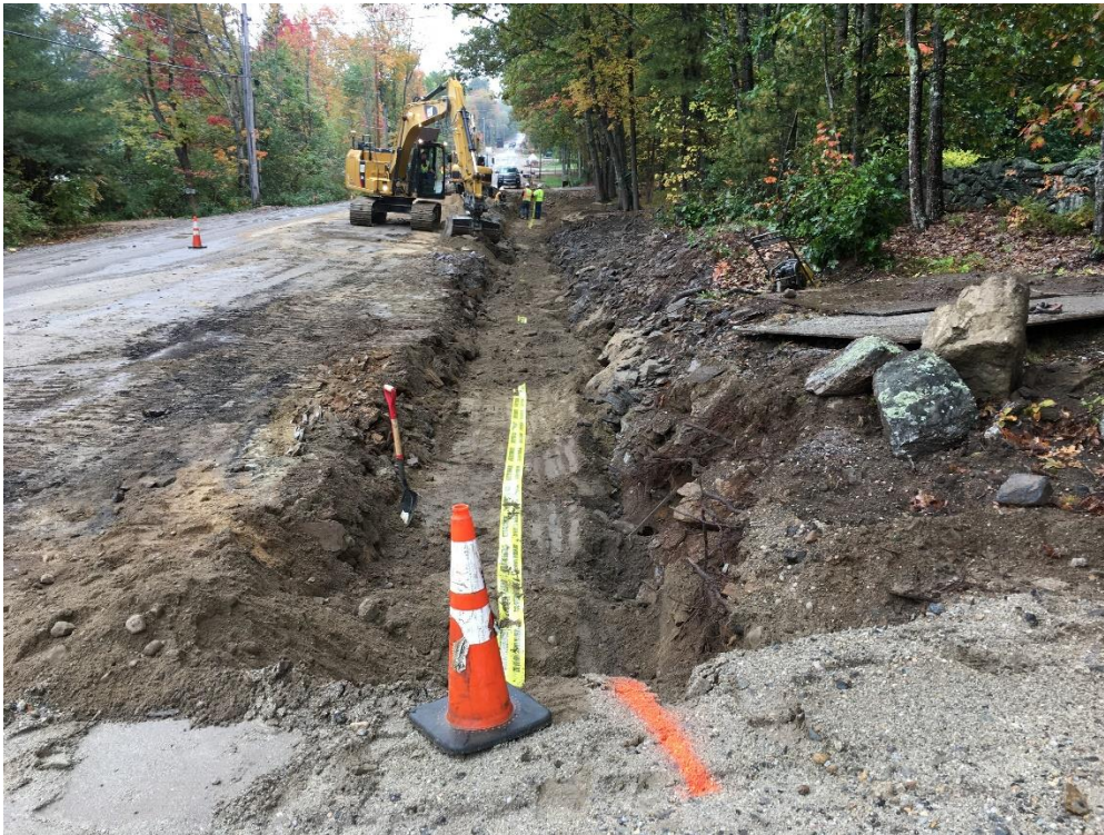
By mid-afternoon the crew was backfilling gas trench using 2 excavators to place sand over the gas main (in the background) followed by second excavator backfilling to grade for drainage swale with native material.
