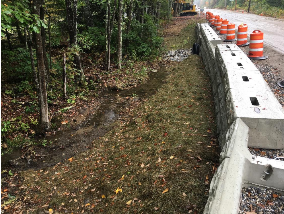
Flow through the stream bed along the retaining wall to the inlet of the new 42-inch culvert. Flow is from flushing of the hydrant at Evergreen Lane and about ½ inch of rain.
