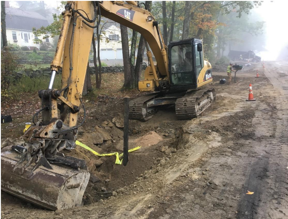
End point of 240 feet of gas main installation (4x4 post at STA 32+20). Afterwards, crew shaped drainage swales, installed culverts under the 2 affected driveways and re-positioned mailboxes in the work area.
