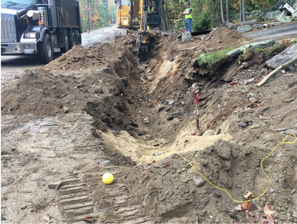
Initial excavation to extend the natural gas main further southward from 70 Middle Road.
