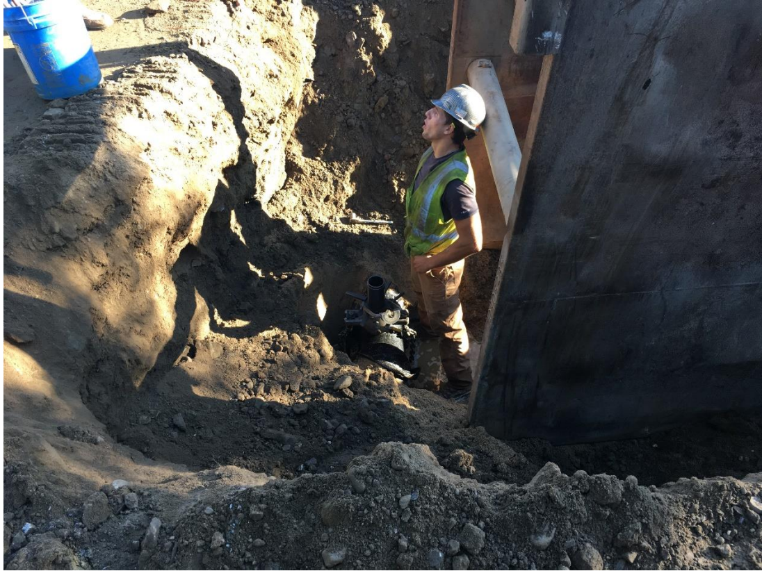
Preparing to tap the 12-inch water main extension to receive the 1-inch corporation stop valve and copper water service line.
