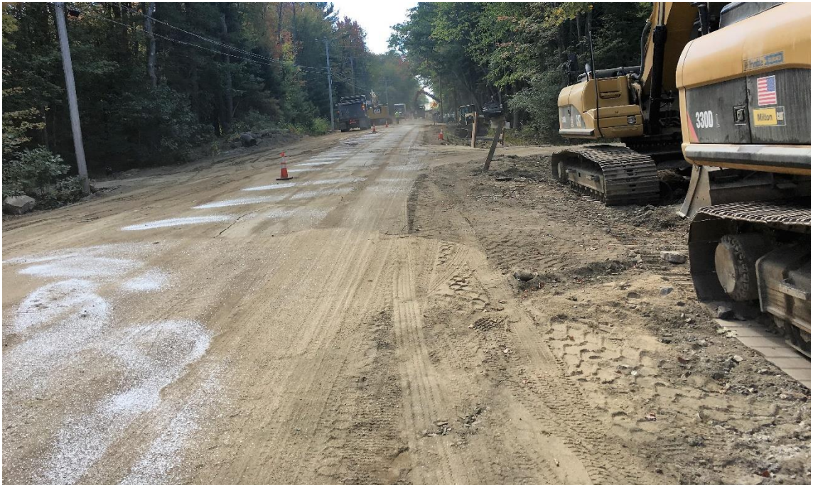
Overall work zone. Unloading retaining wall block to the right of the road and installing a "short side" water service at Waterfall Way on the left side of the road. In the foreground, freshly broadcasted calcium chloride for dust control on the left and idle excavators parked on right.
