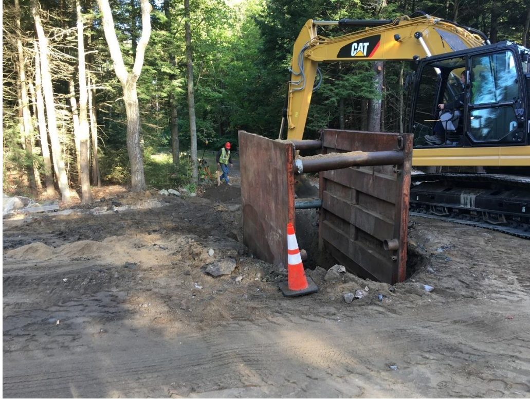
Began the day installing the "long side" water service at 38 Middle Road working back from the curb stop to the main across the road.
