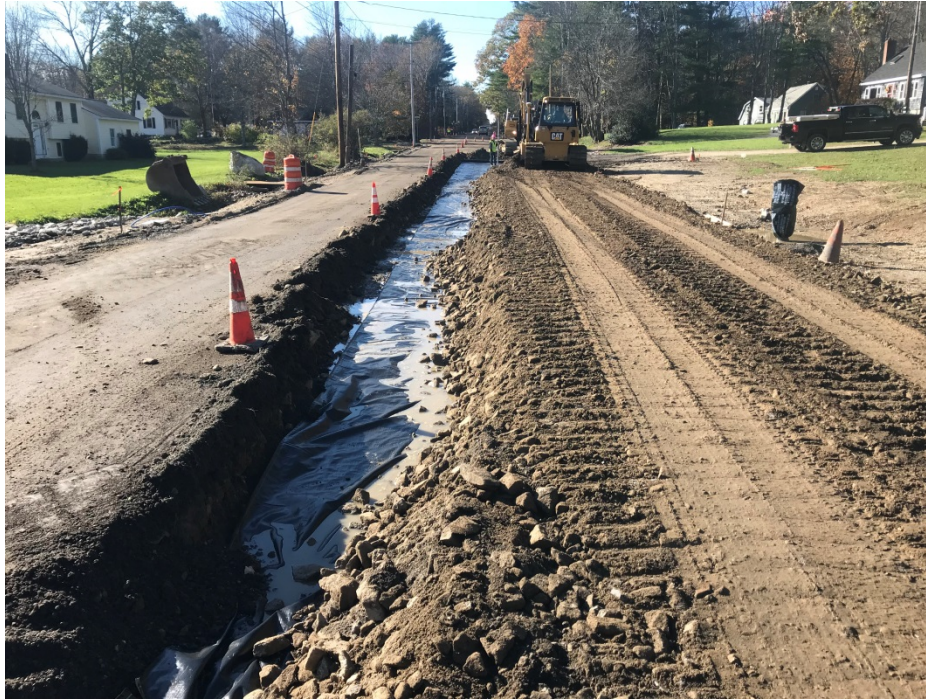
Photo 3 – Box cut for full depth construction on west side of Middle Road.
