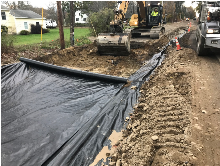
Photo 6 – Box cut for full depth construction on east side of Middle Road.
