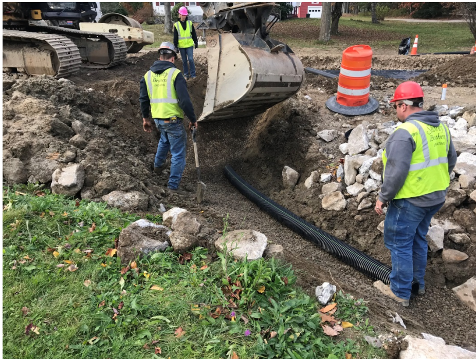
Photo 4 – Installing 6 inch UD at STA 26+75 to daylight into rip rap swale.
