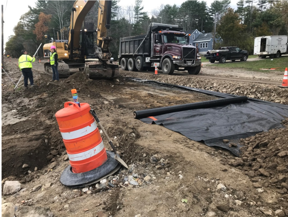
Photo 5 – Continuing box cut for full depth construction on east side of Middle Road STA 26+00.
