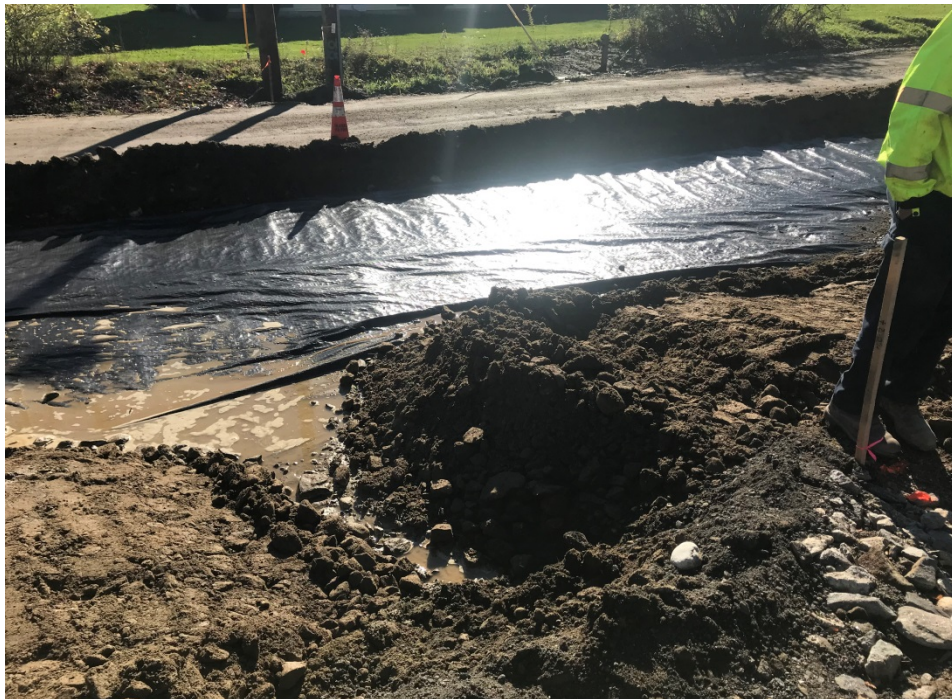
Photo 2 – Placing woven fabric on subgrade. Water is entering the box cut from the adjacent driveway. The new 6 inch UD will be installed through this location.
