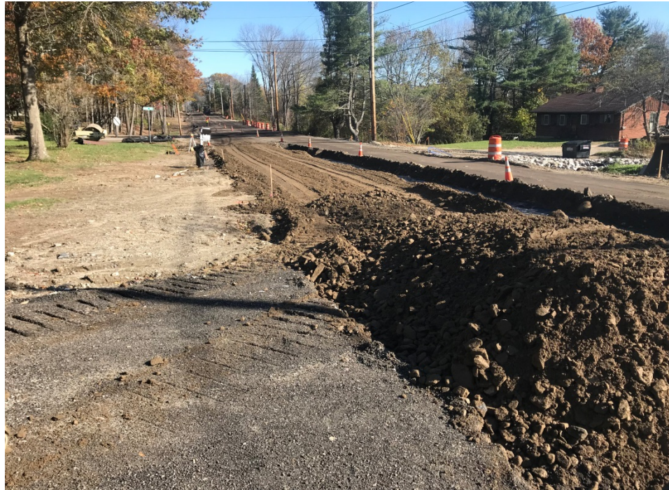
Photo 1 – Actively working on box cut for full depth construction, STA 26+00 headed southward on west side of Middle Road.
