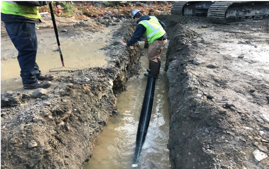
Photo 6 – Installing 6 inch UD at STA 20+75. This helped dewater the water main trench.
