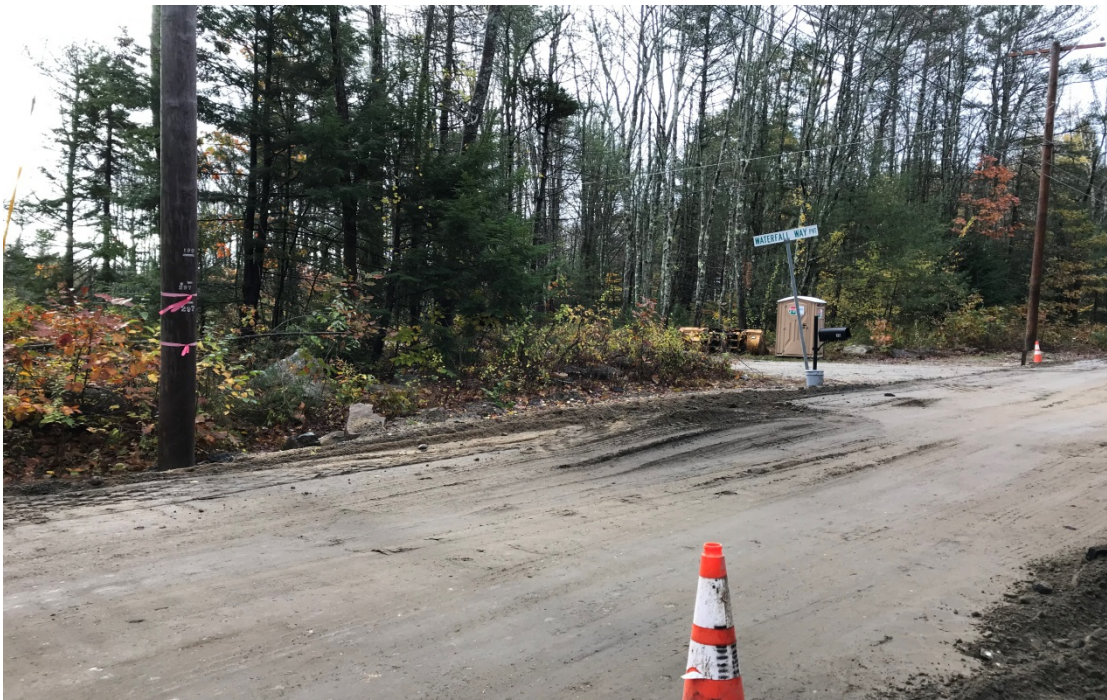
Photo 2 – Soft area found over water main trench at STA 19+50. Water from the rain event seems to be traveling through veins in the ledge. 6inch UD was installed just below this spot, per plans, and this began dewatering the area.
