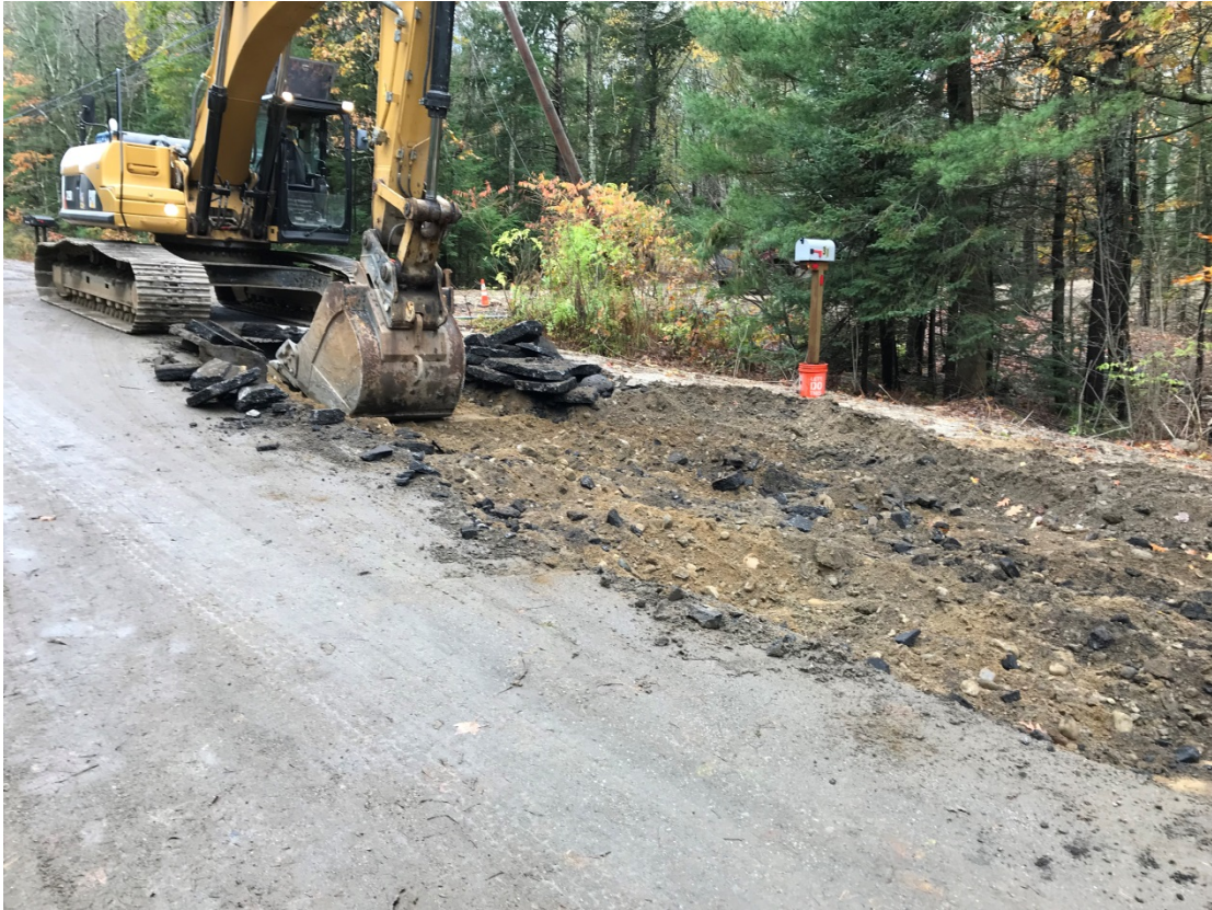
Photo 5 – Stripping existing pavement on west travel lane of Middle Road.
