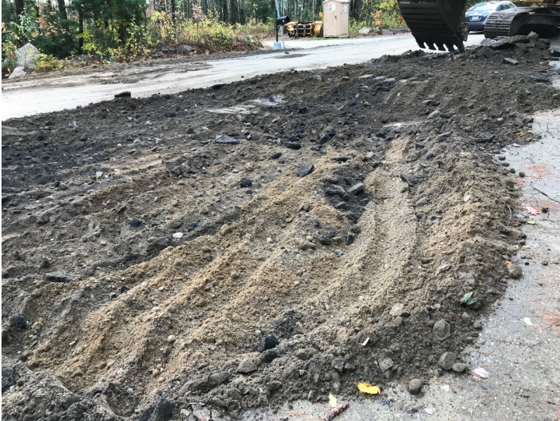
Photo 1 – Stripping existing pavement in west travel lane at STA 20+00
