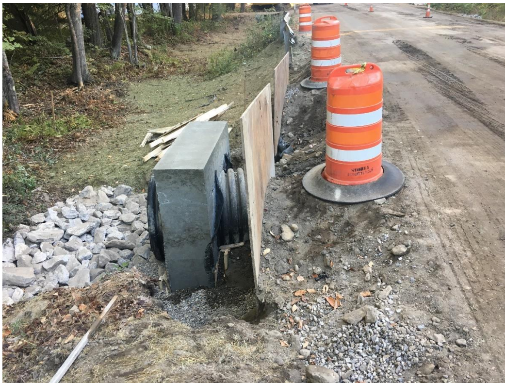
Form removed from cast-in-place headwall for culvert at STA 17+00.
