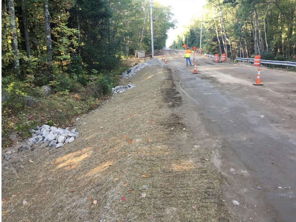
Example of erosion control measures. Here mulch placed on disturbed areas and stone check dams placed along drainage routes.
