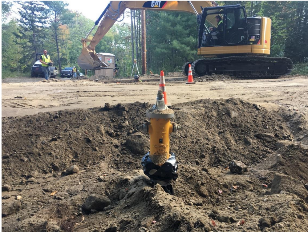
Completing the connection of the "long side" hydrant at STA 19+05 across from Waterfall Way.
