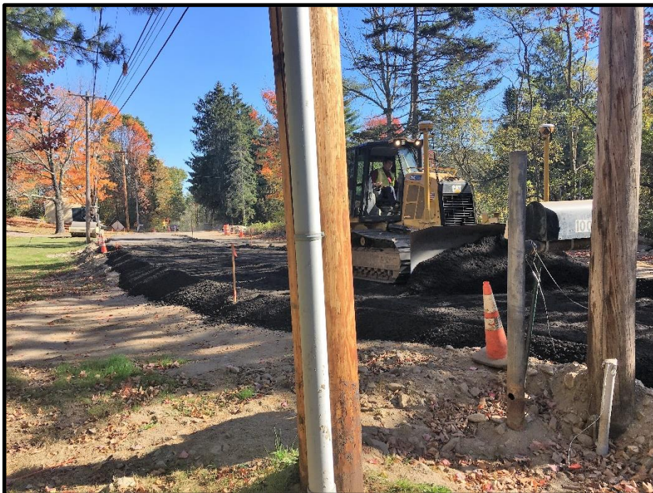
Photograph 4 - Friday, October 20 th – GPS equipped dozer and laser measured grade stakes used to set road to proper grade. Crew placed surface gravel for 900 feet of roadway to STA 40+50 just south of Storey Brook Lane.
