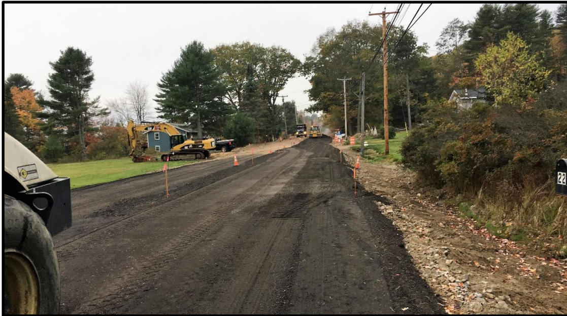
Photograph 5 – Monday, October 23 rd – Began the day at STA 40+50 placing surface gravel (pavement millings) in the southbound lane in a southerly direction.
