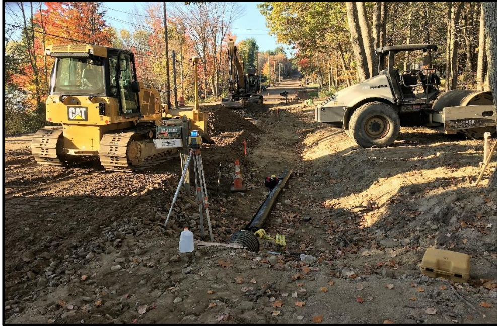
Photograph 1 – Thursday, October 19 th - Began the box cut at STA 32+75 (south edge of 62 Middle Road Driveway) in the southbound lane working southward.
