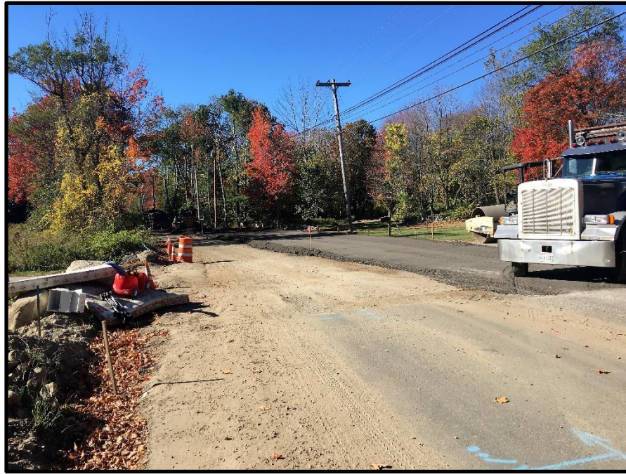
Photograph 3 - Friday, October 20 th – Began the day at STA 49+50 placing surface gravel (pavement millings) in the southbound lane in a southerly direction.
