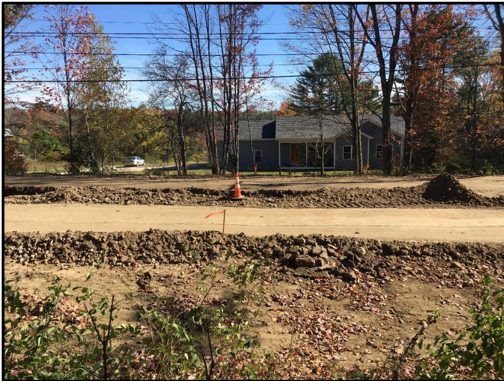
Photograph 2: Thursday, October 19 th - Southern end of the day's box cut at STA 31+00 in front of 57 Middle Rd. (meeting up with 400-foot section previously box cut to STA 27+00). Crew then switched to east side of the road at STA 32+75 and worked southerly to match up to this point.
