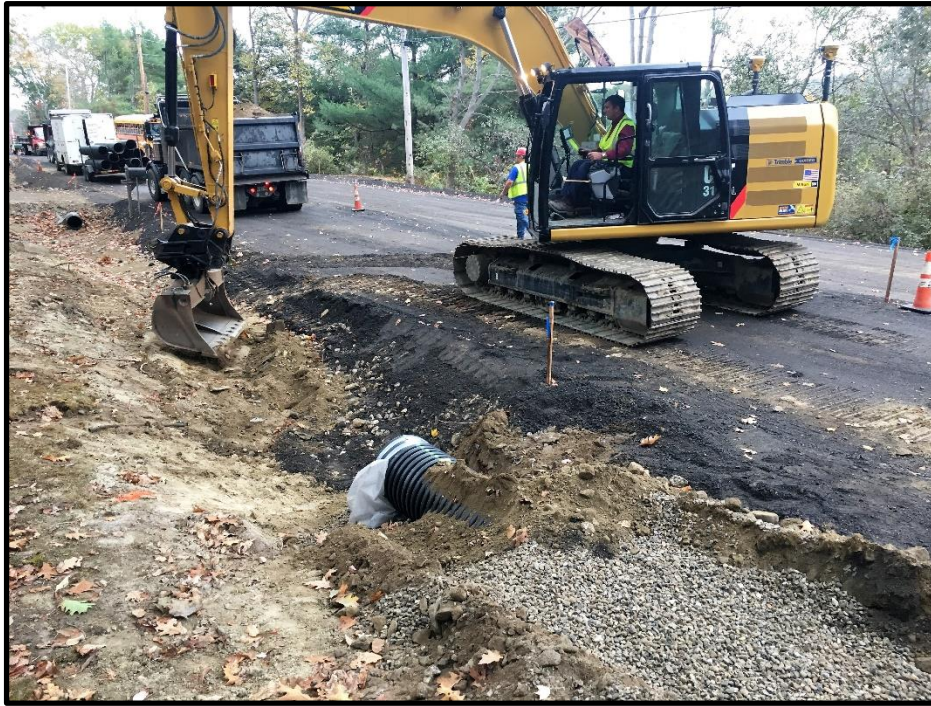
Photograph 7 – Tuesday, October 24 th - Shaping drainage swale between culvert installations.
