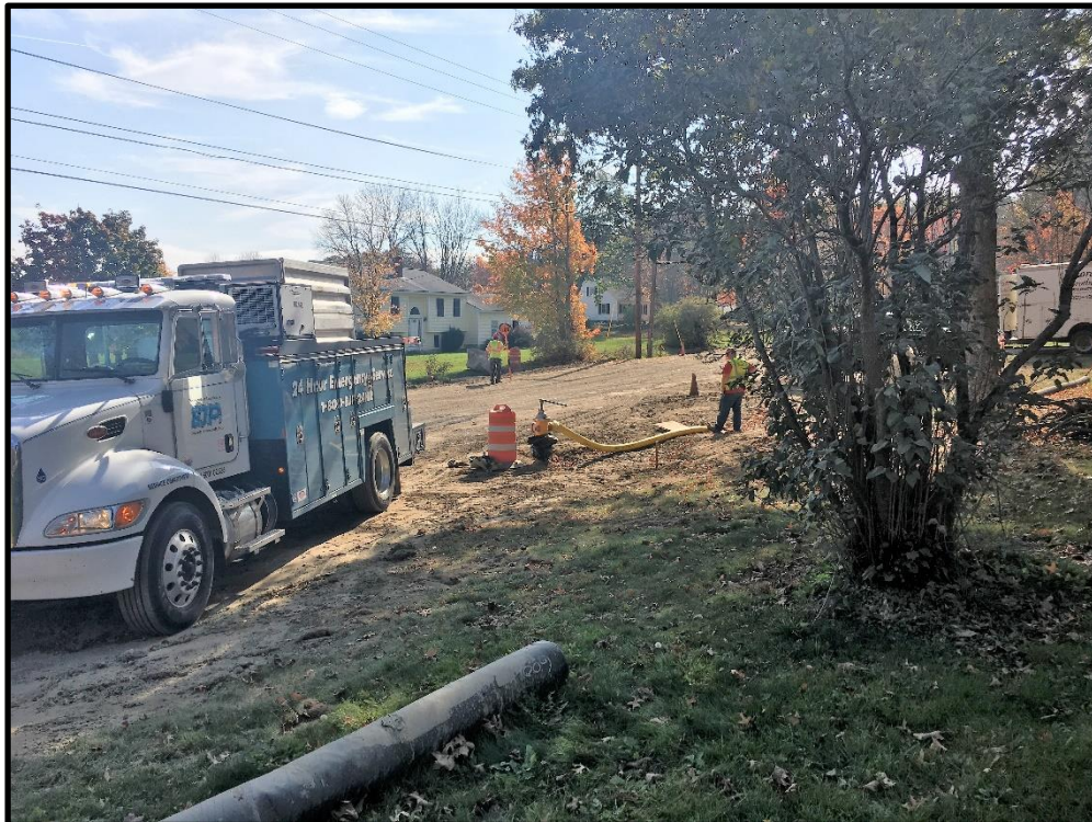
Photograph 6 - Monday, October 23 rd - Flushing at the Hydrant at STA 27+00. Flow is directed to the catch basin in front of 54 Middle Road which discharges to the drainage easement at 55 Middle Road.
