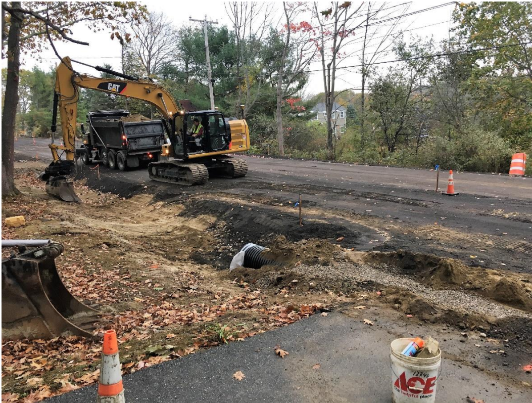
Photo 2 – Shaping drainage swale between culvert installations.
