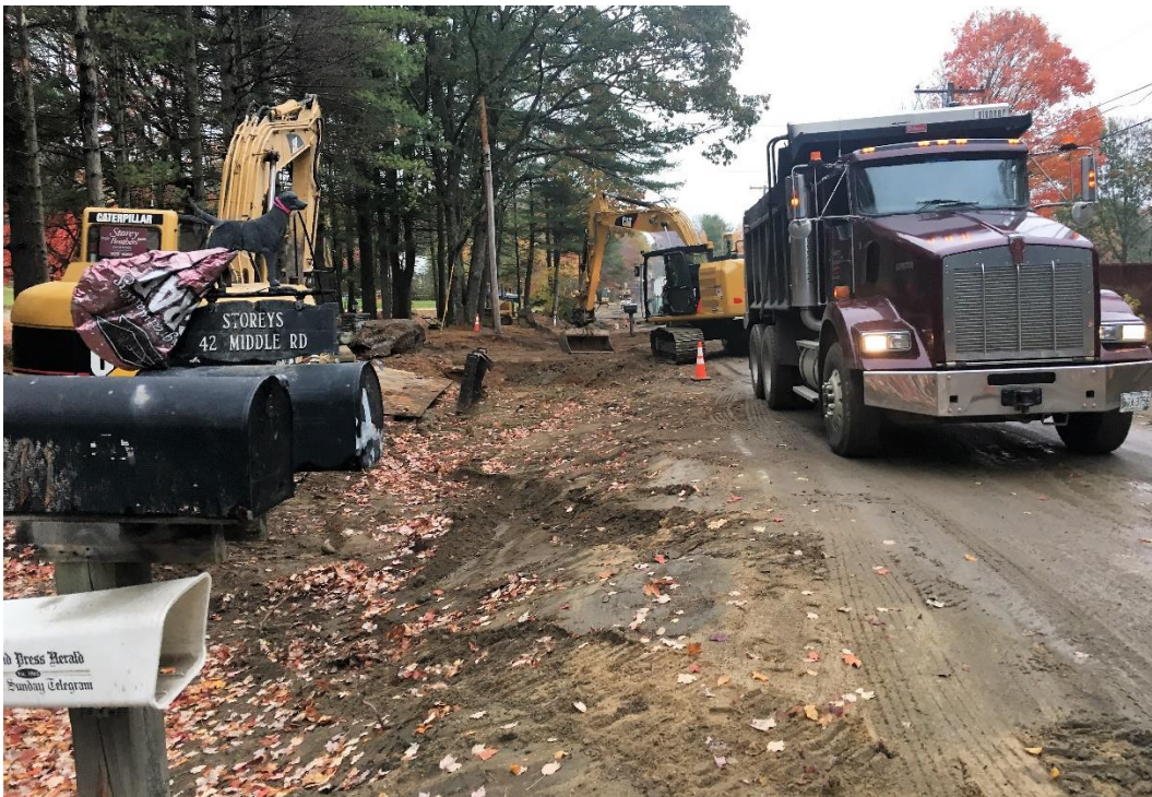
Photo 4 – Crew installed driveway culverts from STA 32+00 to STA 18+00 along the west side of the road. Here installing culvert at 44 Middle Road near STA 23+00.
