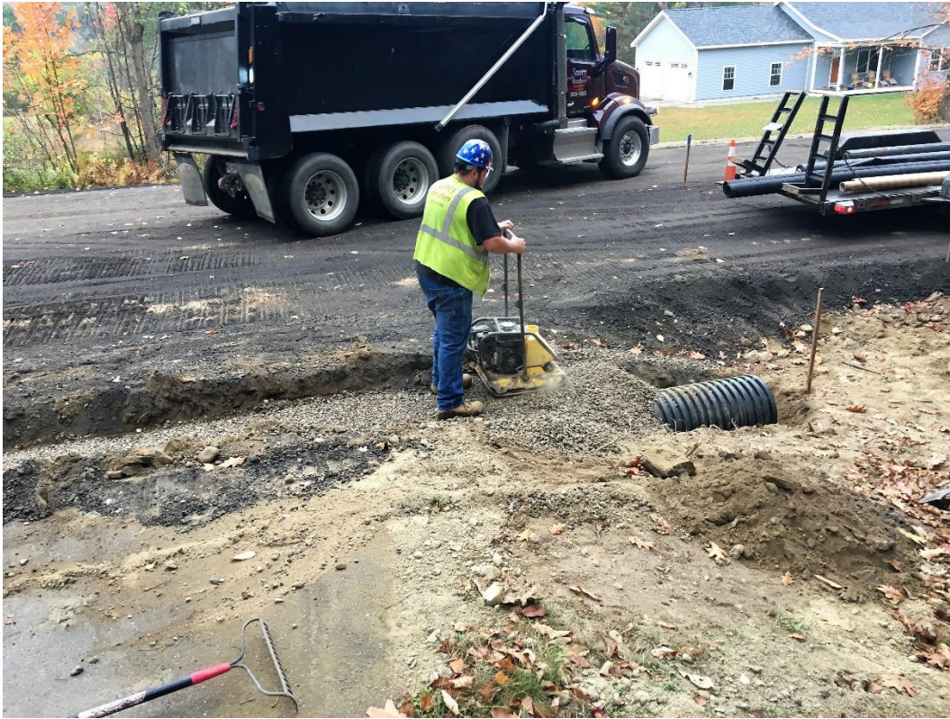
Photo 3 – Using a plate compactor to bed the crushed stone around and over the driveway culvert prior to placing gravel.
