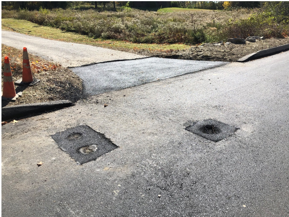
Photo 4 – Valve stem adjustments
