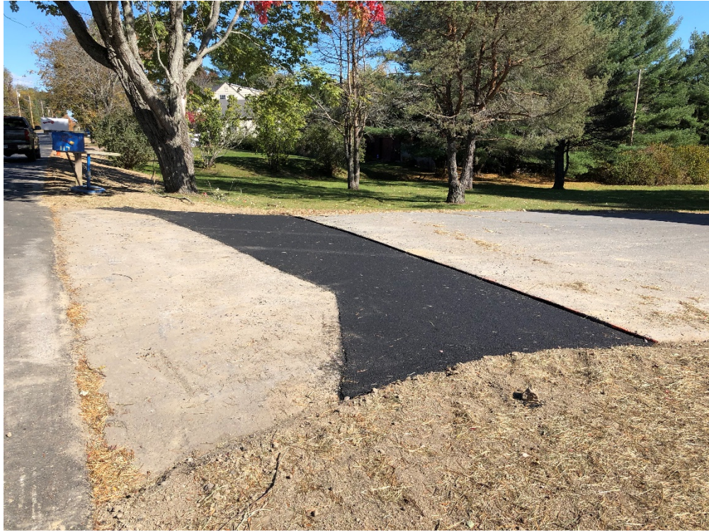
Photo 3 – Driveway repair at water line crossing
