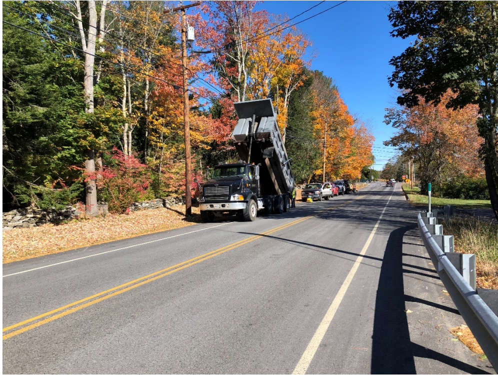
Photo 1 – Placing pavement for driveway apron
