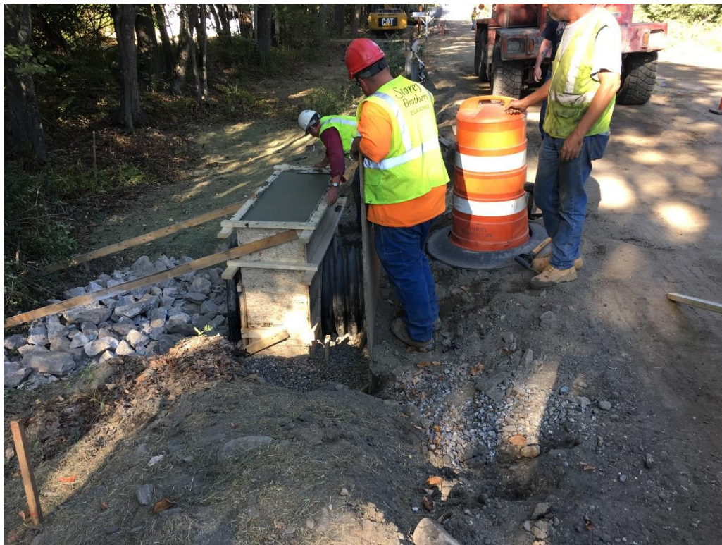
By 3:15 PM, the concrete was placed in the form and troweled to a smooth finish.
