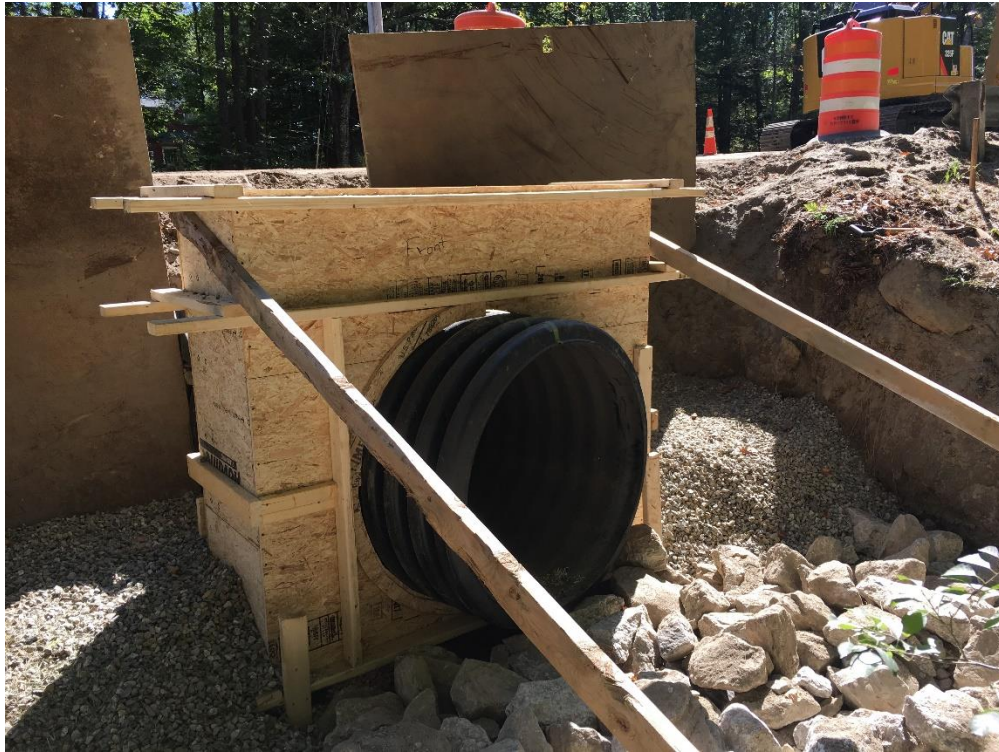
Form constructed in the morning for the cast-in-place concrete headwall.
