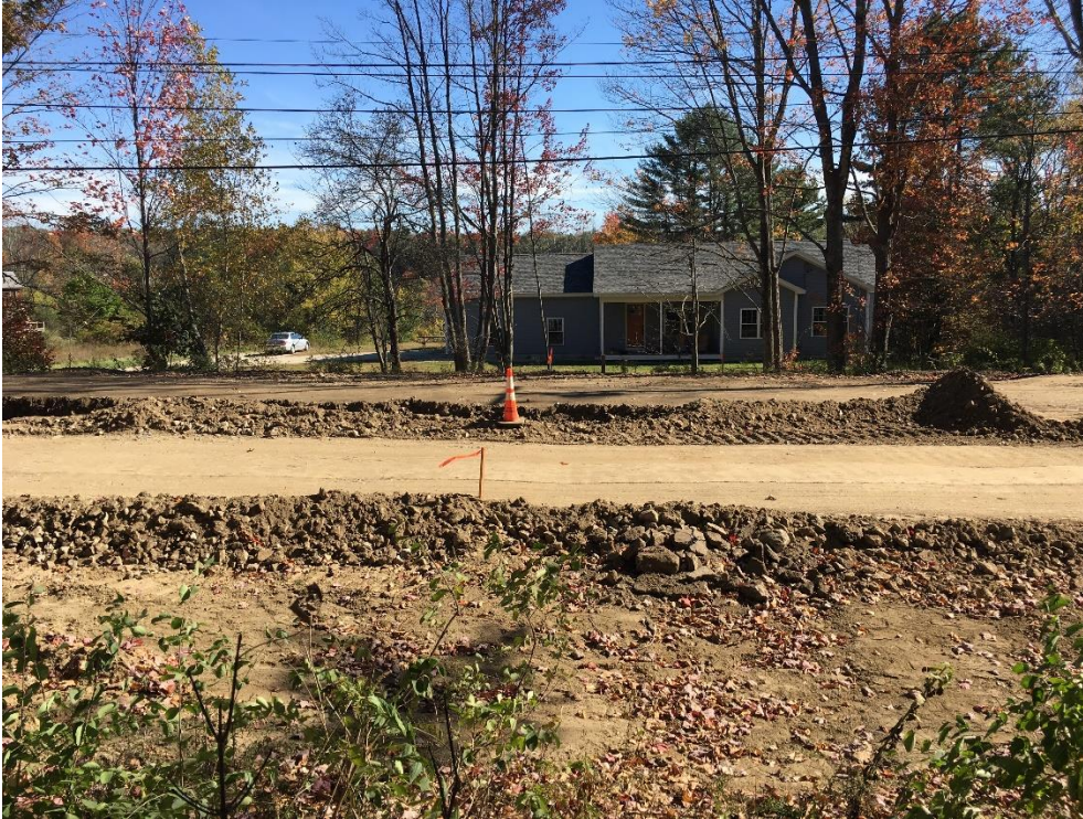
Photo 3 – Southern end of the day's box cut at STA 31+00 in front of 57 Middle Rd. (meeting up with 400-foot section previously box cut to STA 27+00). Crew then switched to east side of the road at STA 32+75 and worked southerly to match up to this point.
