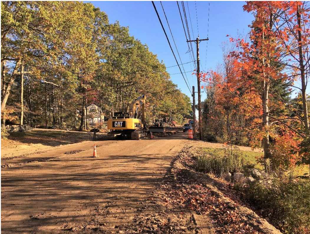
Photo 2 – Box cutting and placing new base gravel at STA 31+75 along the west side of the road (in front of 58 Middle Road) approaching the southern end of the day's box cut at STA 31+00.
