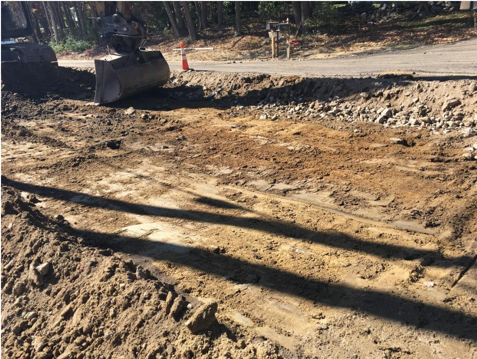
Photo 4 – View of subgrade at STA 31+50 showing a hard, dry silty clay in the northbound lane near the end of the day. This was typical for the day.
