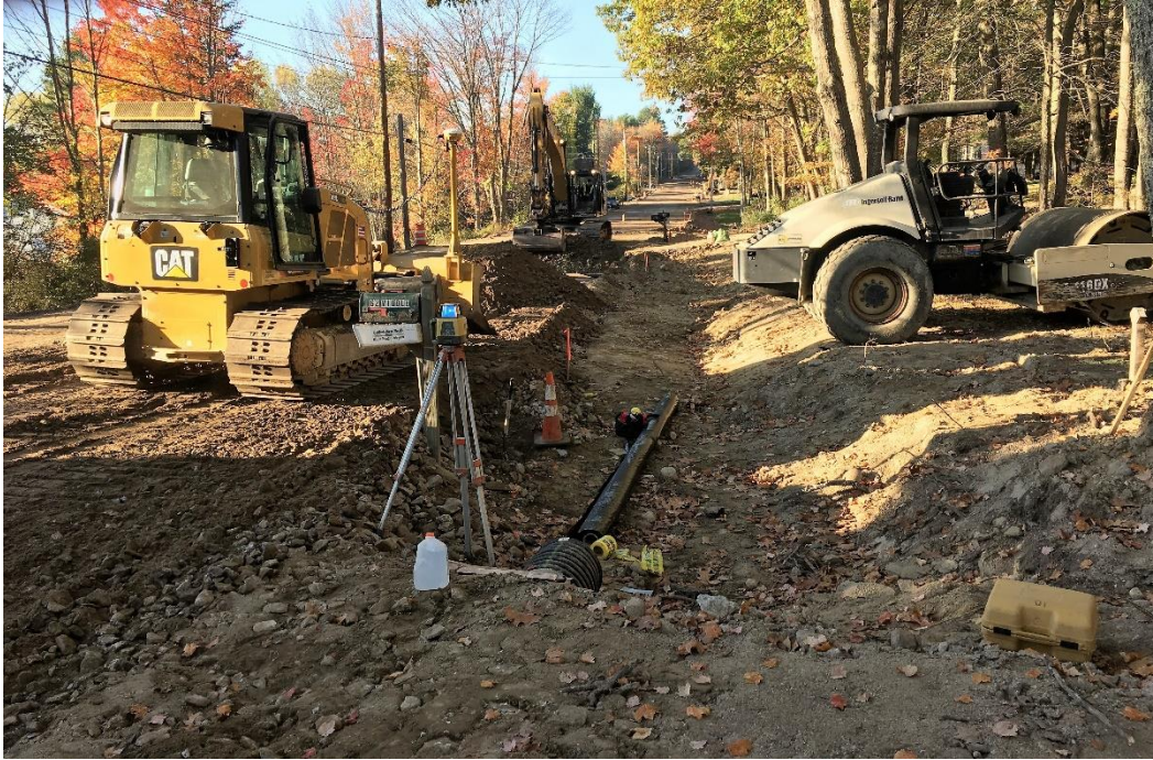
Photo 1 – Began the box cut at STA 32+75 (south edge of 62 Middle Road Driveway) in the southbound lane working southward.
