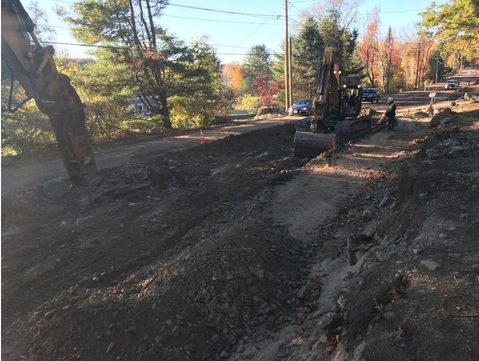
Photo 3 – South of the ledge hump in Photo 1, the subgrade was approximately the top of ledge to approximately 70 Middle Road where the subgrade transitioned to a firm dry silty tan clay.
