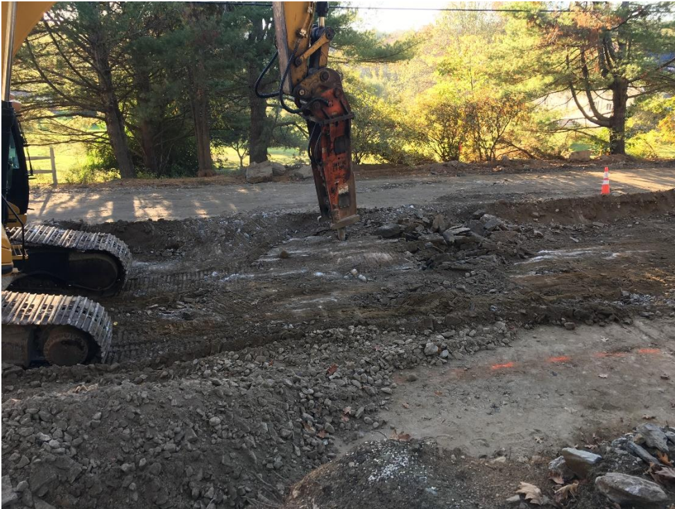
Photo 2 – Early into the box cut a small mound of ledge was encountered near the center of the road at STA 35+25. The size of the mound was approximately 20'x7'x1' and yielded fairly quickly to the hoe ram given the earlier blasting along each edge of the road for water and underdrain/gas.
