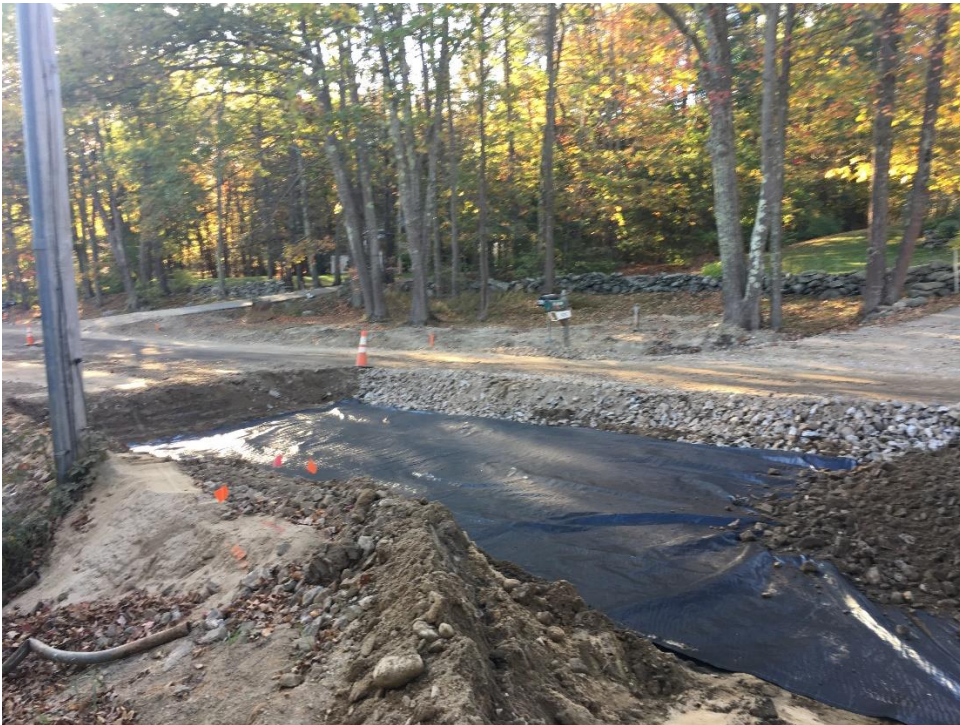
Photo 4 – At the end of the day the box cut finished up on the east side of road at STA 32+75 to match up with the west side near the southern edge of the 62 Middle Road driveway.
