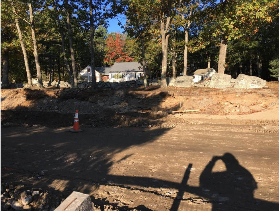
Photo 1 – Began the box cut at STA 35+50 (south edge of 72 Middle Road Driveway) in the southbound lane working southward.
