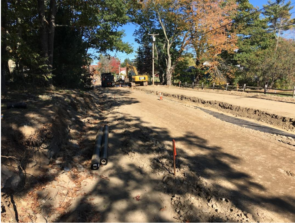
Photo 3 – In the afternoon the crew switched to the northbound lane to box cut and place new gravel in a southerly direction to match up with the southbound lane to STA 35+50 excavated in the morning.
