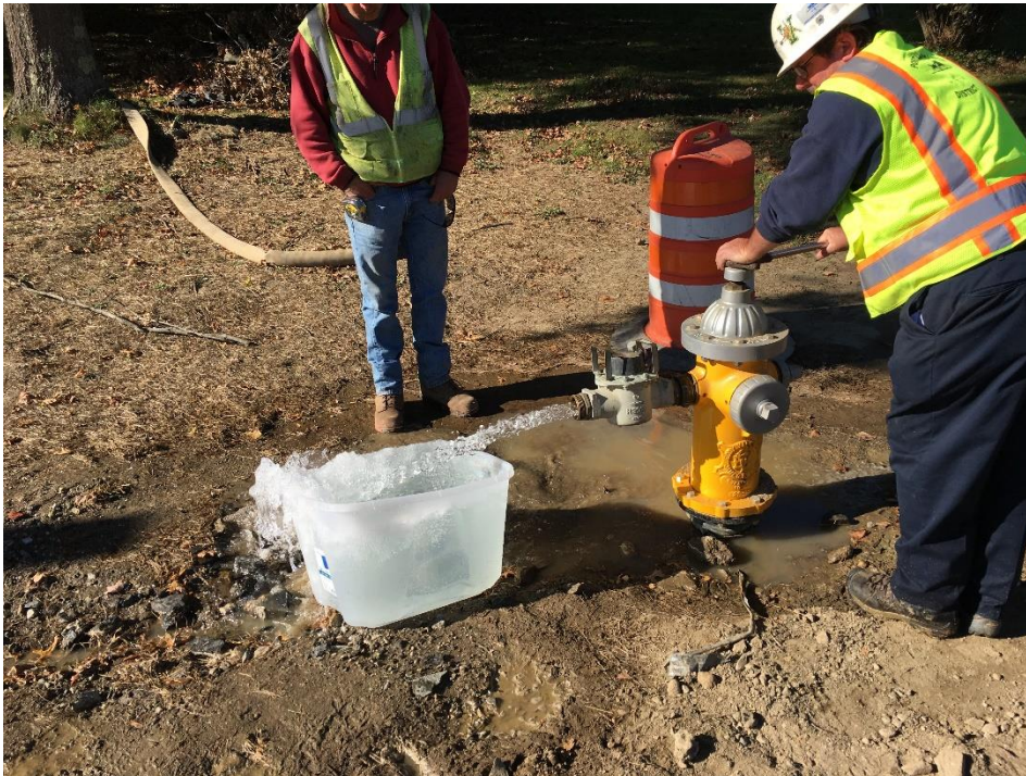
Photo 4 – Rob Story (Storey Brothers) and Jeff McGill (Portland Water District) flushed and visually inspected the water from the hydrant at STA 27+00 (54 Middle Road). After brief discoloration, the flush became clear and did not return after a second flush. It is planned to excavate and inspect the hydrant branch.
