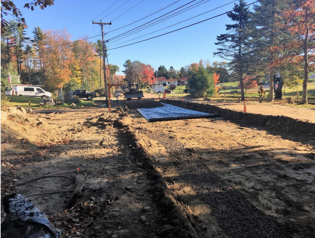
Photo 1 – Initial placement of new gravel at the beginning of the day at STA 39+00 over geotextile fabric following the box cut of the existing gravel. Crushed stone trench of the previously installed 6-inch underdrain in the foreground.
