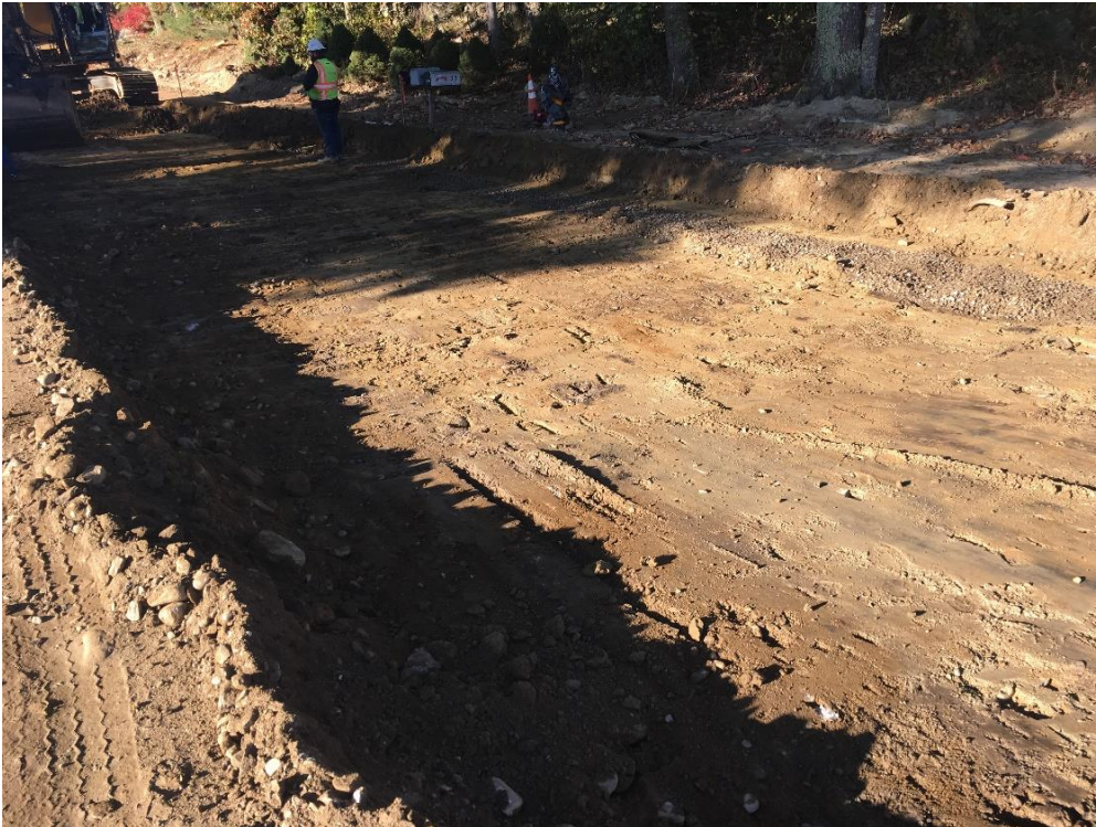
Photo 2 – View of the road subgrade in the vicinity of STA 38+00. Subgrade a stiff dry consolidated silty clay.
