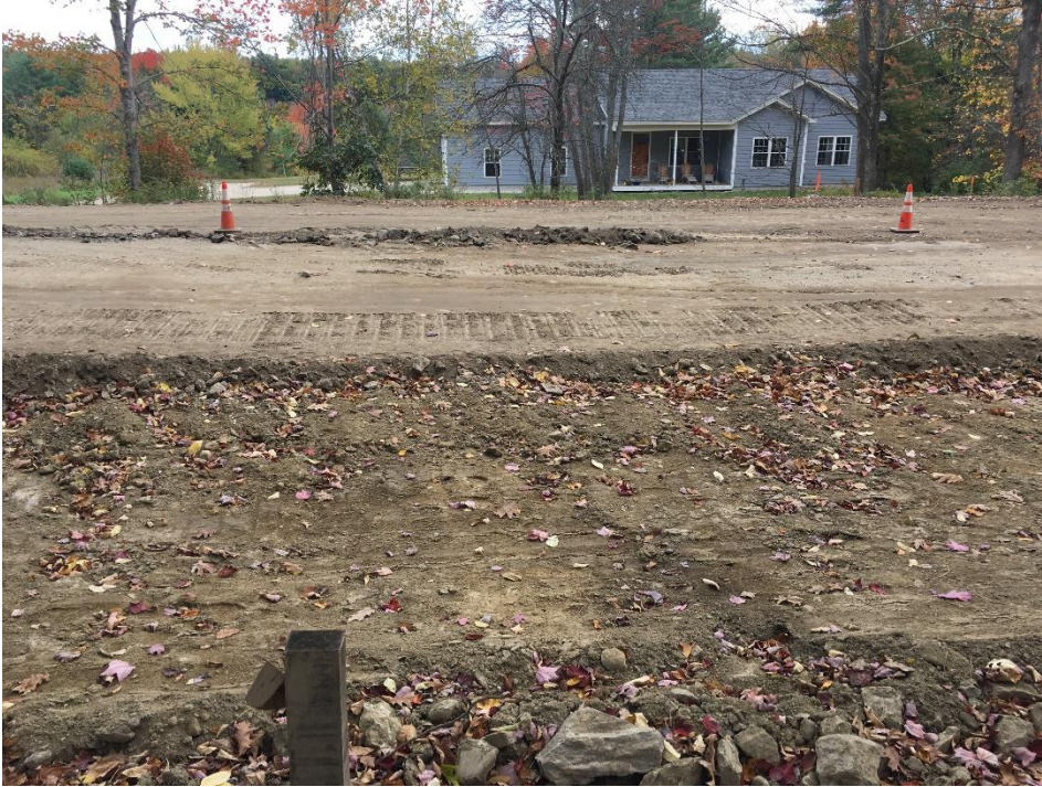
Photo 3 – Crew removed pavement to STA 31+00 (in front of #57 Middle Road) to meet up with the section that was previously box cut and new gravel placed.
