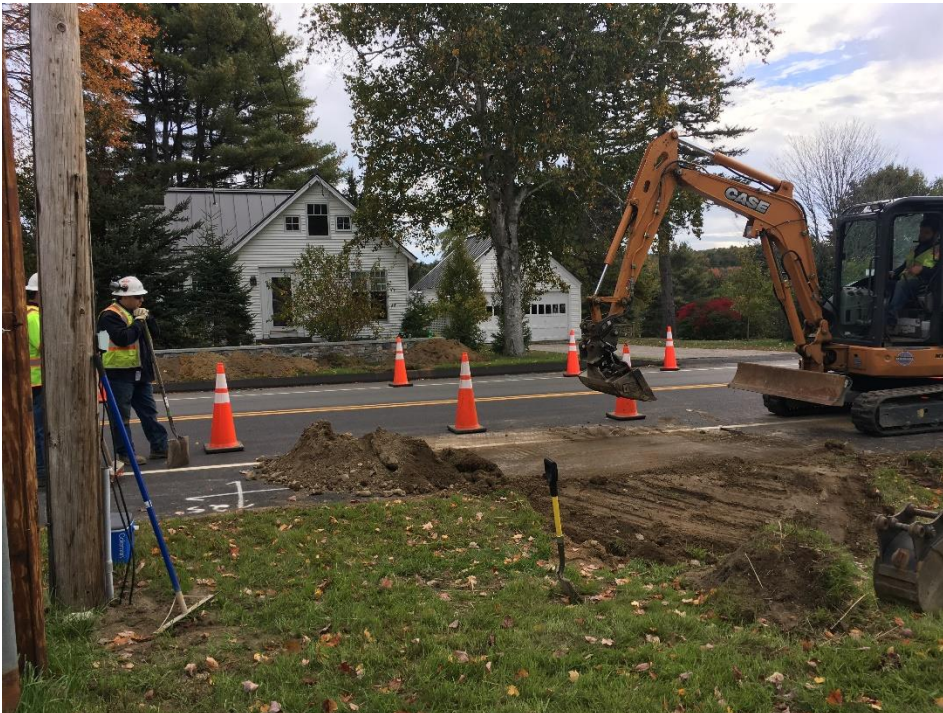
Photo 4 – Summit completing the backfilling after making the connection of the gas service line for #129 Middle Road to main across the road near Butterworth Farm Road.
