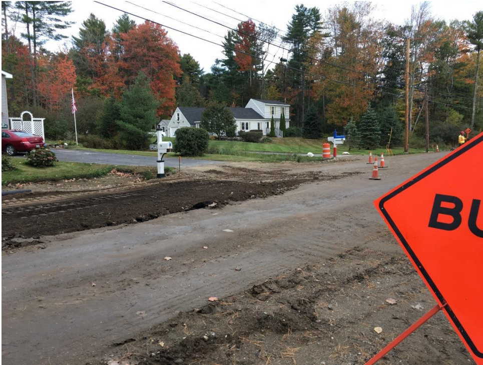
Photo 1 – Crew began the day stripping pavement in the southbound lane at STA 39+00 (south of #78 driveway) in a southerly direction.
