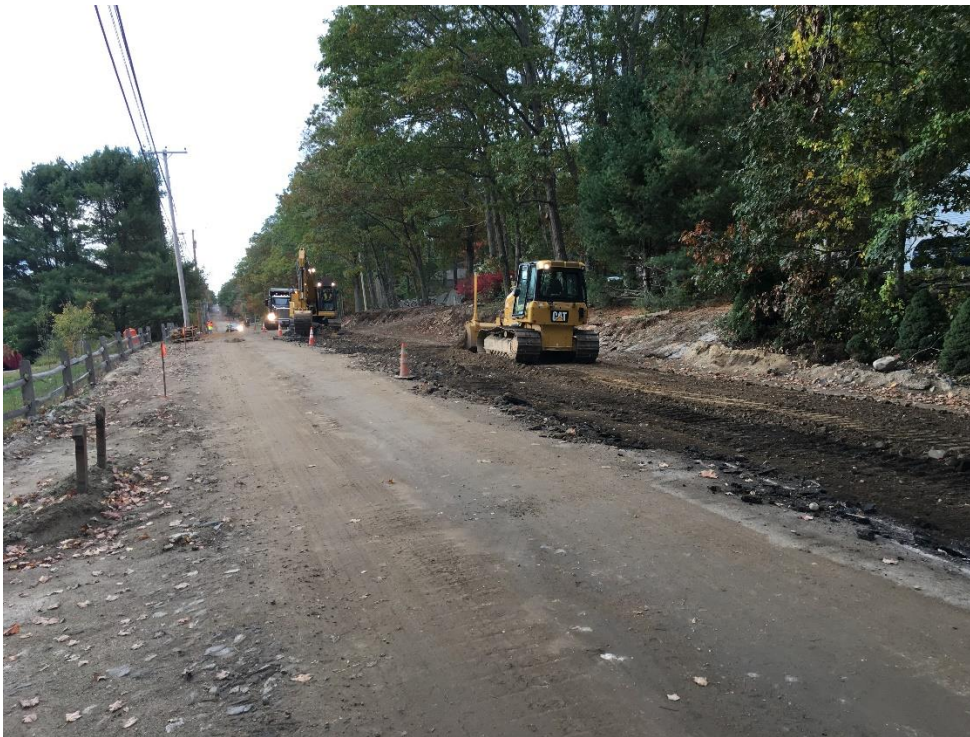
Photo 2 – General depiction of pavement stripping operation. Excavator strips pavement from top of existing gravel and loads into truck. Dozer follows to gather additional chunks of pavement to be trucked away and re-establish a temporary road grade that is then re-compacted with a roller to receive vehicle traffic.
