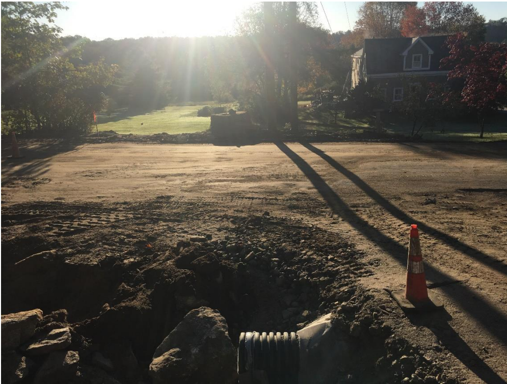
Photo 2 – While installing underdrain the crew also replaced driveway culverts along the route. Above is the inlet of the driveway culvert for 70 Middle Road. Across the road is the stump of the large oak tree next to Pole #307 in front of 67 Middle Road.
