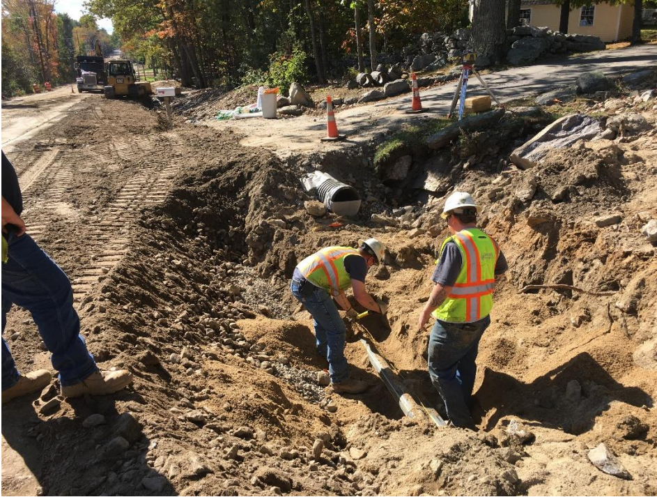
Photo 3 – Summit in front of 72 Middle Road (STA 36+00) preparing to bring the rest of the installed gas main online southward to 31 Middle Road (STA 14+00).
