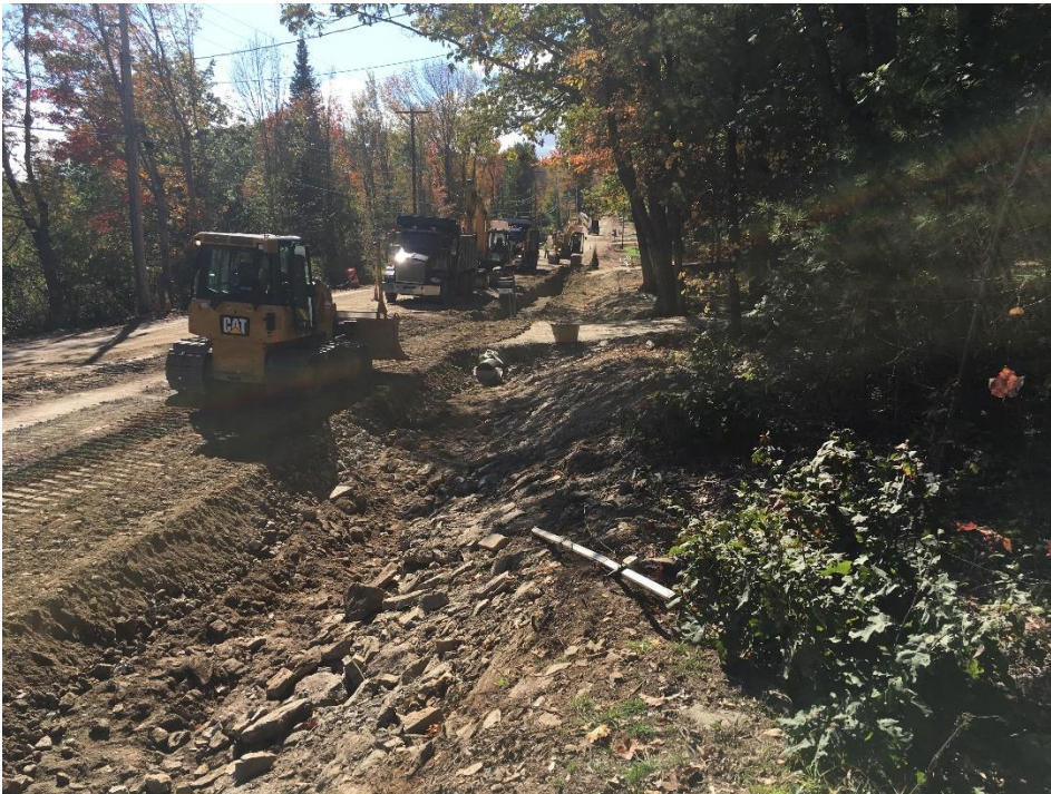
Photo 4 – View looking south depicting the underdrain installation process. The excavator in the background excavates the trench to the proper grade. A second excavator places bedding stone from the dump truck as the pipe is installed followed by stone above the pipe. Gravel from dump trucks is then dropped by the edge of the road and placed by the dozer.
