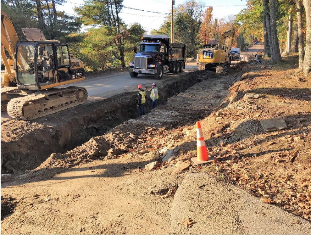
Photo 1 – Crew began the day installing 6-inch underdrain from STA 35+50 (south of #72 driveway) southward.
