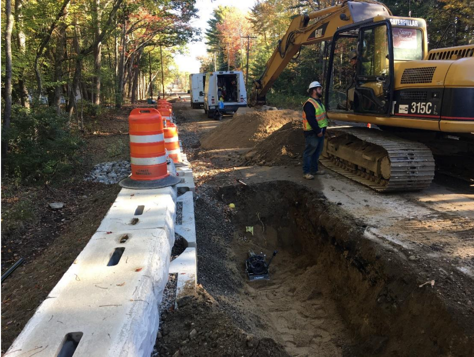
Photo 1 - At the beginning of the day, the southern end of the section of gas main placed during the installation of the retaining wall was exposed. The trench was then excavated southward and bedding sand placed prior to placing the gas main.
