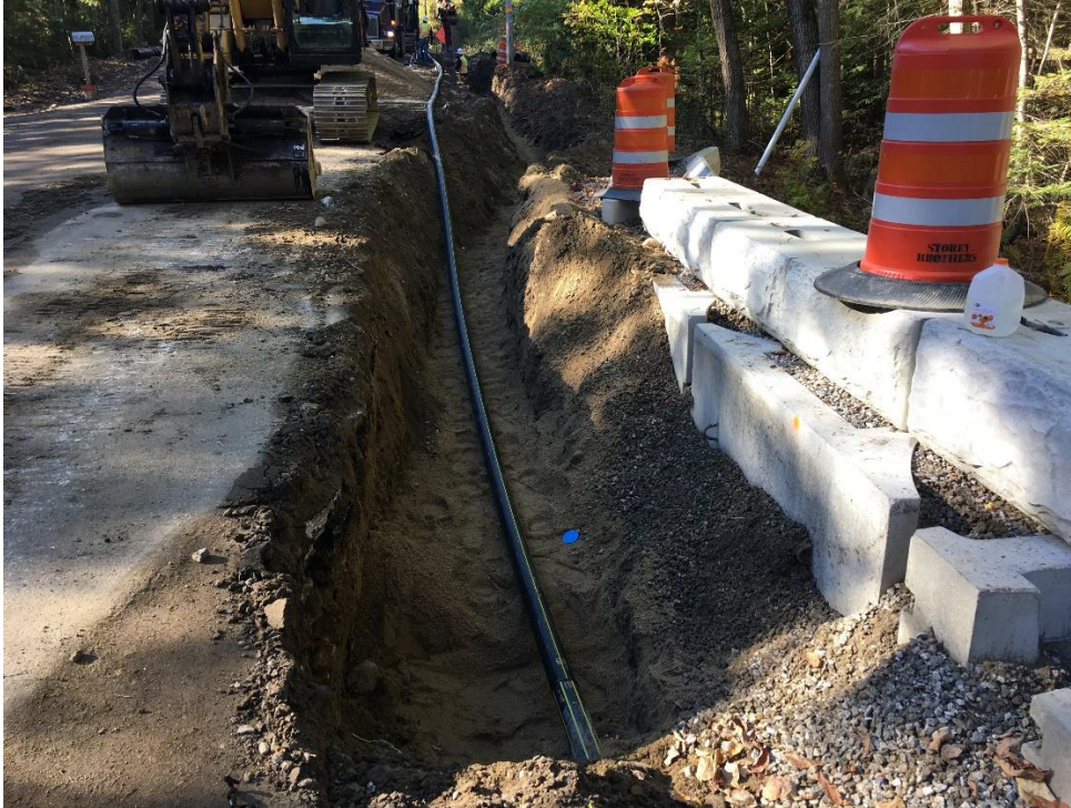
Photo 3 – Looking southward, a section of gas main has been welded onto the previously installed section shown in Photo 1 and placed over bedding sand. The rest of the gas main will be placed in the trench after bedding sand has been placed in the entire length of the trench.
