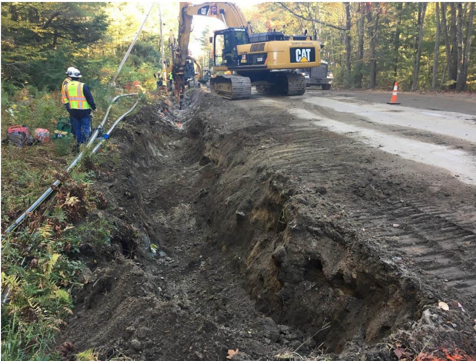
Photo 2 – A short section of ledge south of Evergreen Lane had to be removed with a hoe ram before the trench excavation could be completed to match up with the southern extend of the water main extension.
