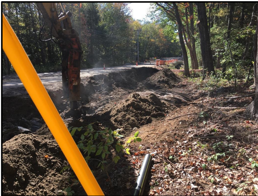
Photograph 10 – Wednesday, October 11 th – A section of ledge between 38 and 34 Middle Road that was not blasted had to be removed with the hoe ram before the crew could connect to the previously install main behind the retaining wall.
