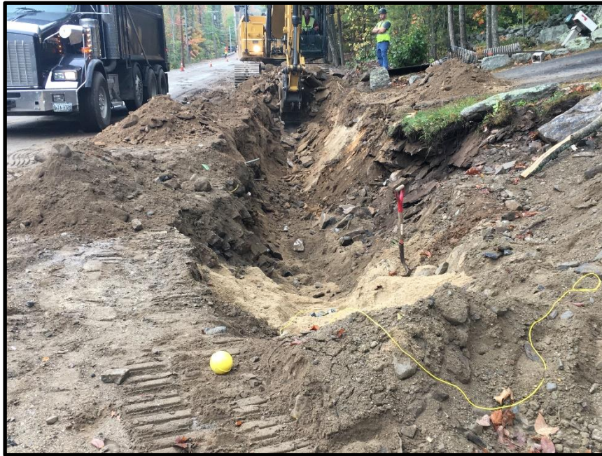
Photograph 5 – Monday, October 9 th – Initial excavation to install natural gas main in areas previously skipped due to ledge. Here in front of 70 Middle Road.
