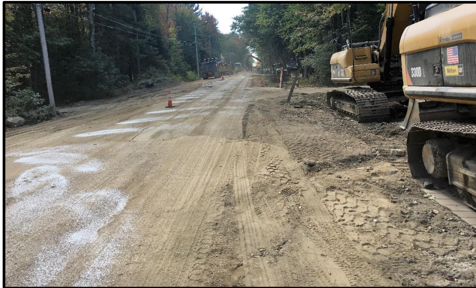
Photograph 2: Thursday, October 5 th - Overall work zone. Unloading retaining wall block to the right of the road and installing a "short side" water service at Waterfall Way on the left side of the road. In the foreground, freshly broadcasted calcium chloride for dust control on the left and idle excavators parked on right.
