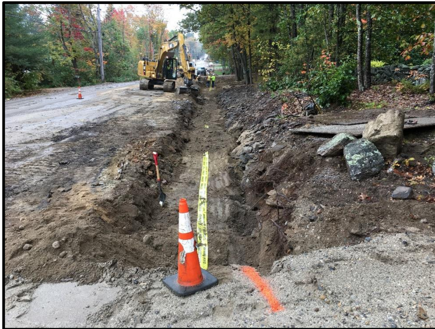
Photograph 6 - Monday, October 9 th - By mid-afternoon the crew was backfilling gas trench using 2 excavators to place sand over the gas main (in the background) followed by second excavator backfilling to grade for drainage swale with native material.
