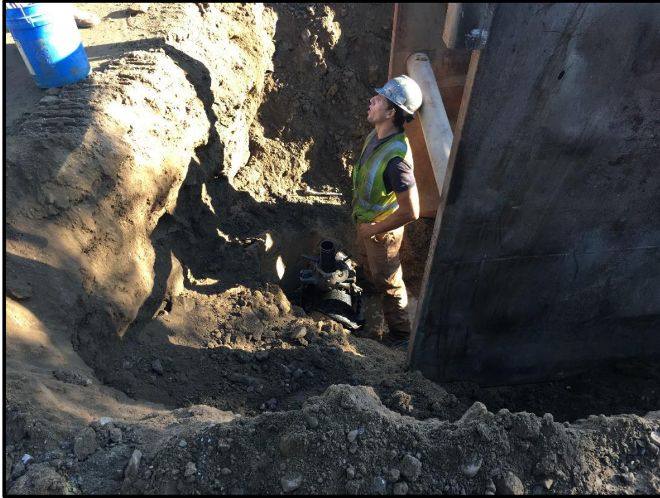
Photograph 1 – Thursday, October 5 th - Preparing to tap the 12-inch water main extension to receive the 1-inch corporation stop valve and copper water service line.
