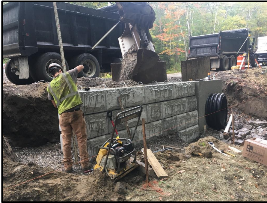
Photograph 3 - Friday, October 6 th – Placing precast blocks of the retaining wall, checking alignment and backfilling with crushed stone. Here crew is working on the northern half of the wall.
