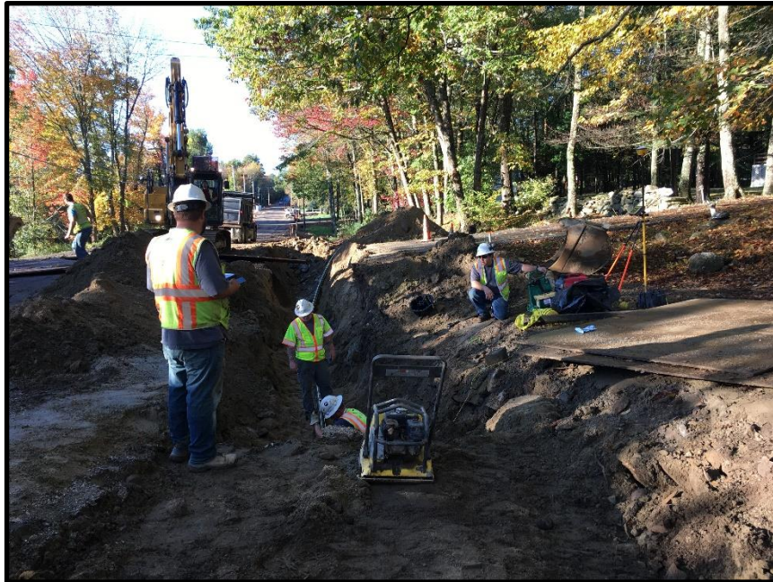
Photograph 7 – Tuesday, October 10 th - Initial excavation to complete the gap in the natural gas main installation skipped earlier due to ledge near 58 Middle Road.
