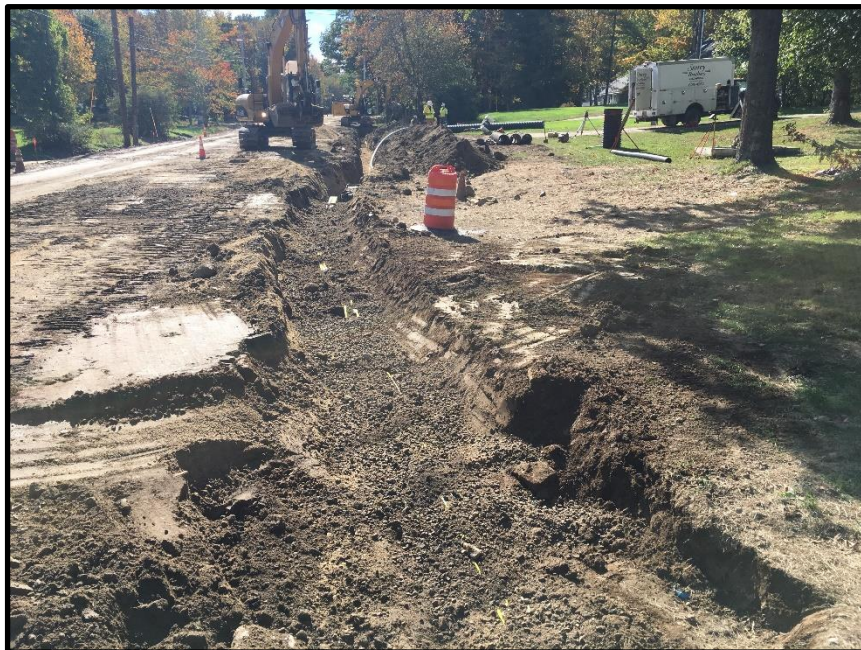
Photograph 8 - Tuesday, October 10 th – After the gap in the gas main installation was installed, the crew resumed where the installation has previously stopped at STA 24+40 (just south of Range Way). The jog in the alignment of the gas main trench is due to the retention of the 12-inch underdrain in front of 54 Middle Road.
