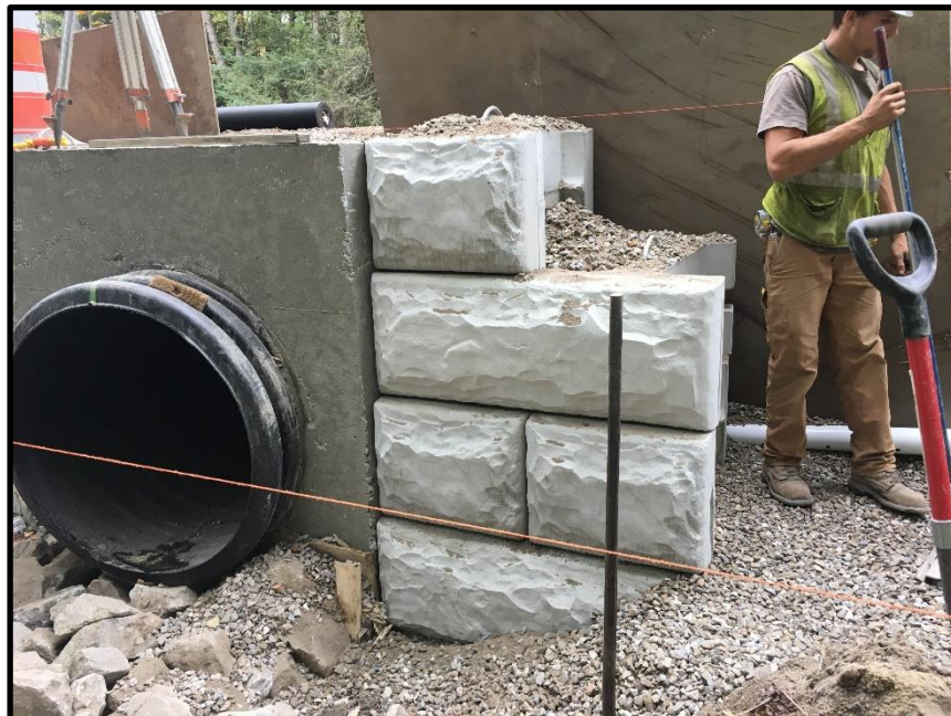
Photograph 4 - Friday, October 6 th – Starting the southern half of the wall and preparing the base for the next block. PVC underdrain for the wall shown behind worker.
