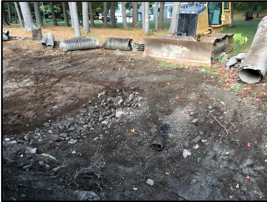
Photograph 9 – Wednesday, October 11 th – Undocumented underdrain exposed in front of 44 Middle Road discharging to swale.
