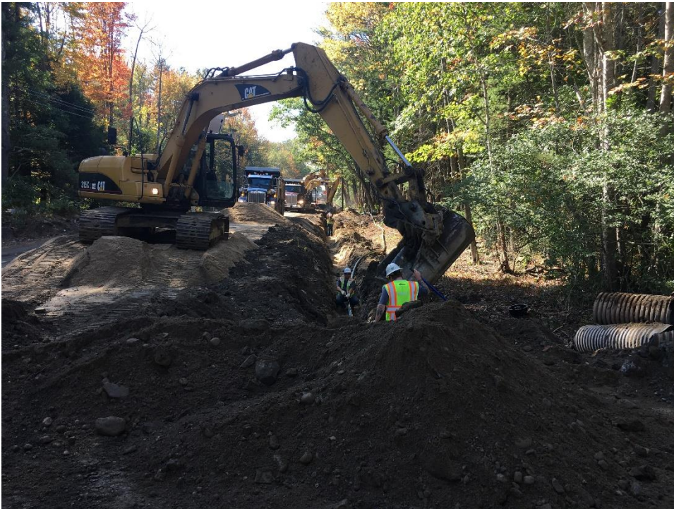
View showing three (3) excavators. One in the background hammering ledge ahead of the second in the middle excavating the trench to proper subgrade, followed by the third in the foreground placing the bedding sand for the pipe.
