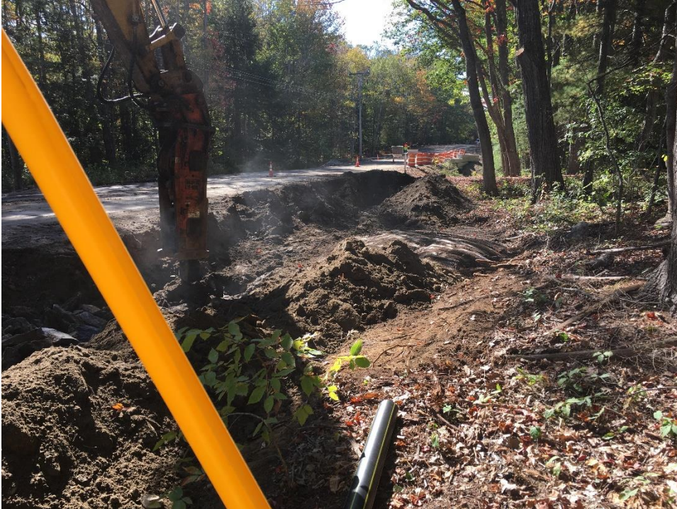
A section of ledge between 38 and 34 Middle Road that was not blasted had to be removed with the hoe ram before the crew could connect to the previously installed main behind the retaining wall.
