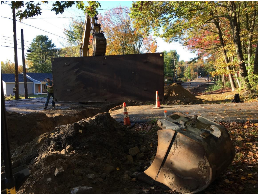
To maintain access to the driveway two steel plates were placed over the gas main trench.
