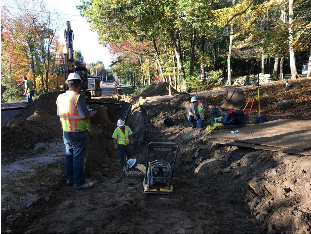
Initial excavation to complete the 160-foot gap in the natural gas main installation skipped earlier due to ledge near 58 Middle Road.
