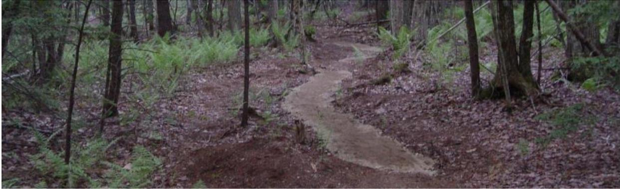
*Example of stabilizing sand/gravel path used to harden soft area that had become mucky due to wet conditions and heavy use. The goal is to keep the width of the trail from expanding and allow the vegetation along the alternate path (to the left of the original path) to grow back to its natural state.*
