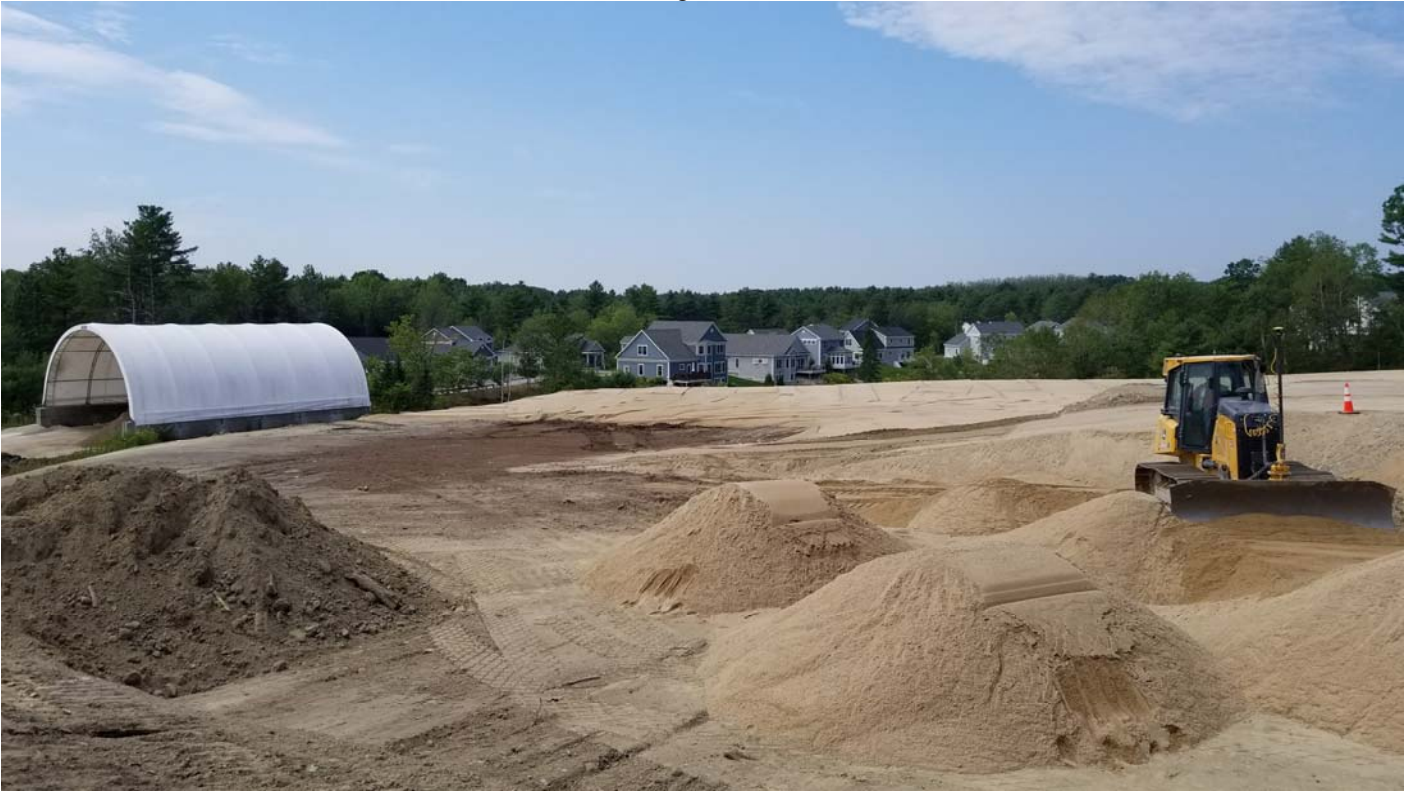
Placing the gas vent sand over the northeast corner of the landfill.
