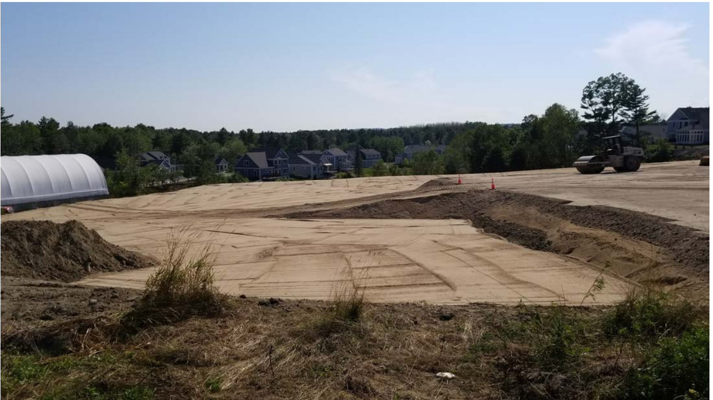
Gas vent sand finished over the graded areas.
