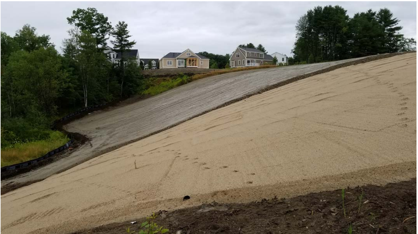
Placed and compacted eighteen inches of barrier soil over the southwest corner of the landfill. Photo taken Tuesday morning after the rain.
