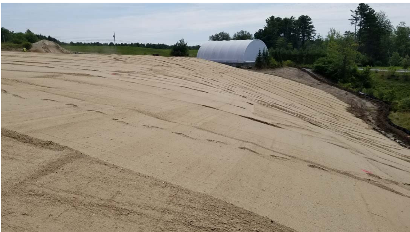
Six inches of gas vent sand across the southern slopes of the landfill.
