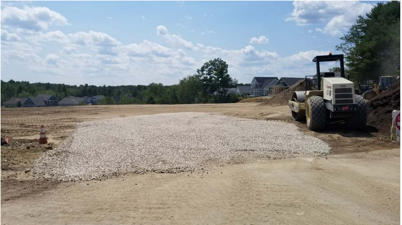
Stabilized construction entrance placed once the gravel pad was complete. Contractor plans to begin placing gas vent sand over the remainder of the landfill on Wednesday.
