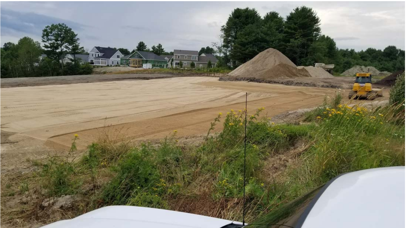
Six inches of gas vent sand placed over the subgrade under the compost pad area.
