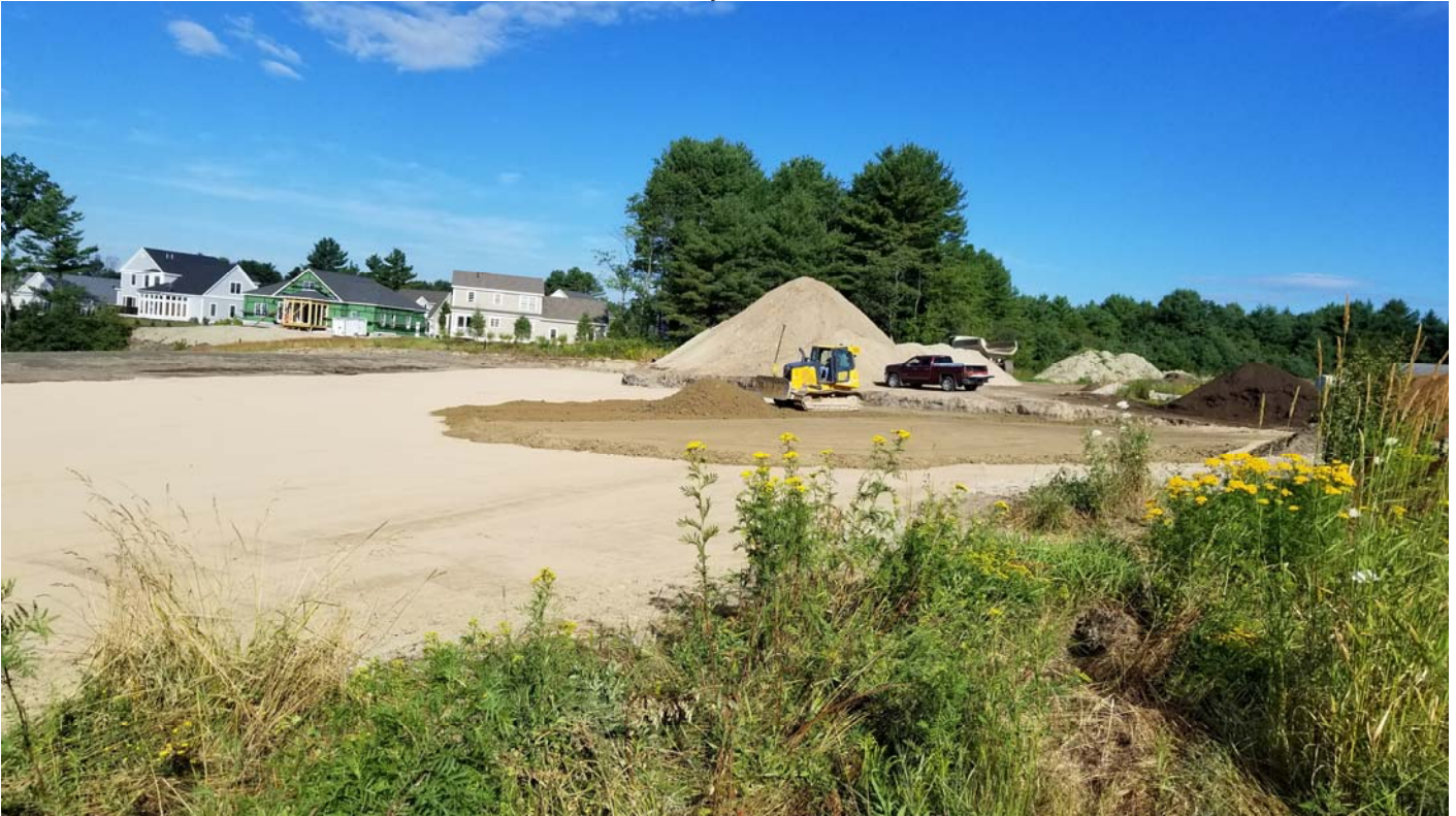
Barrier soil was placed in a twelve-inch lift starting at the entrance ramp compost pad area.
