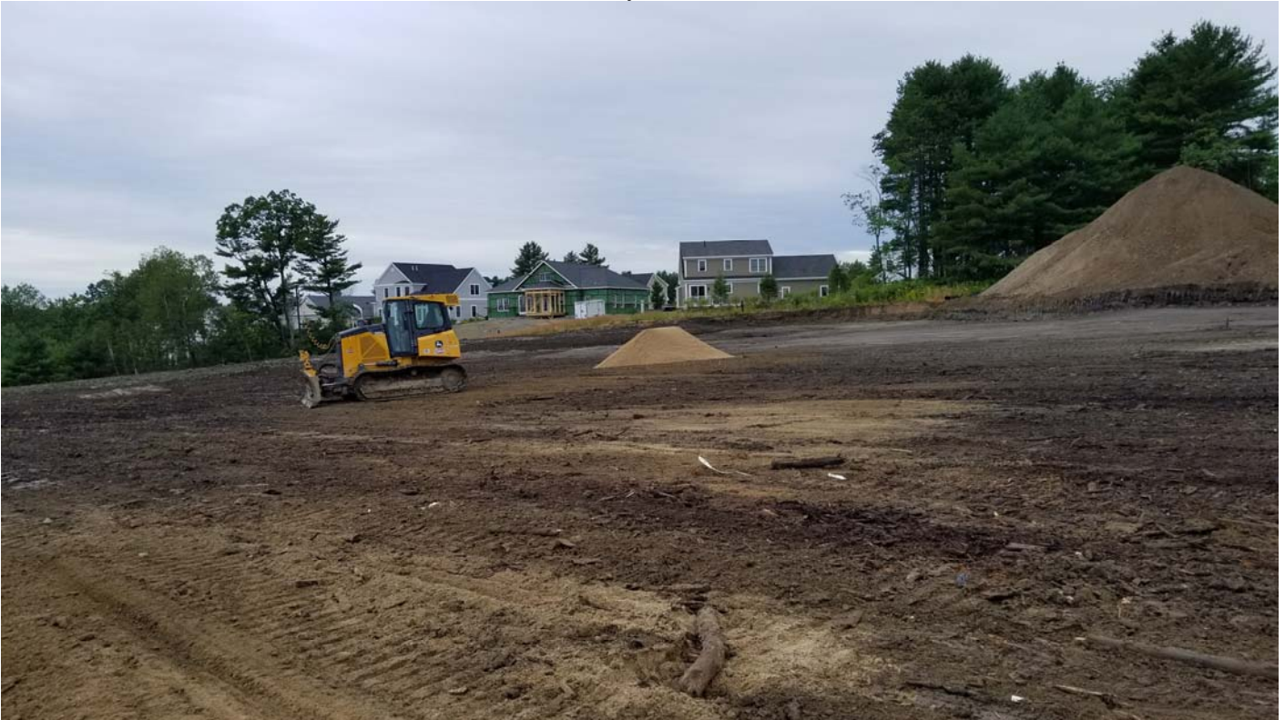
The first load of gas vent sand delivered to the compost pad area. All subgrade has been rolled.
