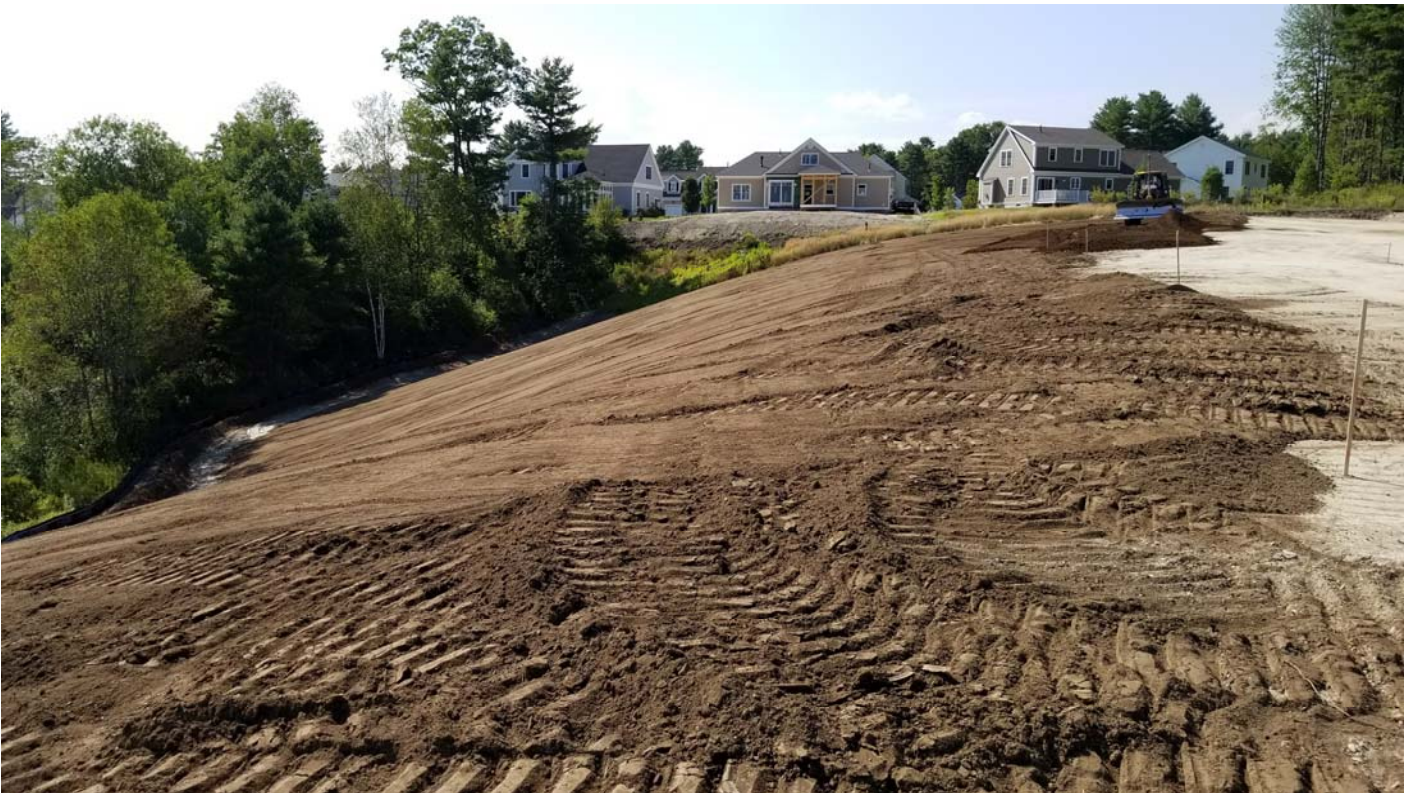
Placing vegetative soil.
