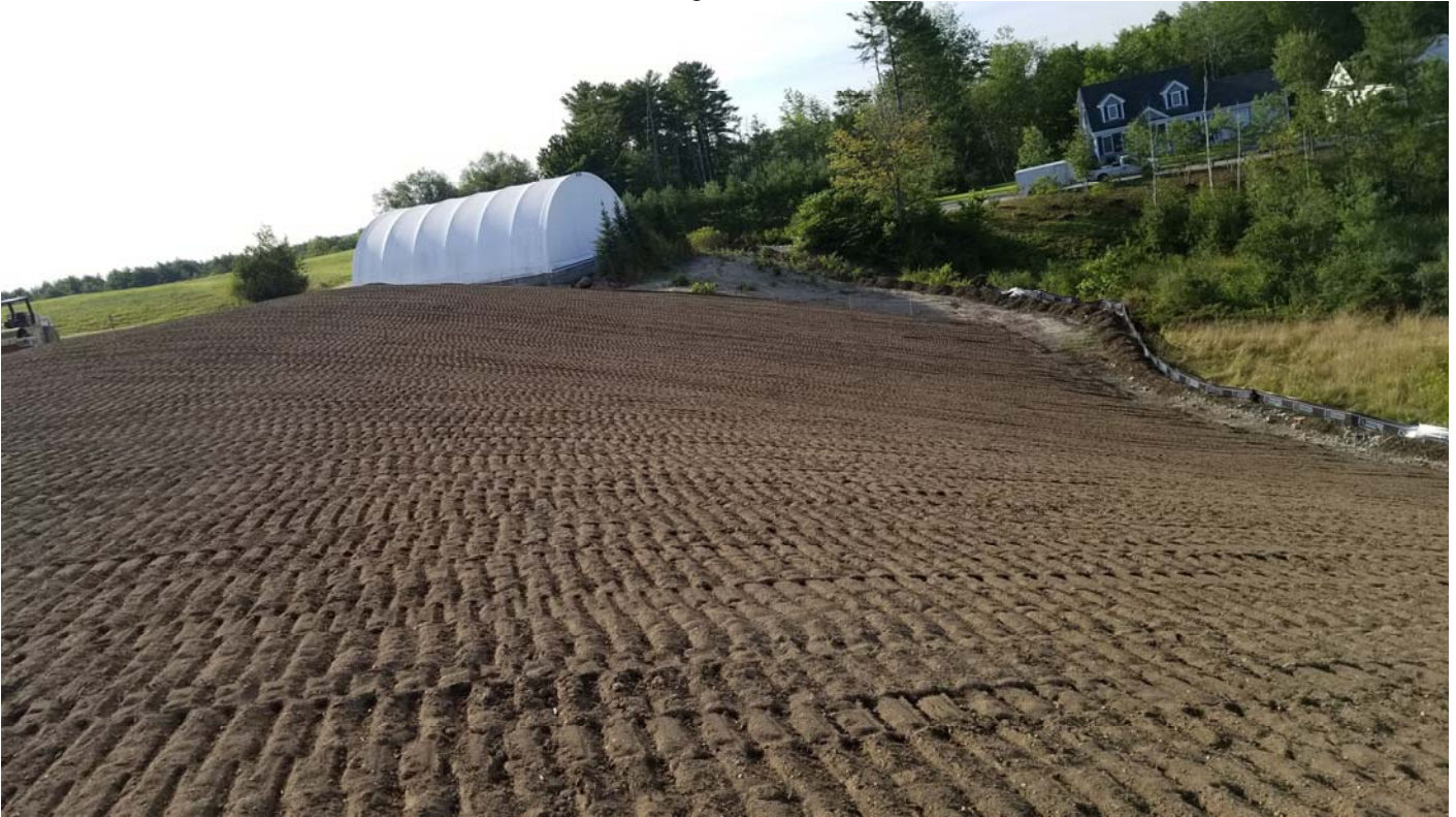
Placed and tracked topsoil over southern slope.
