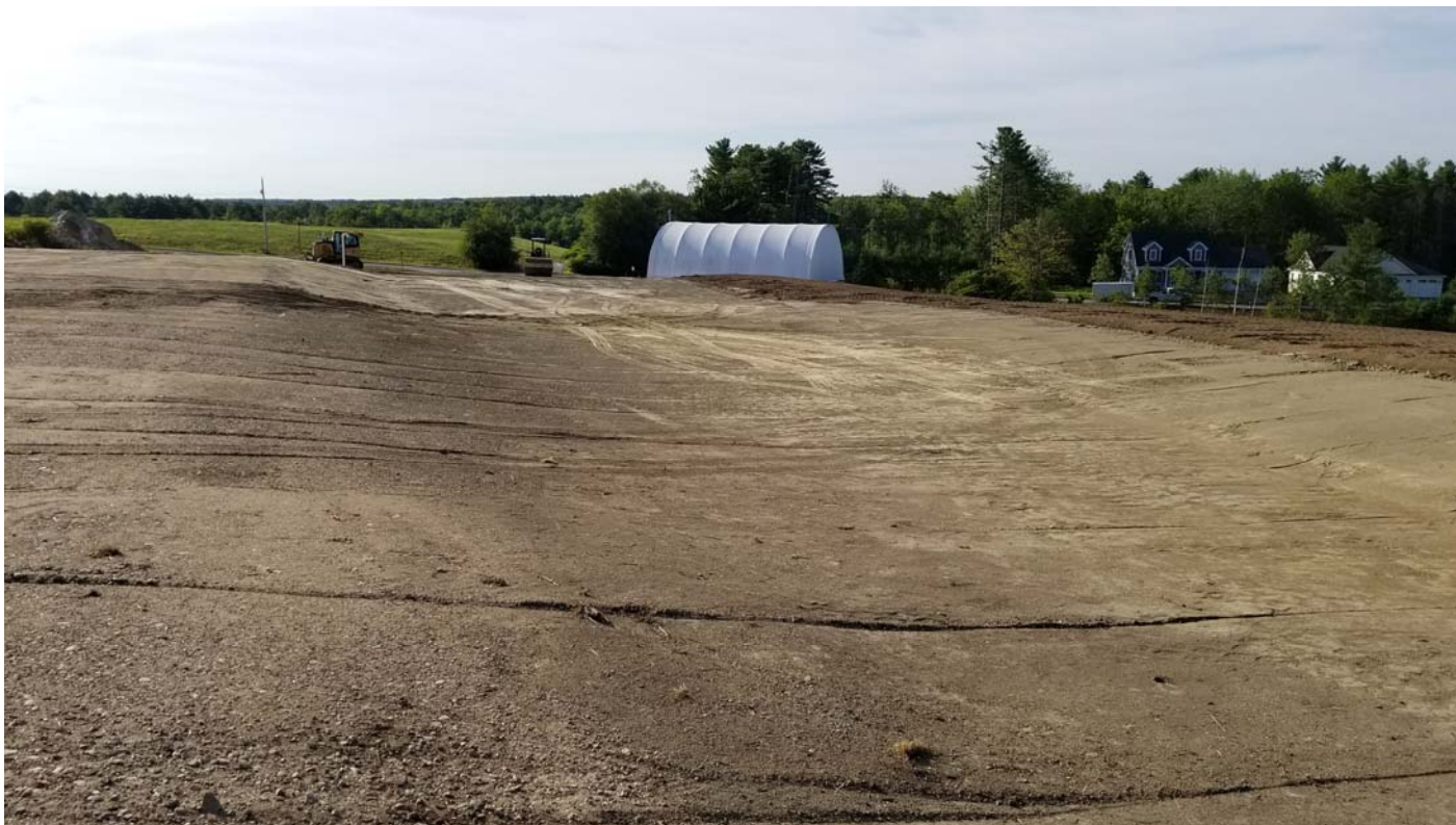
Placed gas vent sand, barrier soil, and then common borrow in the gas vent pipe area.
