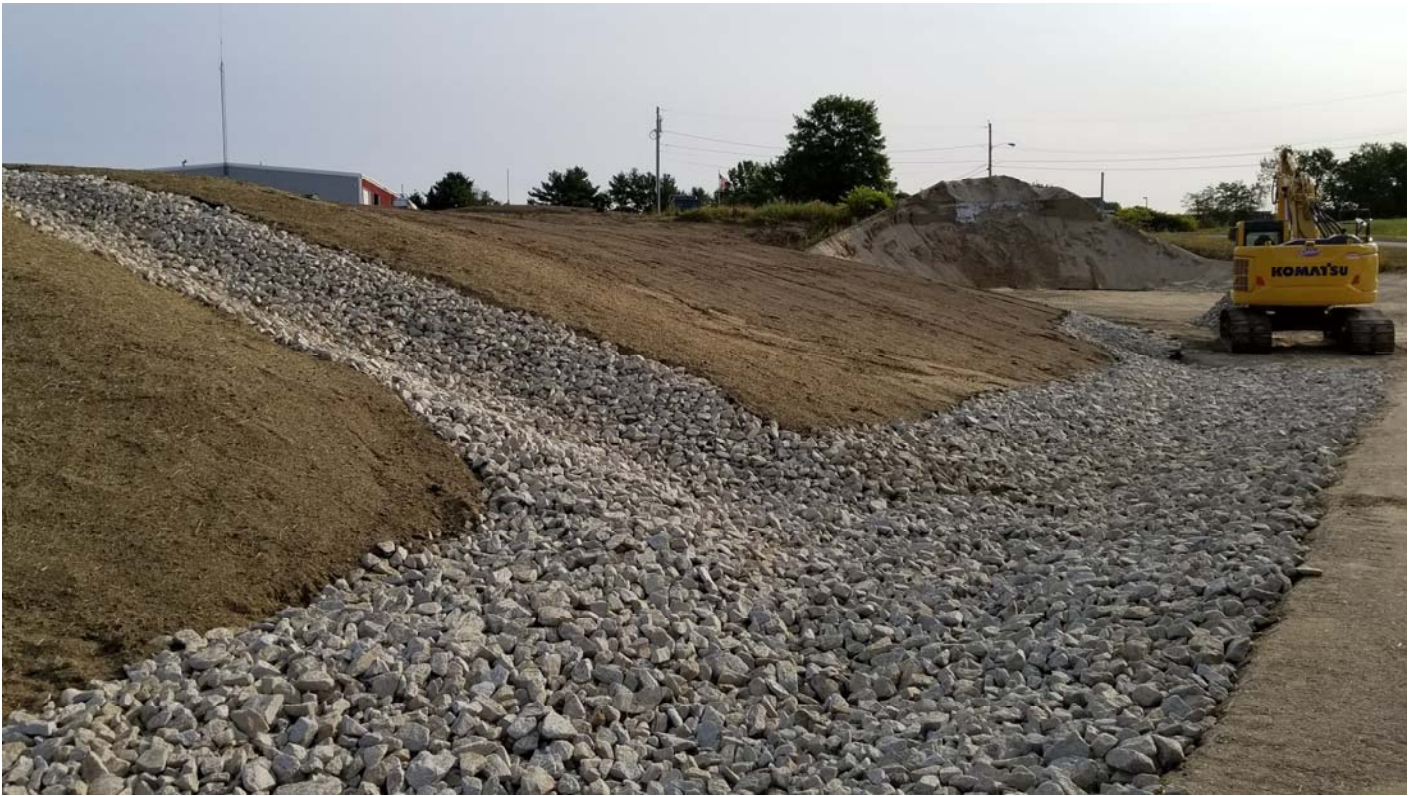
Finished the ditches, downspout, and toe along the eastern edge of the landfill.
