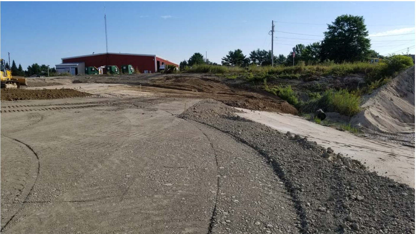
Barrier soil on the northeastern slope of the landfill.
