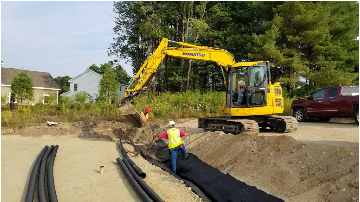
Gas pipe install along the edge of the compost pad.
