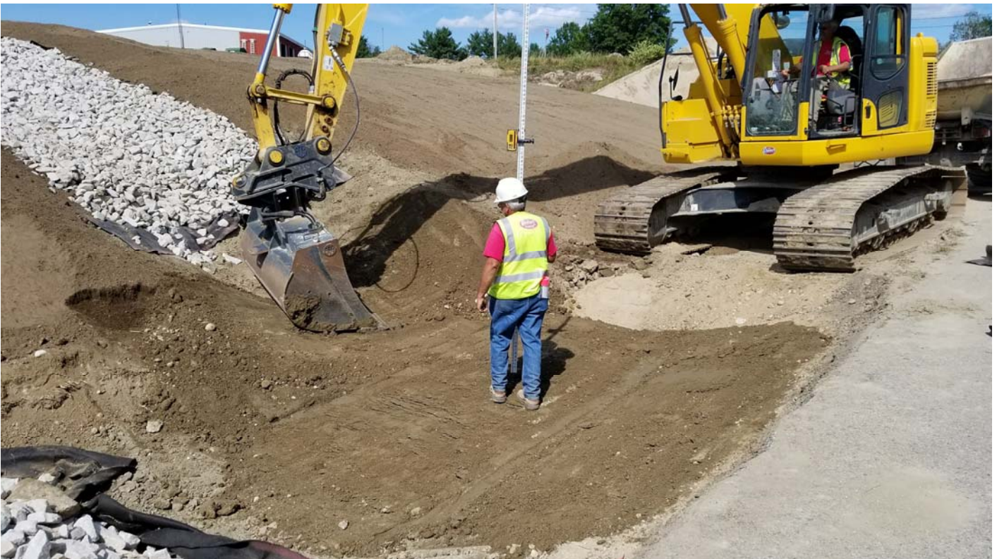
Installing the downspout and ditch along the side of the Salt Shed.
