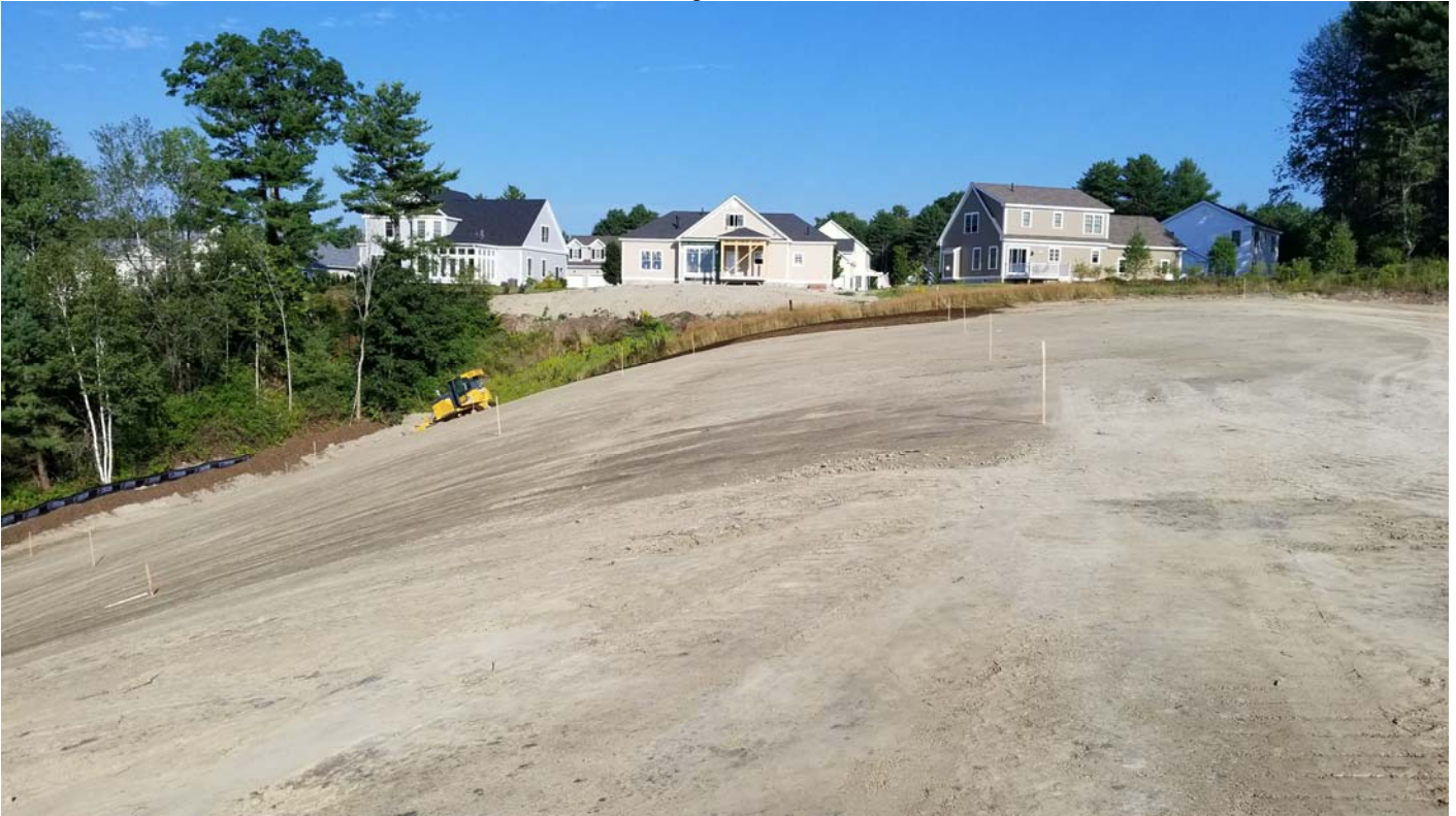
Contractor placing topsoil on the western slope. Staked out the entire slope.
