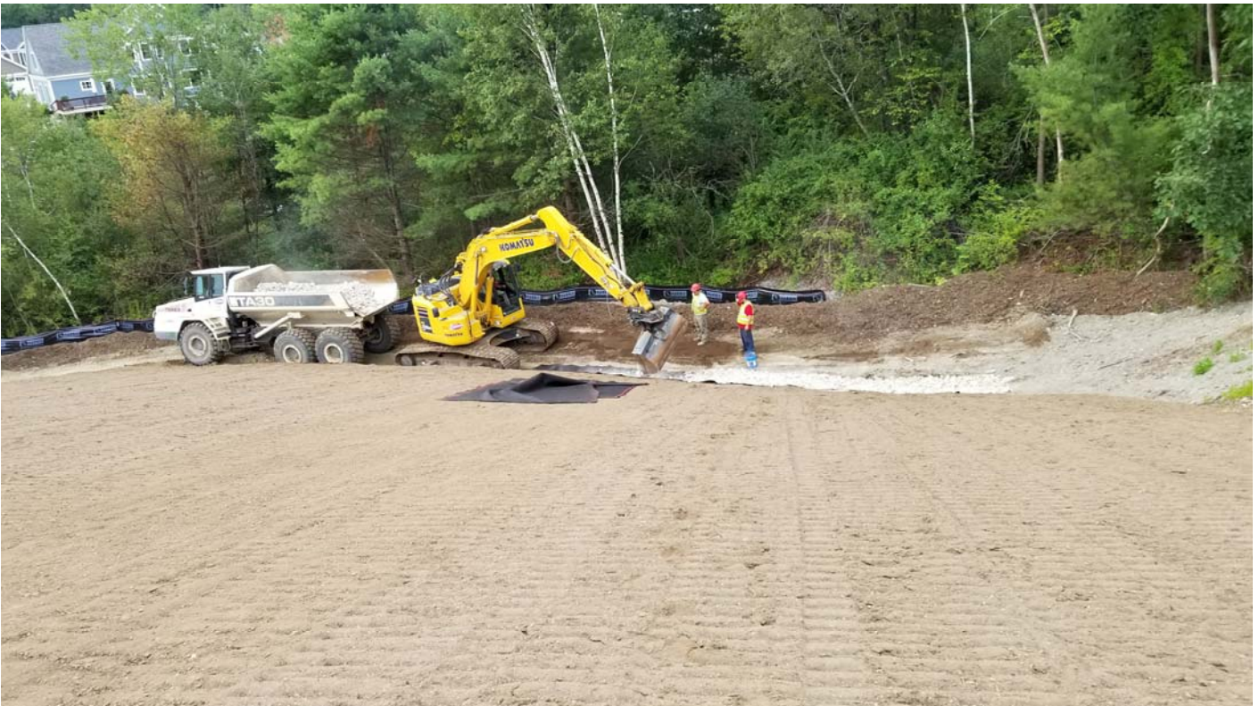
Placing riprap along the southern toe.
