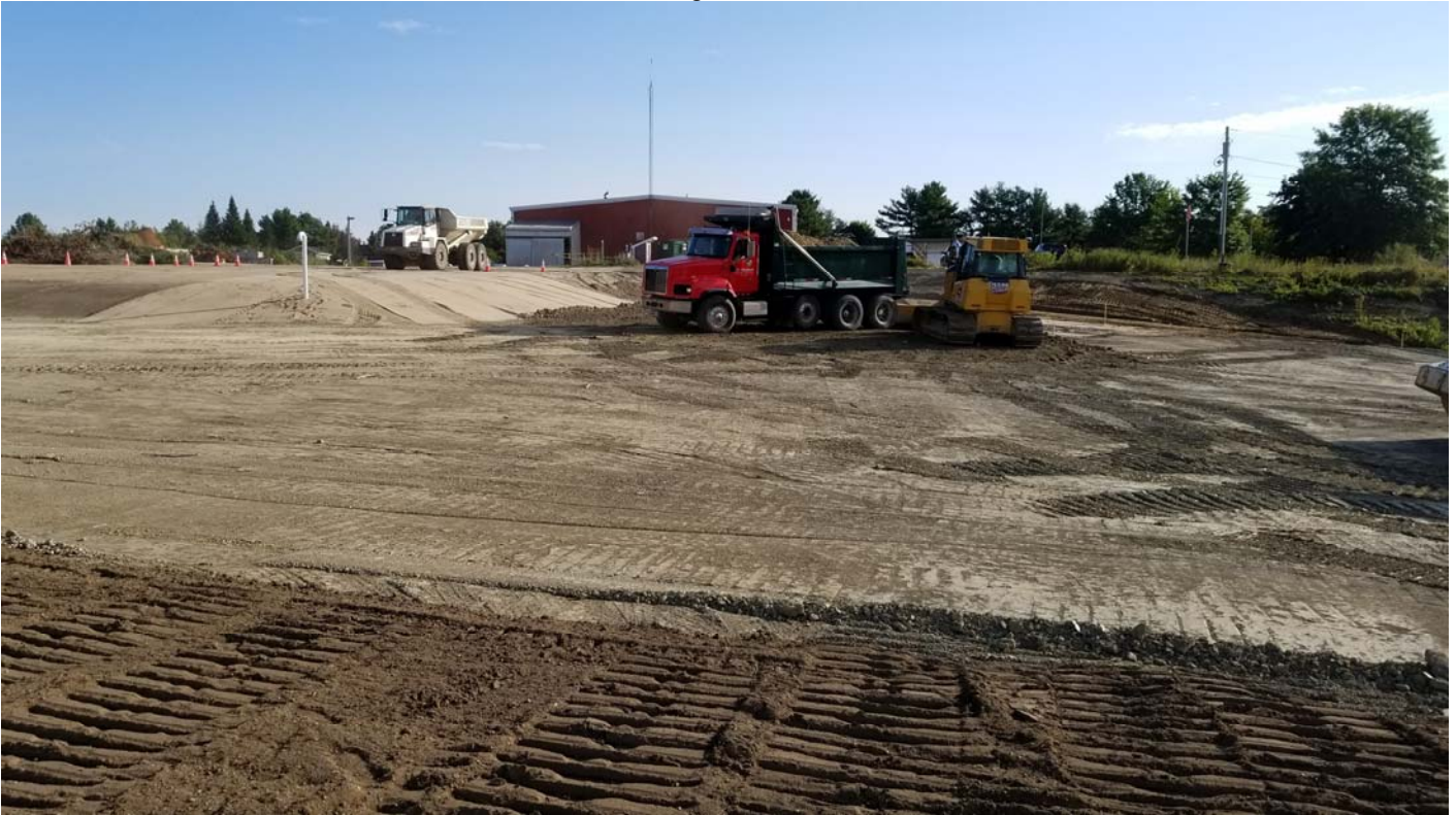
Placing barrier soil in north eastern corner of landfill.
