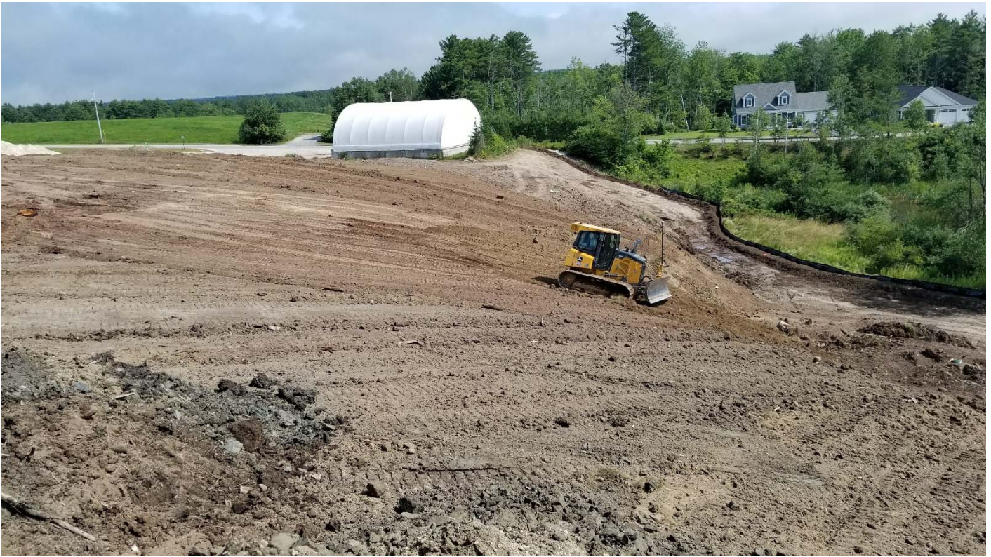
Fill was trucked in from below compost pad and placed at edge of slope and pushed into place by dozer equiped with GPS.
