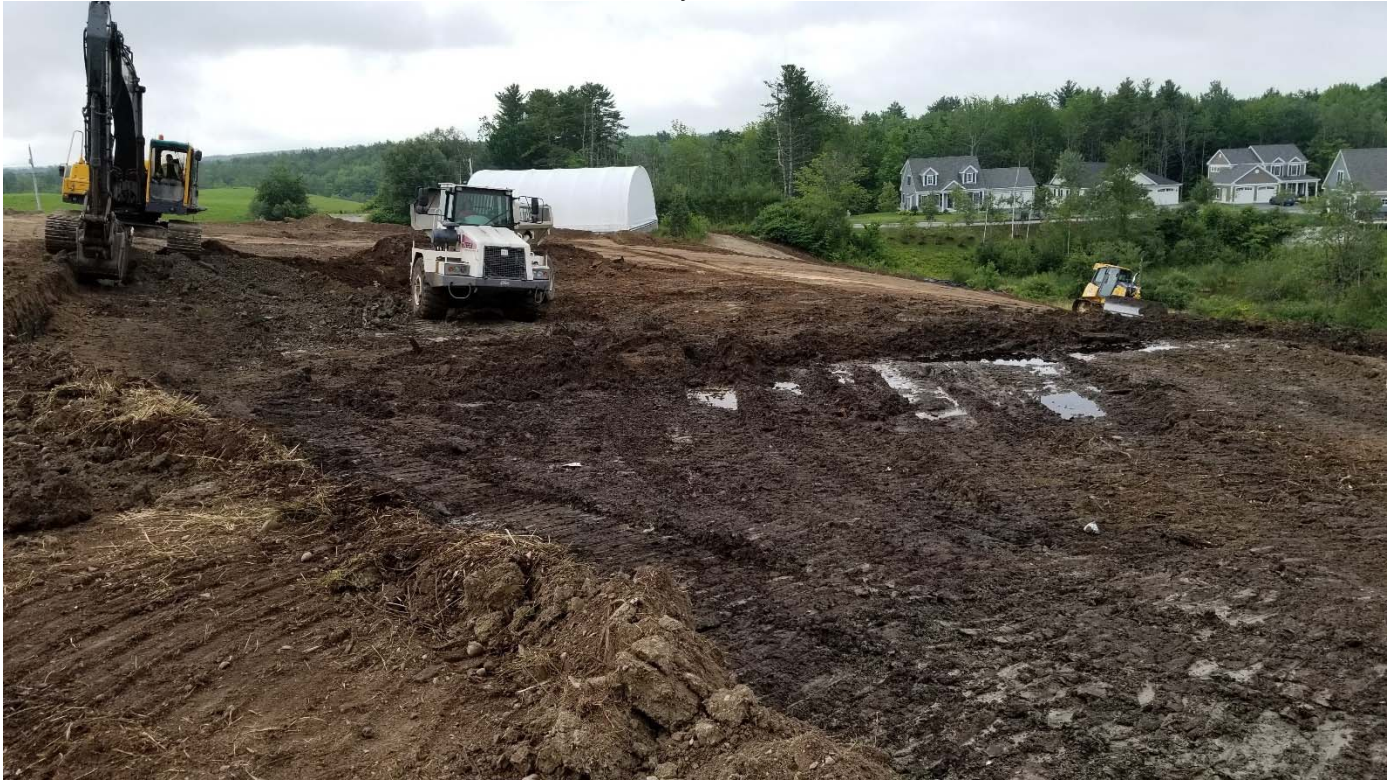
Fill excavated from below compost pad, placed at edge of slope, and pushed into place by dozer equipped with GPS. Wet area in the foreground.
