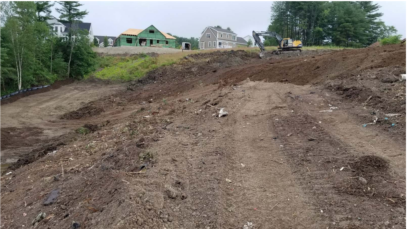
Brush and waste had been placed in lifts and is being covered.
