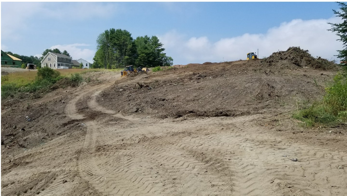
Clearing and grubbing inside clearing limits.
