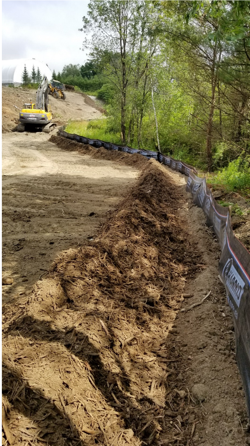
Placing silt fence and bark mulch berm for erosion control.
