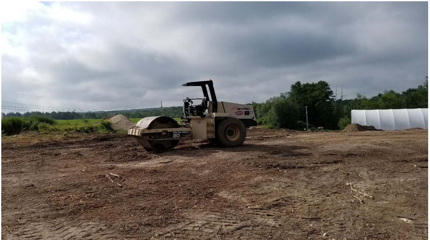
The subgrade was compacted using a smooth barrel roller.
