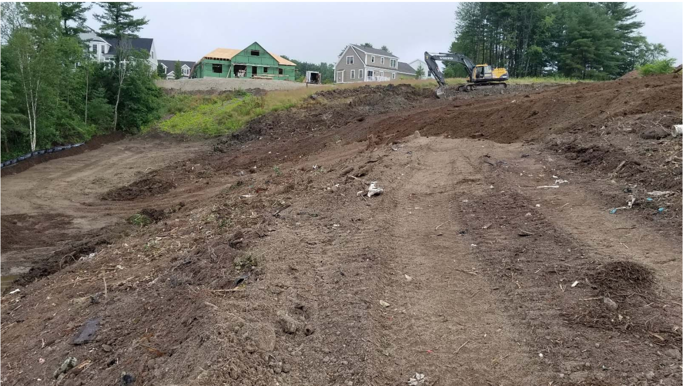
Brush and waste had been placed in lifts and is being covered.
