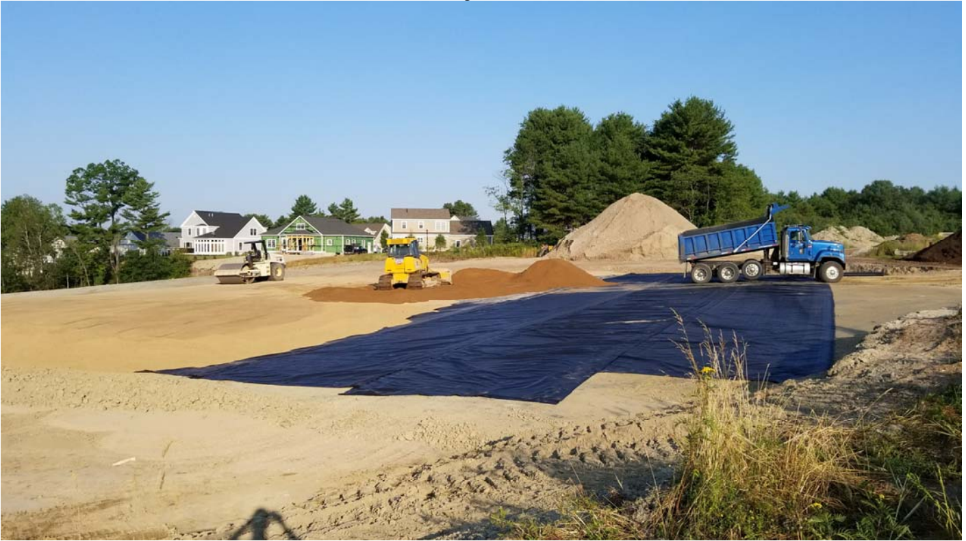
Placing the last lift section of common borrow over the northeast corner of the compost pad area.
