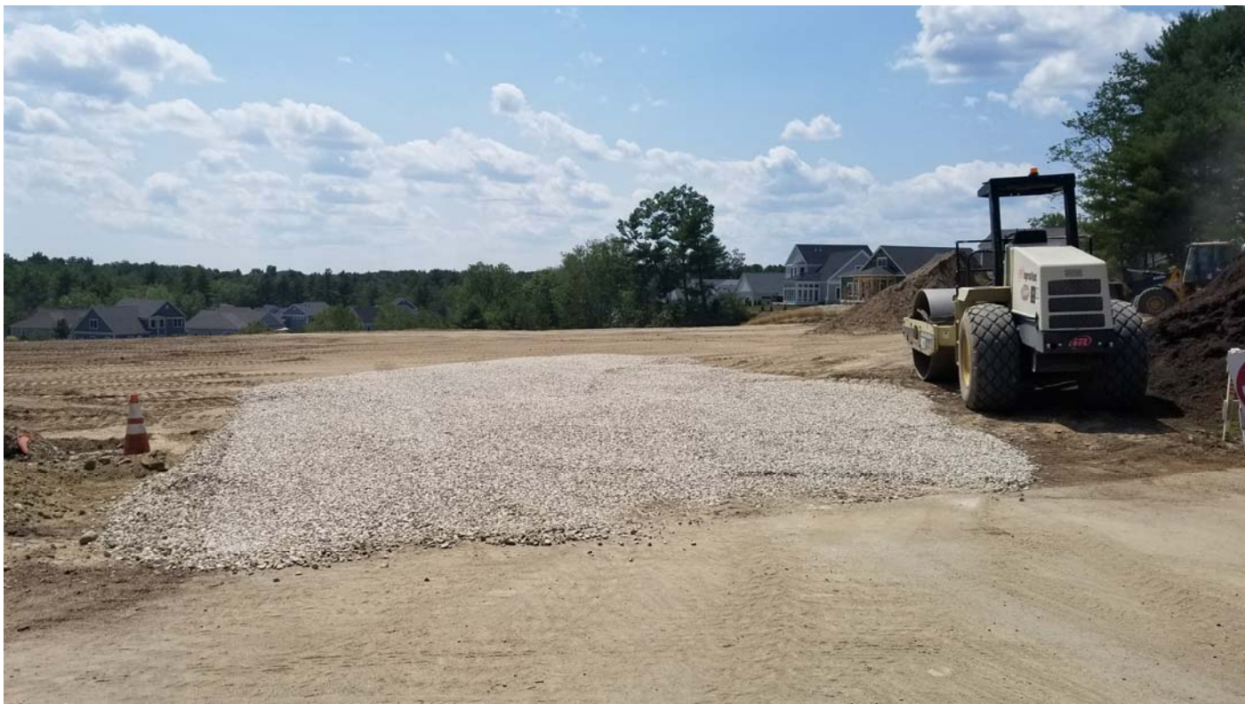
Stabilized construction entrance placed once the gravel pad was complete. Contractor plans to begin placing gas vent sand over the remainder of the landfill on Wednesday.
