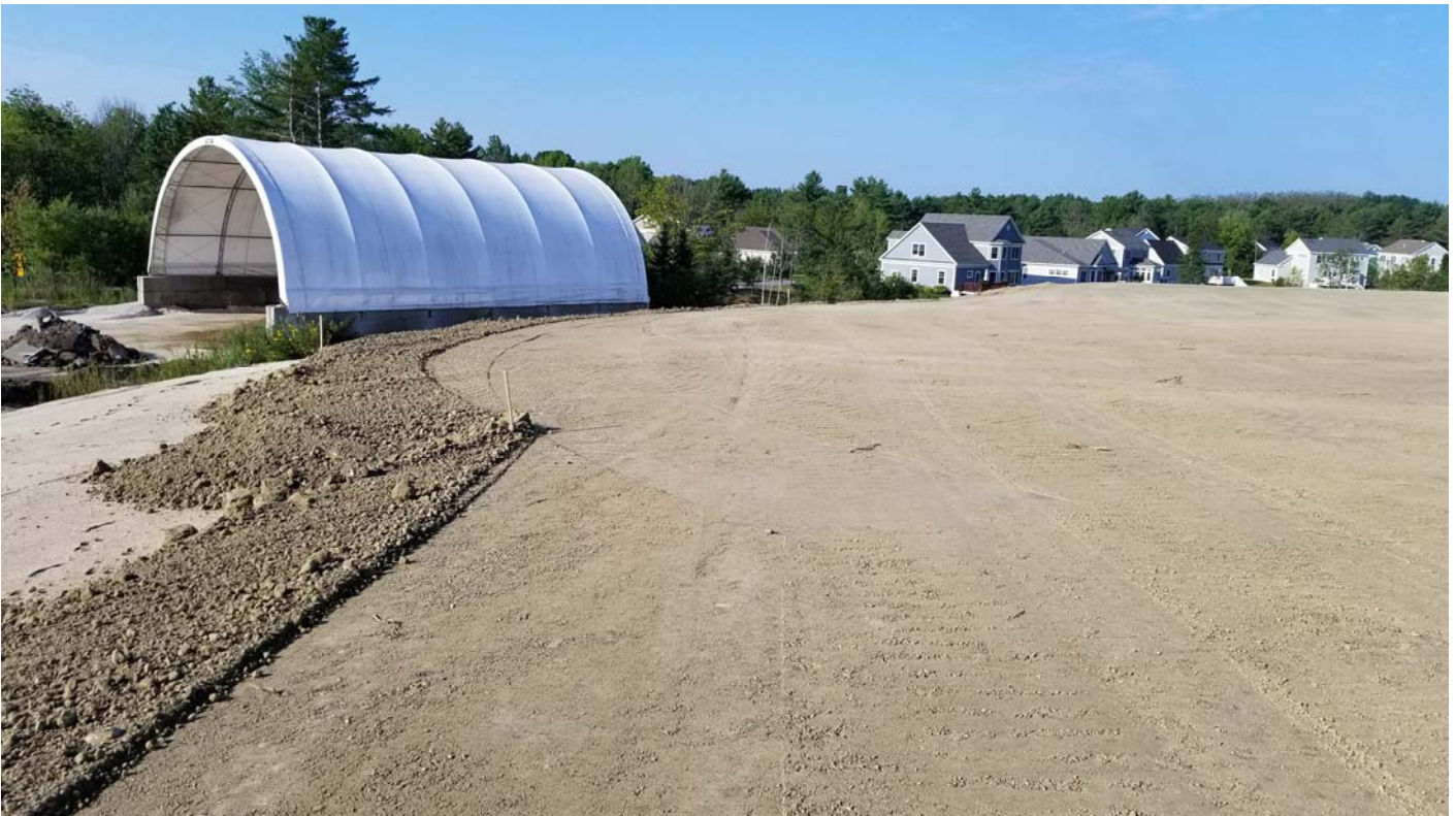
Finished placing and compacting eighteen inches of barrier soil, except for the eastern slope and gas vent pipe trench.
