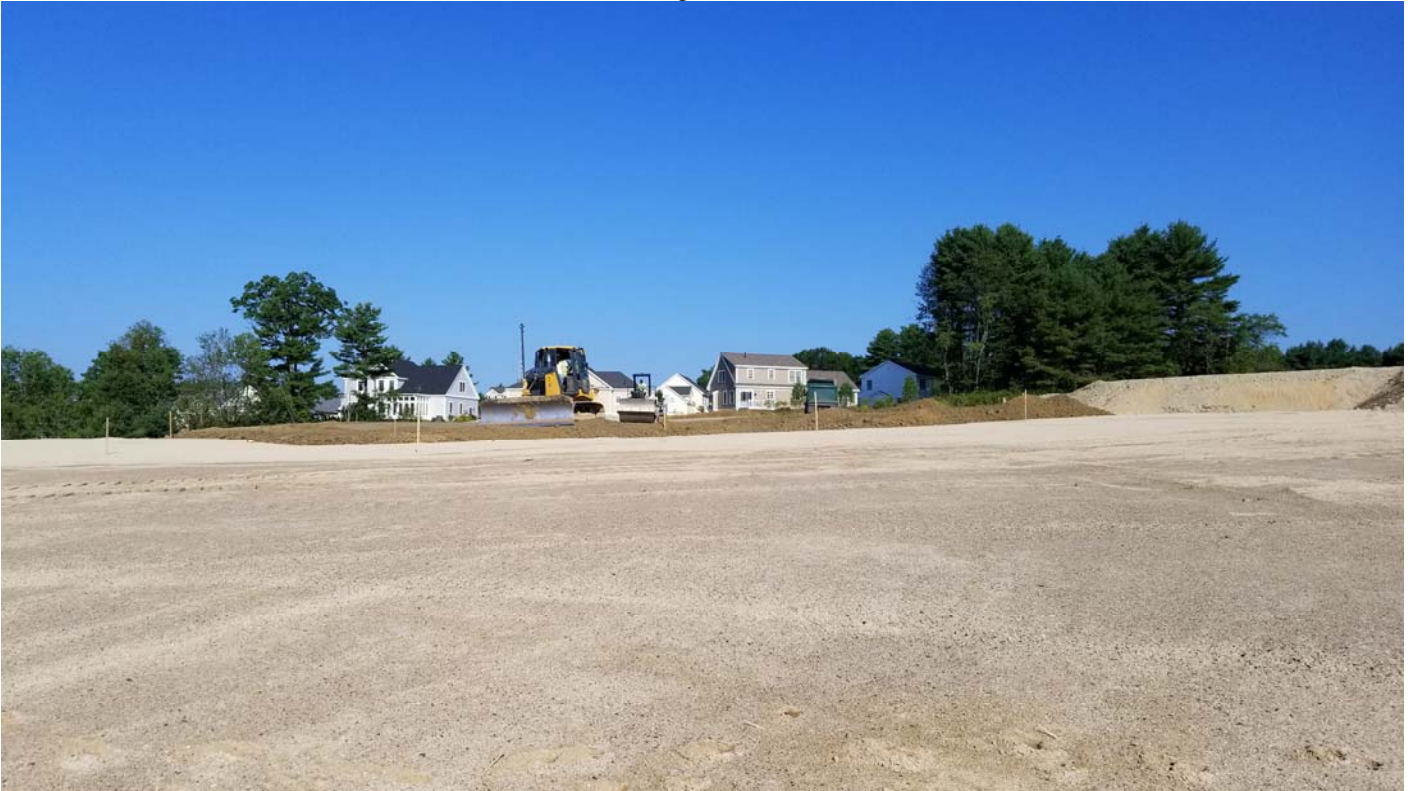
Placing the barrier soil over the northern portion of the landfill just south of the compost pad.
