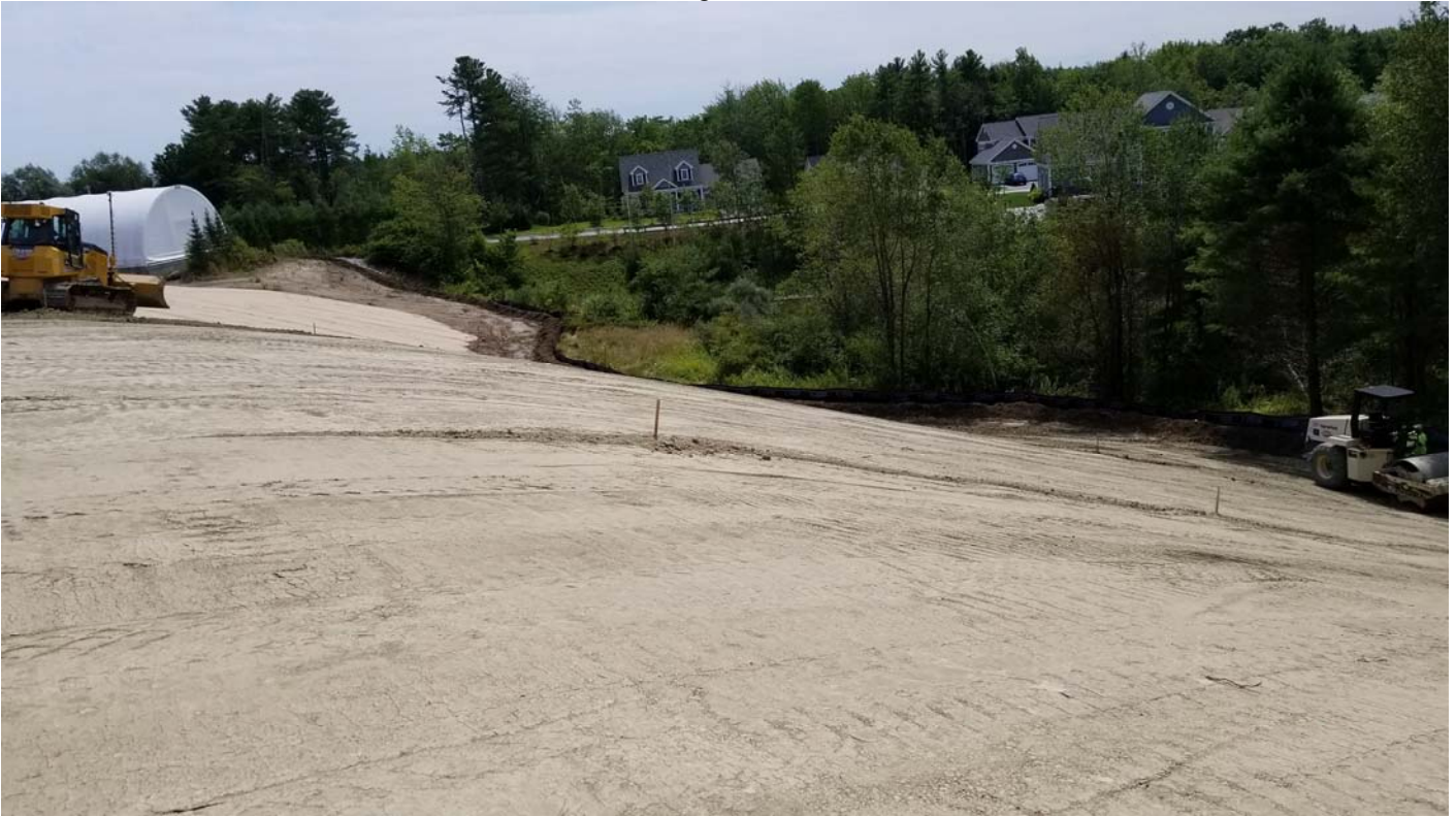
Placing the barrier soil over the southwest slope of the landfill.
