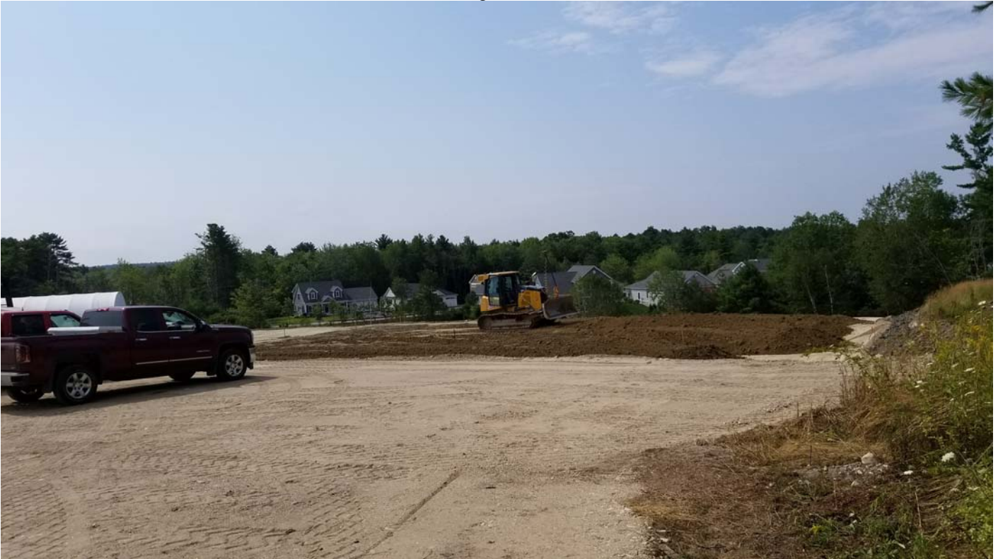
Placing the barrier soil over the northeast coner of the landfill.
