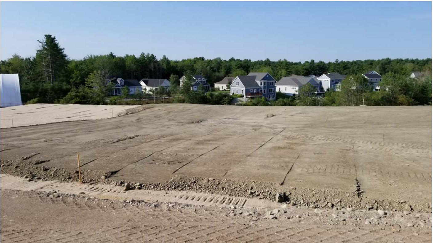
Placed and compacted eighteen inches of barrier soil over the northeast corner of the landfill.
