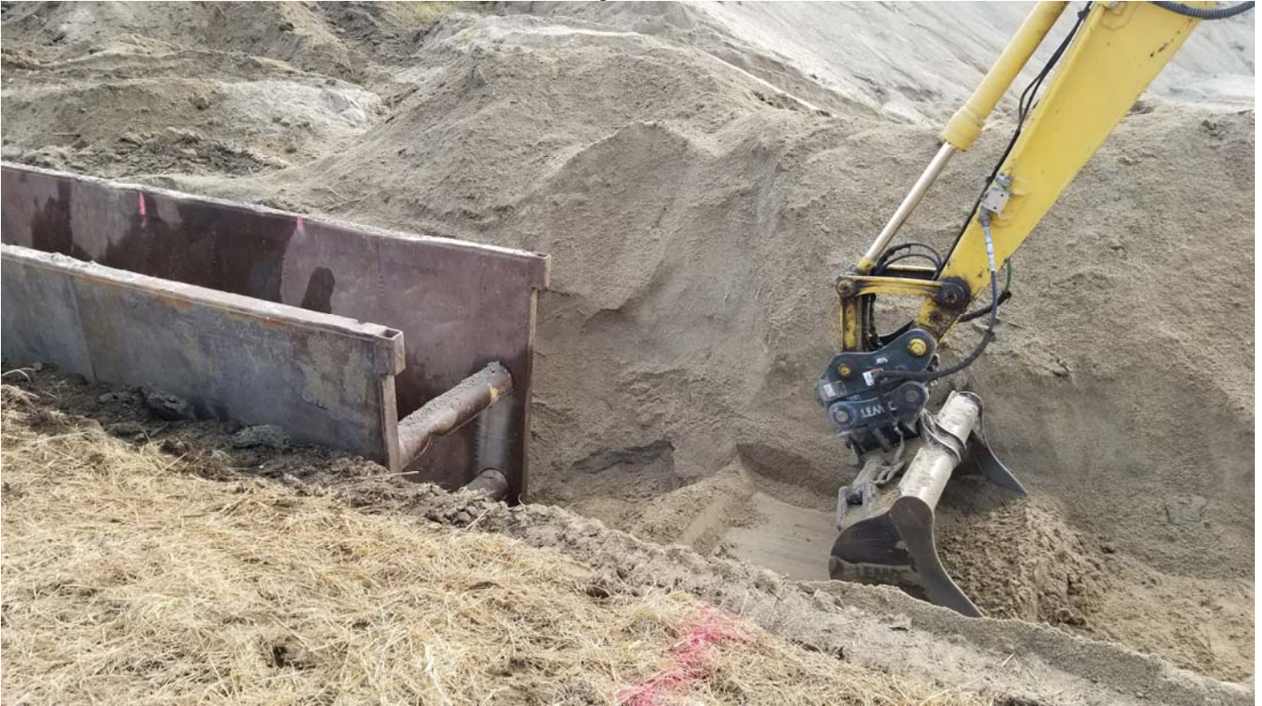
Backfilling behind the trench box.
