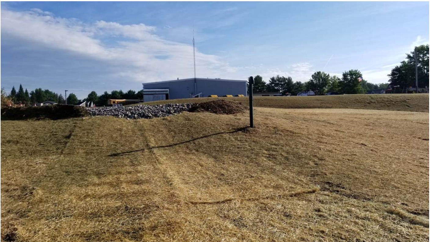
Stone check dam at the corner of the compost pad.
