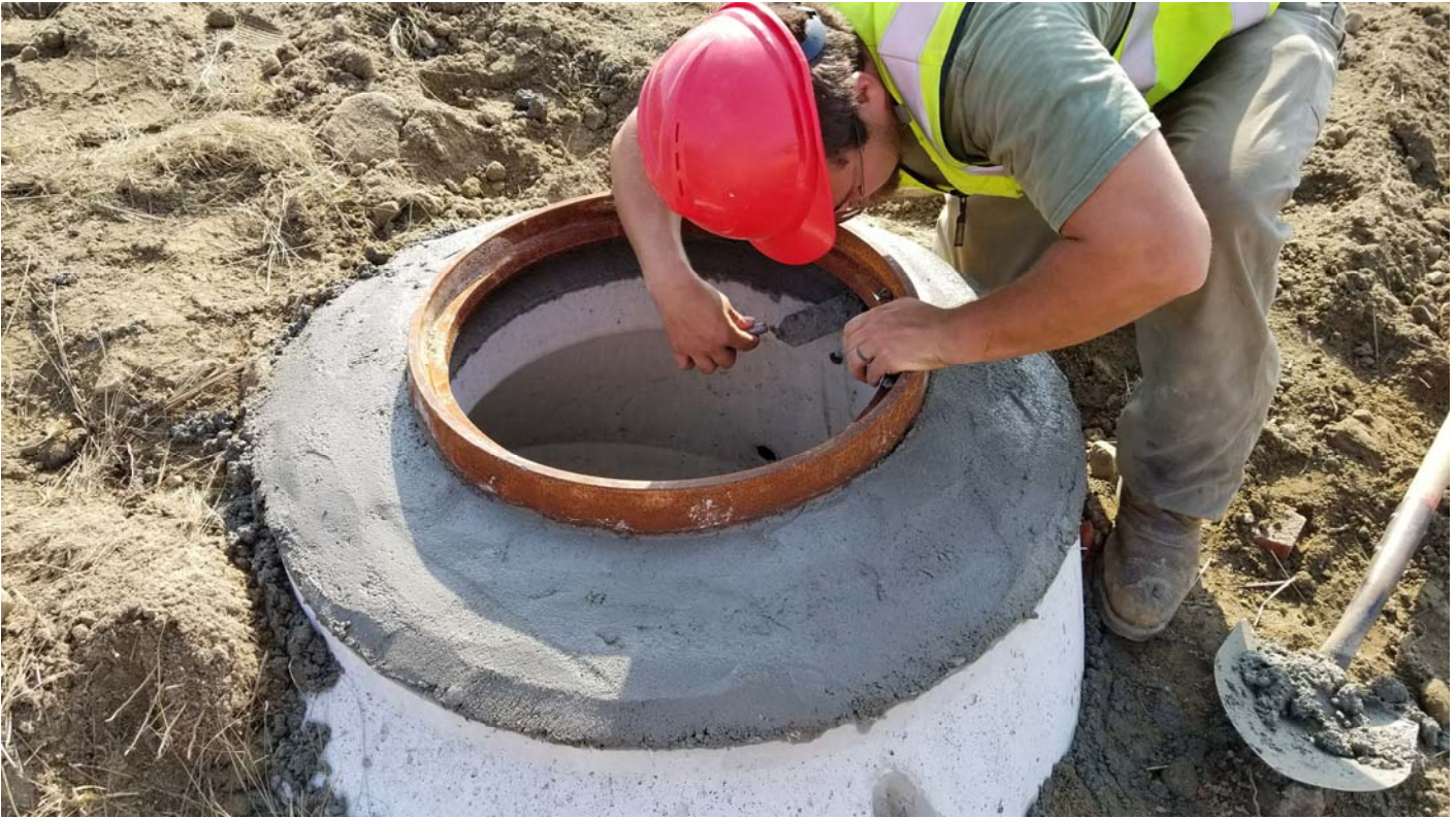
Attaching manholes covers.
