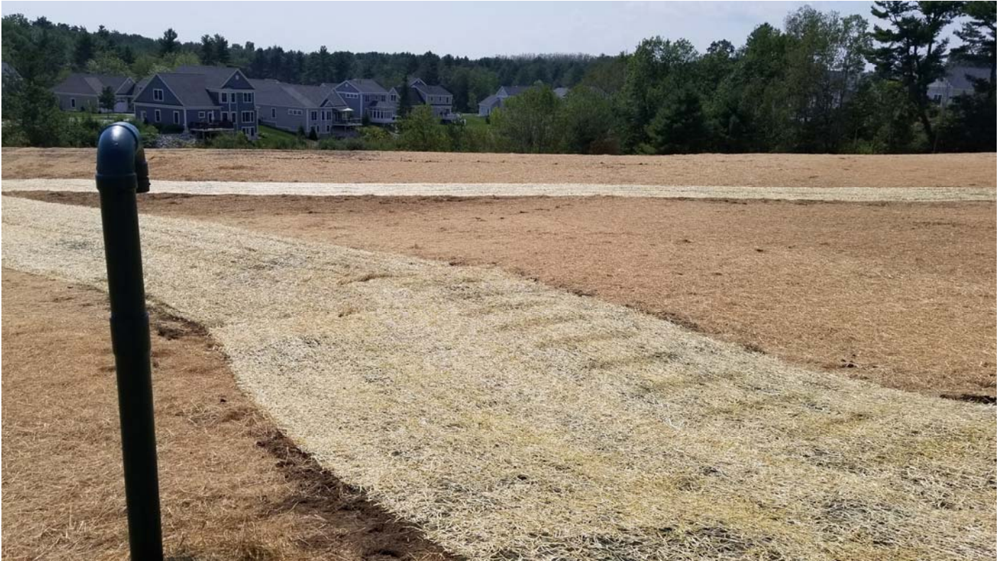
Erosion control mesh placed along drainage berm and from the compost pad.
