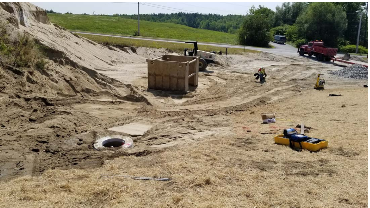
Stormdrain installed and backfilled along eastern edge of landfill.
