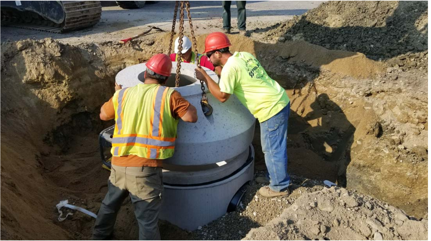
Placing the final manhole section.
