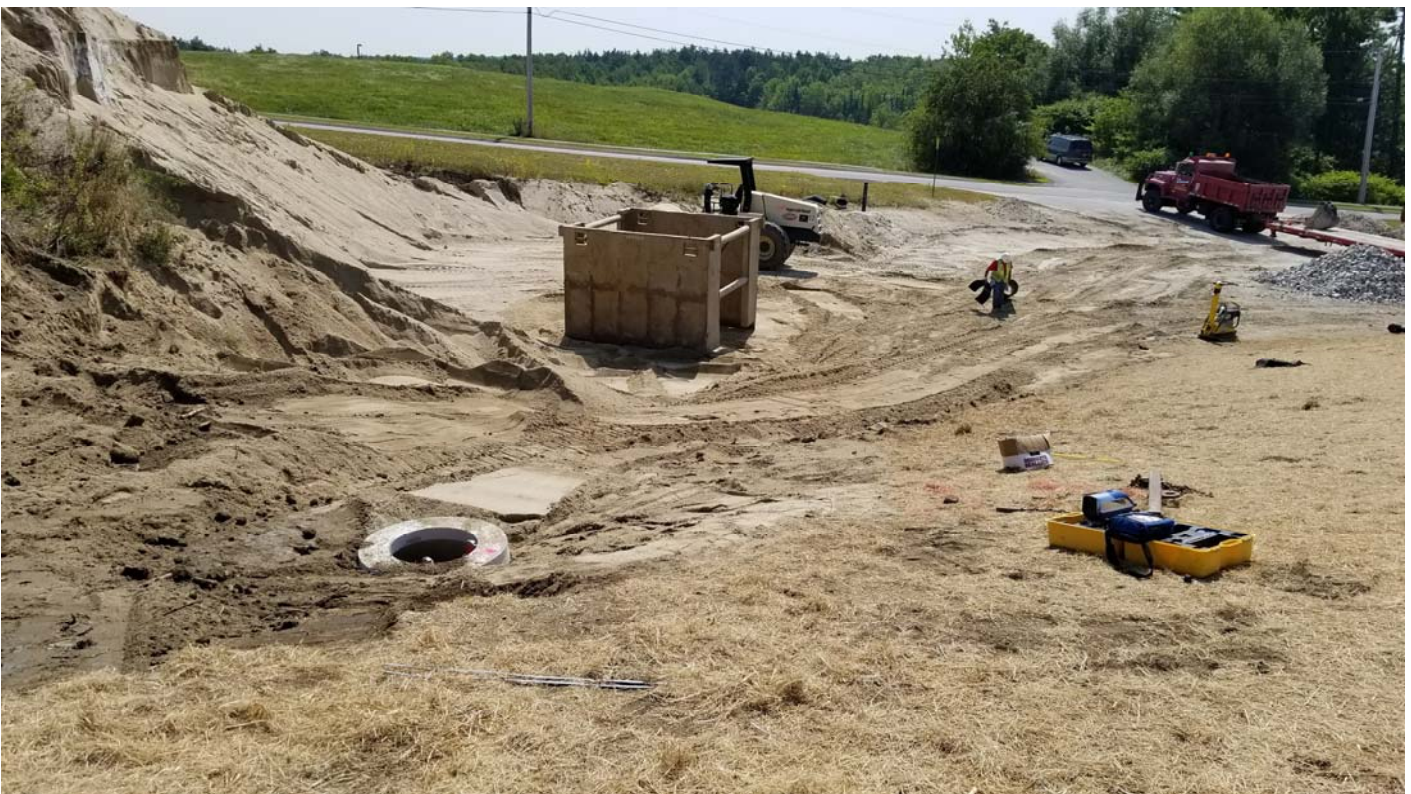
Stormdrain installed and backfilled along eastern edge of landfill.
