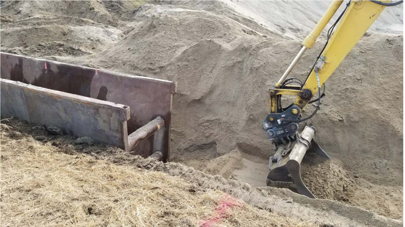
Backfilling behind the trench box.
